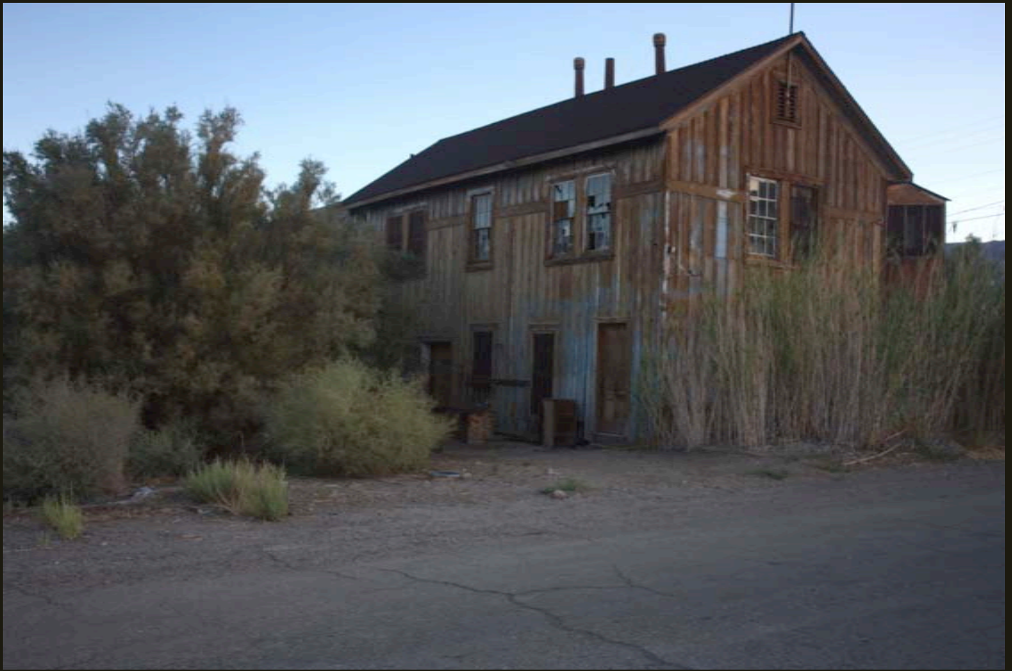
Northward view of the C&C/N&C/SP Keeler station. A siding ran just on this side of the building in the overgrown area and the mainline ran about where the pavement is cracked in the foreground.
