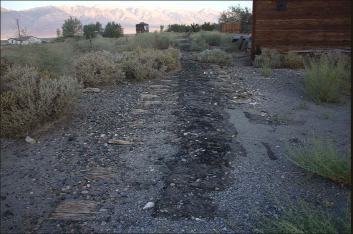
Northwestward view of ties at Keeler, 1,500 feet northwest of the mill. The ties are partly paved over and extend 200 feet from the C&C alignment and run northwestward on the west side of the mainline. I am guessing this track was the Inyo Development Company line, for two reasons: first, it is on the Owens Lake side of the C&C alignment, where the evaporate minerals were produced, and second, the ties may have been preserved because the IDC tracks were abandoned in the 1950's and may have been paved over prior to the salvaging of the SP (former C&C) trackage in 1961.
