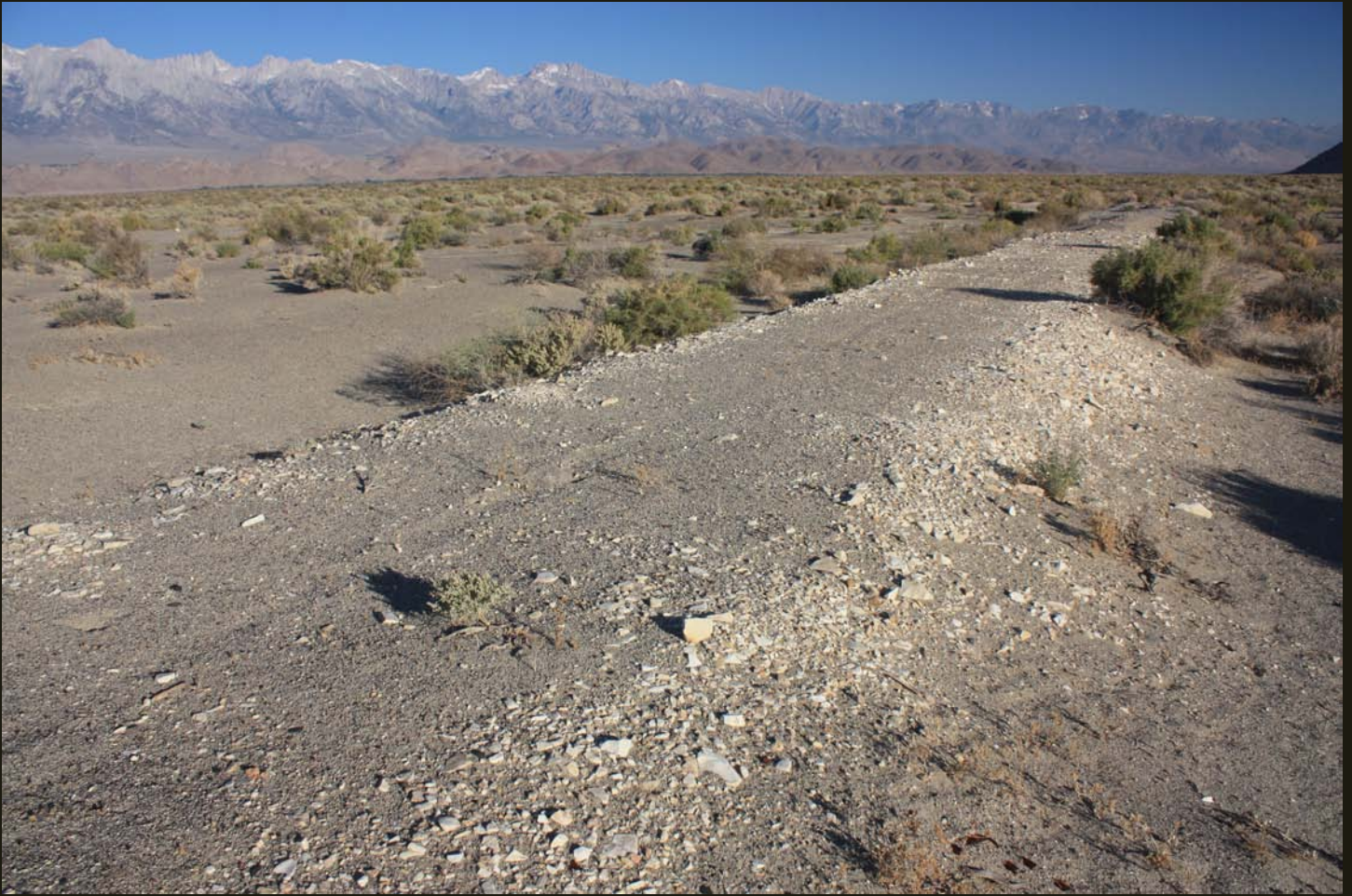
Northwestward view of the C&C/N&C/SP narrow gauge grade, same location as previous. The snowcapped Sierra Nevada, the westernmost normal fault of the Basin and Range geologic province, towers in the distance, and the Inyo Mountains foothills are just visible to the right.
