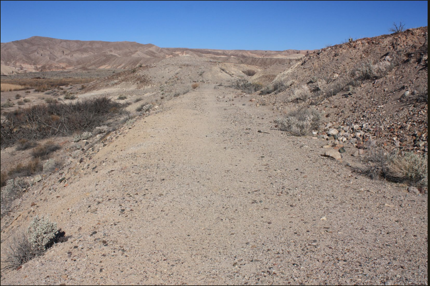
Northwestward view of the T&T (1907) 1,000 feet northwest of the previous location. The Amargosa River is still to the left of the grade. In the distance, the alignment turns to the right through a cut grade in a low hill; the alignment turns north-northeastward after the curve to follow the river.
