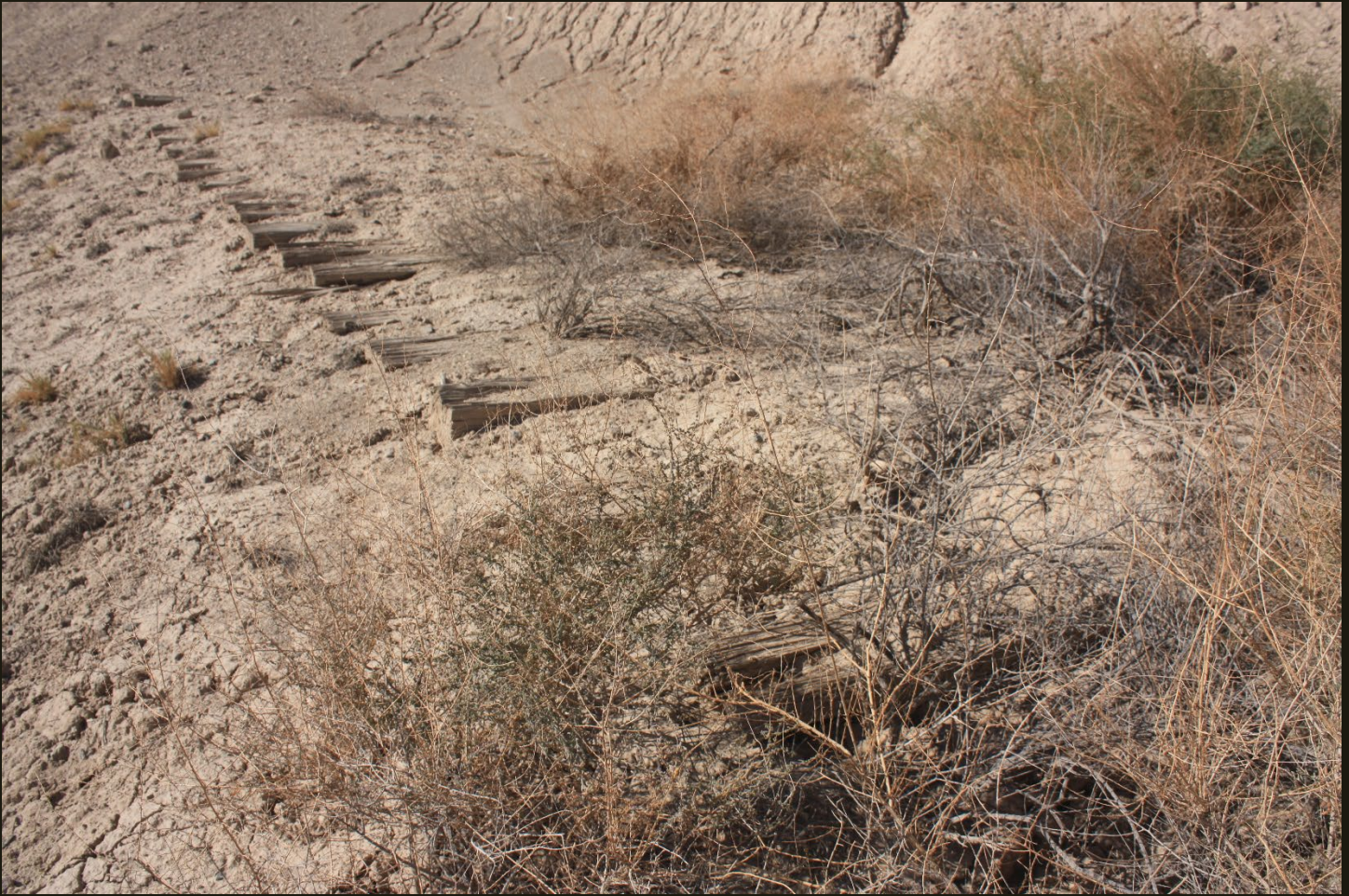
Ramp for runaway ore carts, near previous location. These ties appear to be original.
