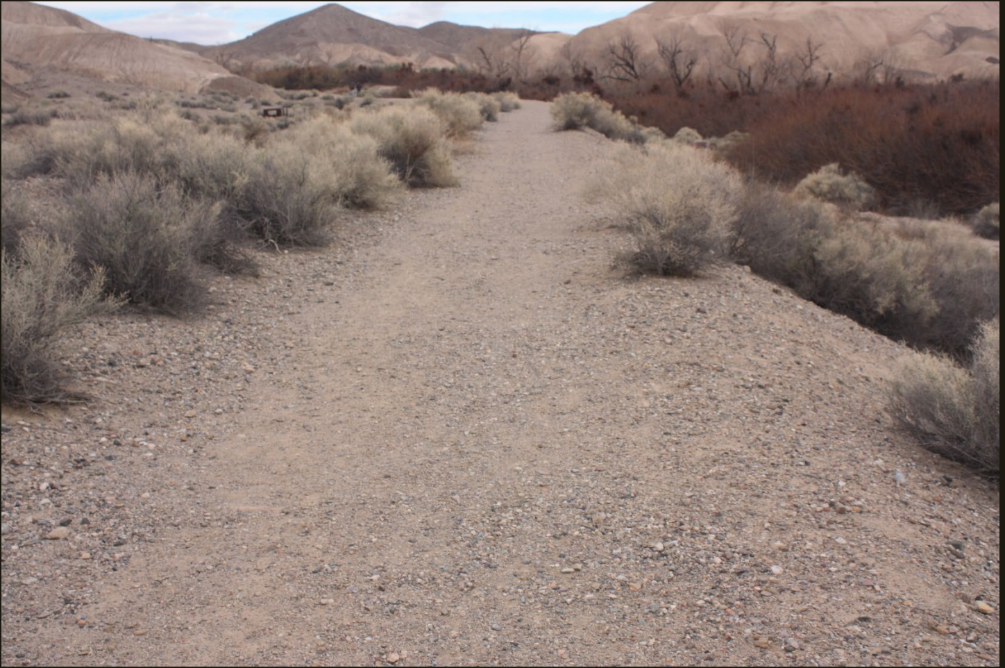
Northeastward view of the grade for Morrison Siding, 2,500 feet northeast of the previous location. Note the curve to the left (north) in the distance and the relatively lush growth, including trees, to the right of the grade along China Ranch Wash; that growth is the beginning of the riparian area associated with the spring at China Ranch.
