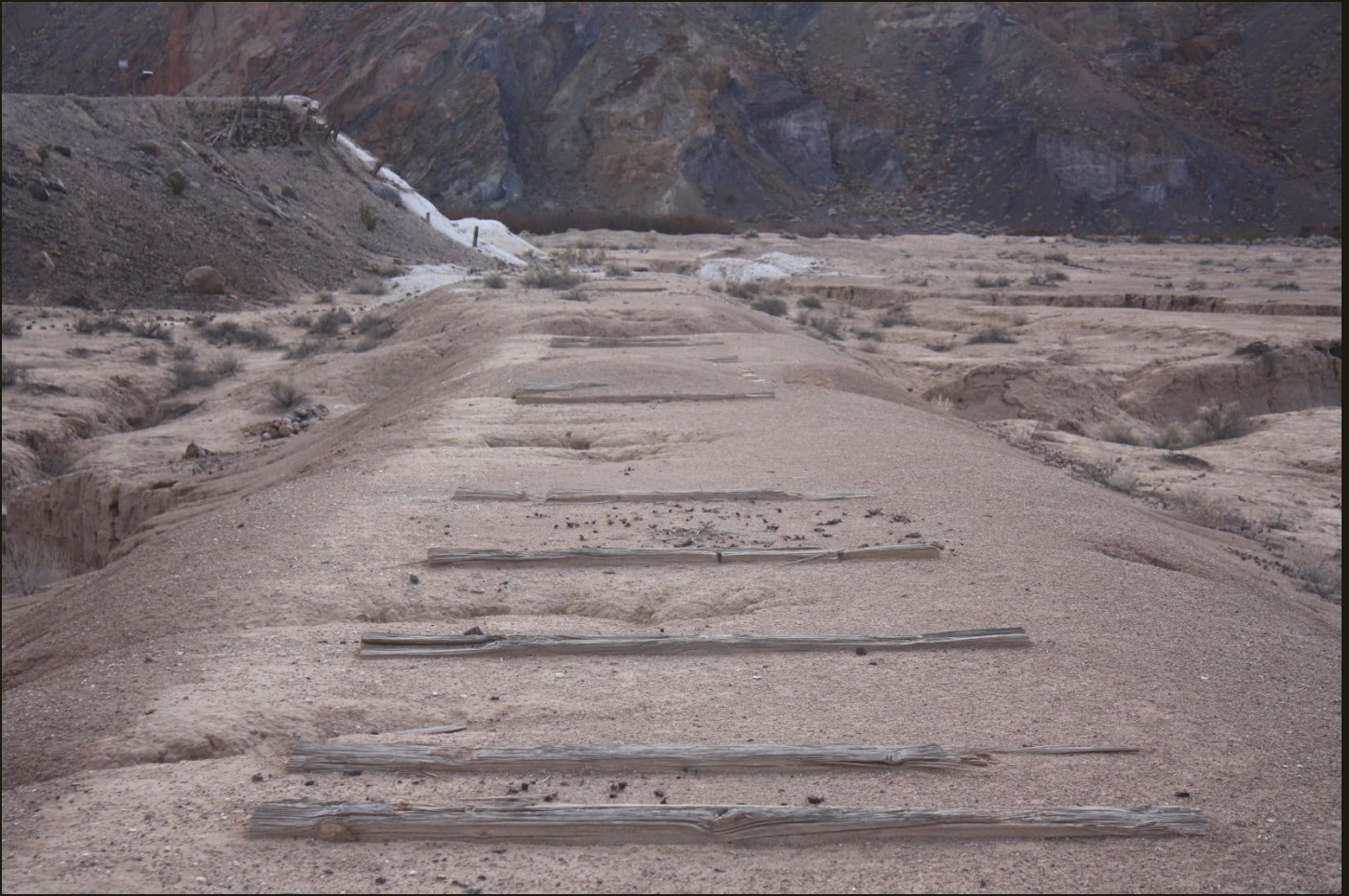
Now we've moved 3,000 feet south to the location of the first photo, looking southeastward at the T&T (1907) fill grade. Note the white dirt and woodwork on the bluff; this was a loading facility for the Morrison Siding, discussed below.
