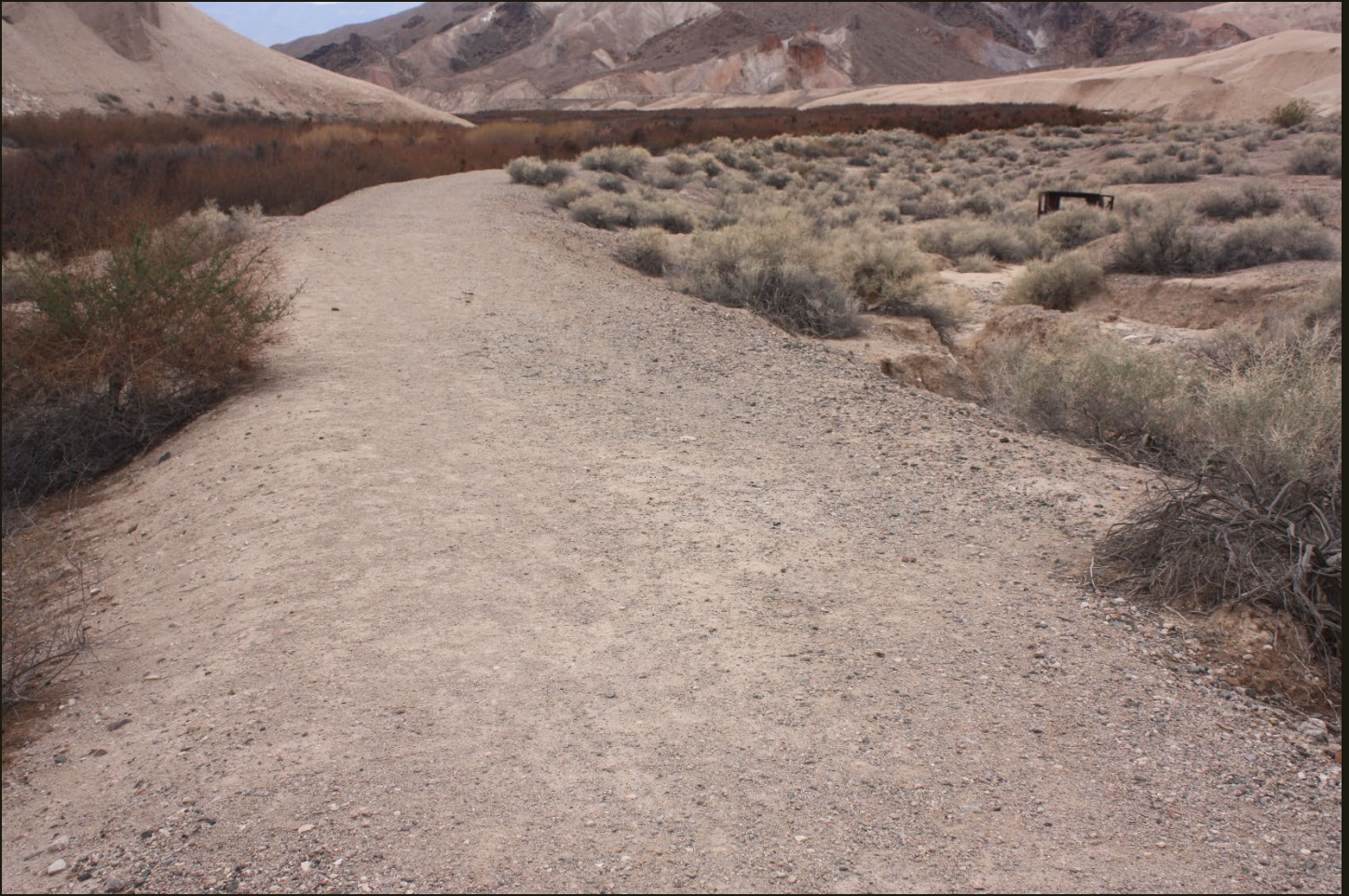
Southwestward view of the grade for Morrison Siding, 1,000 feet northeast of the previous location. The curve is the same curve seen in the distance of the previous photo and the relatively lush growth along China Ranch Wash is to the left of the grade. The Amargosa River and the T&T (1907) are at the far end of the riparian growth and just in front of the darker, higher hill in the middle distance.
