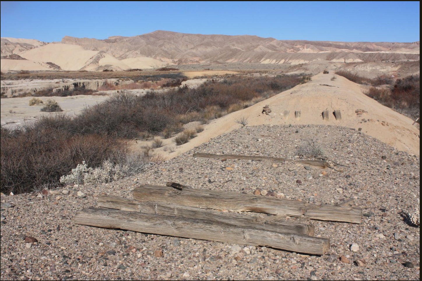
Northwestward view of the T&T (1907) 2,000 feet northwest of the previous location. The ravine with orange foliage to the left of the grade is the Amargosa River. The color of the T&T fill grade changes at a breach in the fill to allow a side wash to flow through to the Amargosa River. Note the wooden posts at the other end of the breach; the posts once supported a small bridge.
