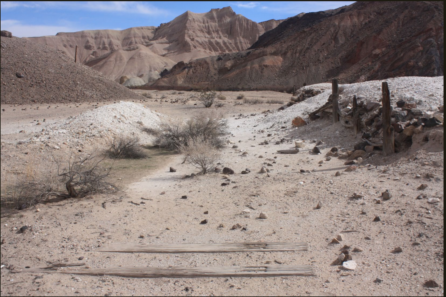
Morrison Siding was built in 1915; it was a one-mile ore-car track built to carry gypsum and talc ore from mines located up China Ranch Wash to the T&T for shipment. In this westward view at the top of the white-dirt-covered bluff we can see a shallow cut grade, ties, and a retaining wall for Morrison Siding. The trackage ended before the drop-off of the bluff, just beyond the retaining wall on the right. The white dirt is gypsum and talc ore that spilled incidentally during unloading of ore carts at this location and loading onto T&T ore cars down off the bluff just to the right of the photo.
