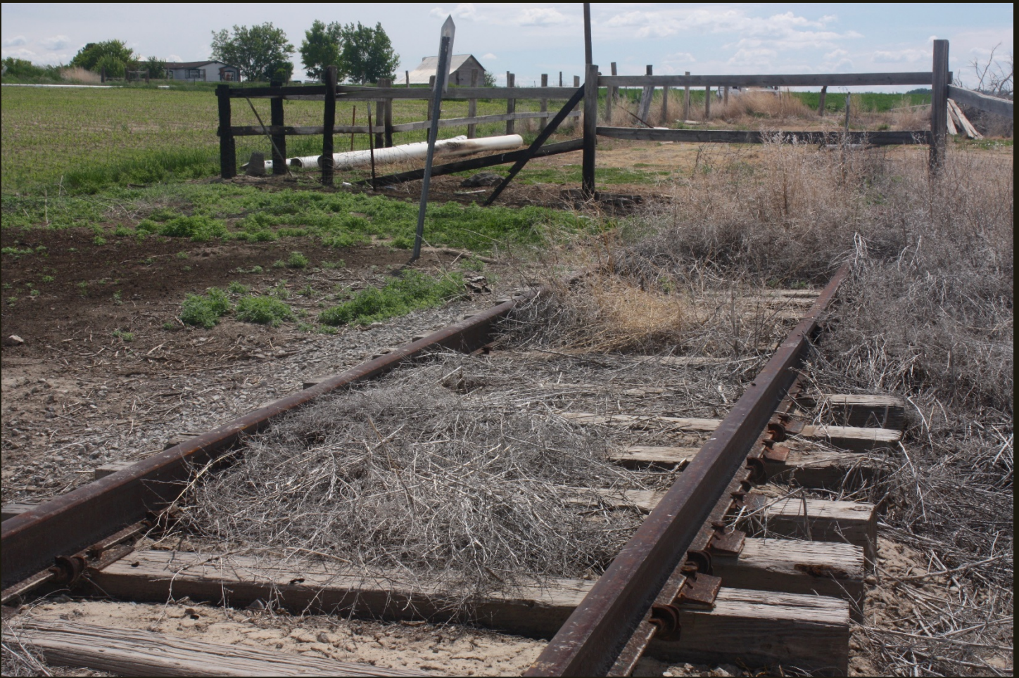
Southward view of IC Rogerson Branch (1910)/OSL Wells Branch (after 1926) end-of-track. The abandoned grade is obliterated here and points south to around Rogerson, where the alignment crosses irrigated agricultural land, but is preserved in non-irrigated land south of Rogerson in Idaho and Nevada.
