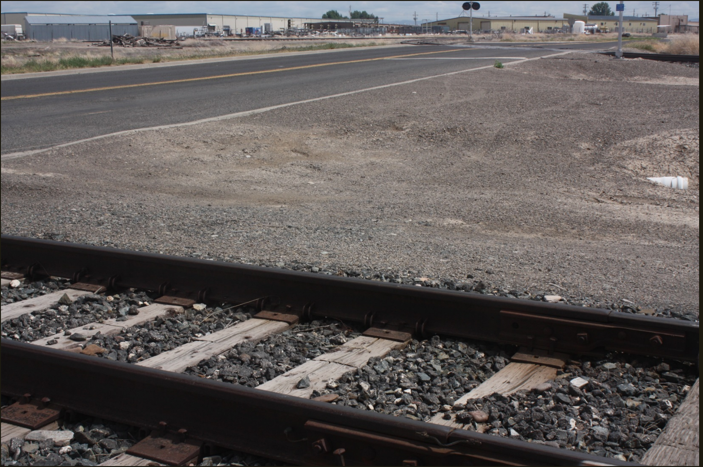
Southeastward view of the M&SW (1905) mainline (foreground) and the wye for the IC Rogerson Branch (1910), same location as previous. The track in the right middle distance (and crossing the road) is the west branch of the wye and the track in the left distance is the east branch.
