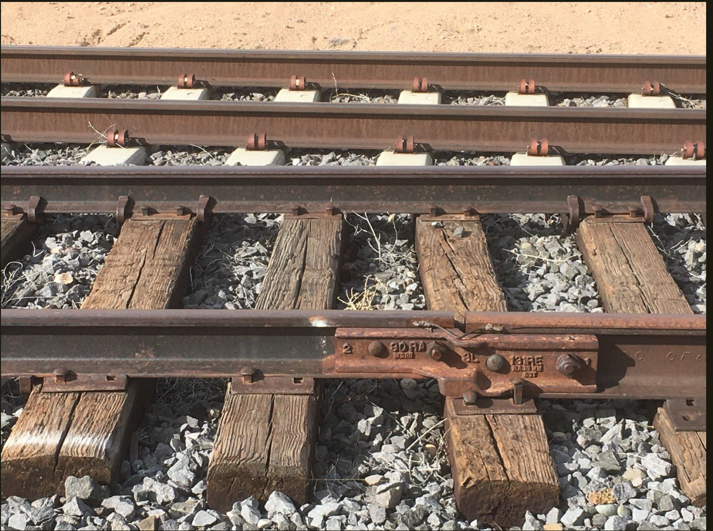
Westward view at the same location as previous. The non-upgraded NM&SP Santa Fe Branch (1880) is in the foreground and the New Mexico Rail Runner Express (2008) is behind it.
