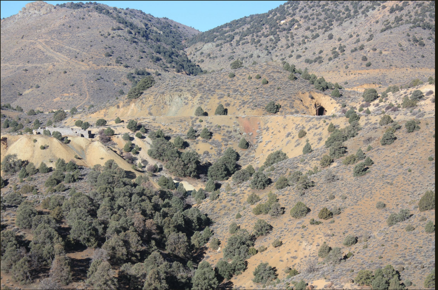
Tunnel on the V&T (1872), one mile south of Virginia City. The foundation of another old mining-related structure is visible at the far left.
