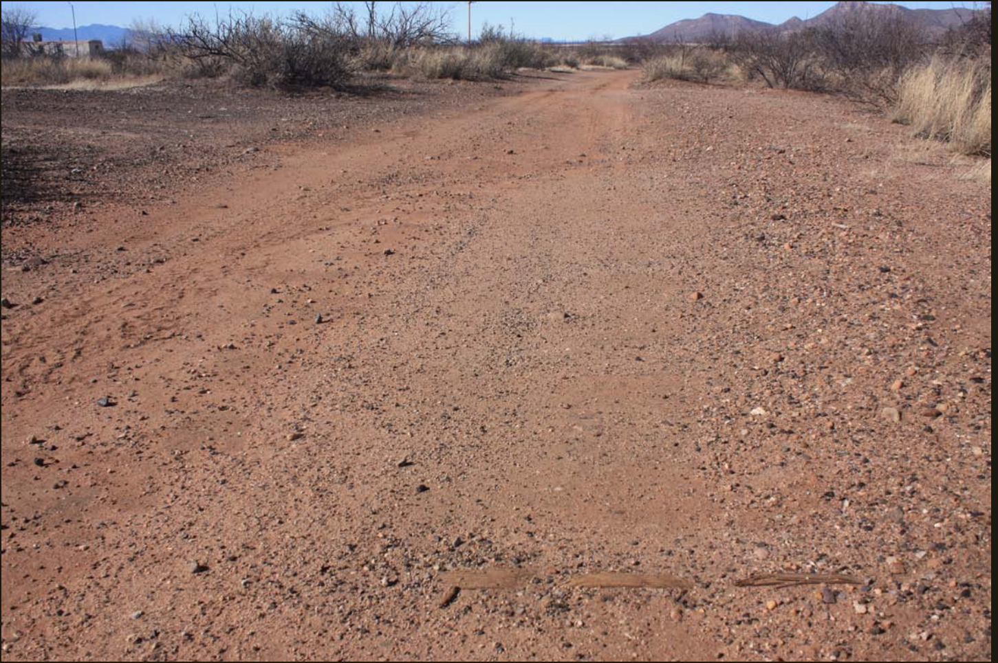
Northwestward view of the N-C (1902), 100 feet south of the previous location; the darker ballast of the EP&SW (1904) is still barely visible in the distance. Note the tie still in the road bed in the foreground; it is wood, not an impression.
