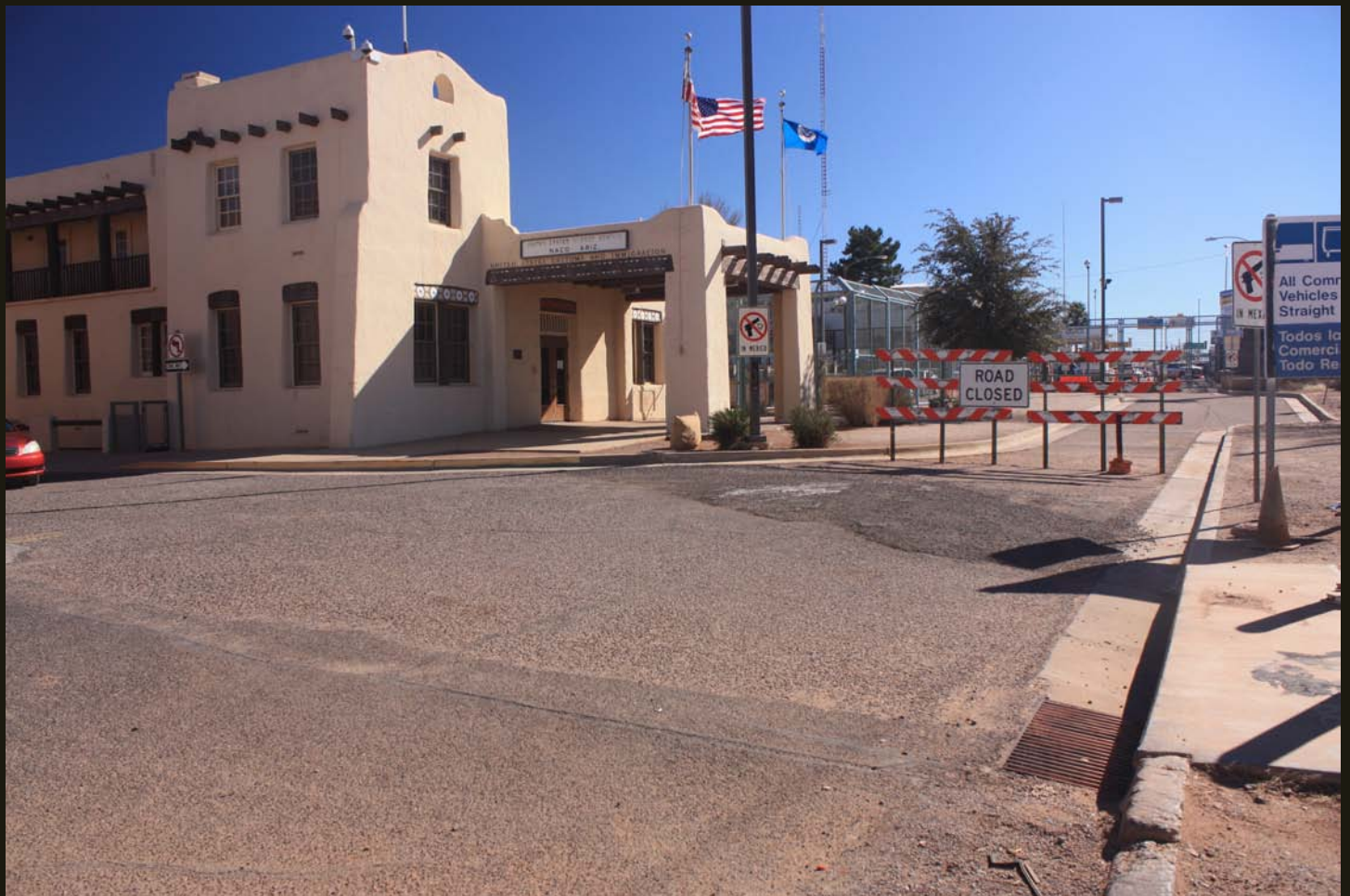
Southward view of the old Naco Port of Entry; the N-C (1902) entered Mexico at the location of the gate in the right distance. The historic Adobe-style border station was built in 1937 and now serves as Customs and Border Control office space. A new border inspection station was built in adjacent space in 1994.
