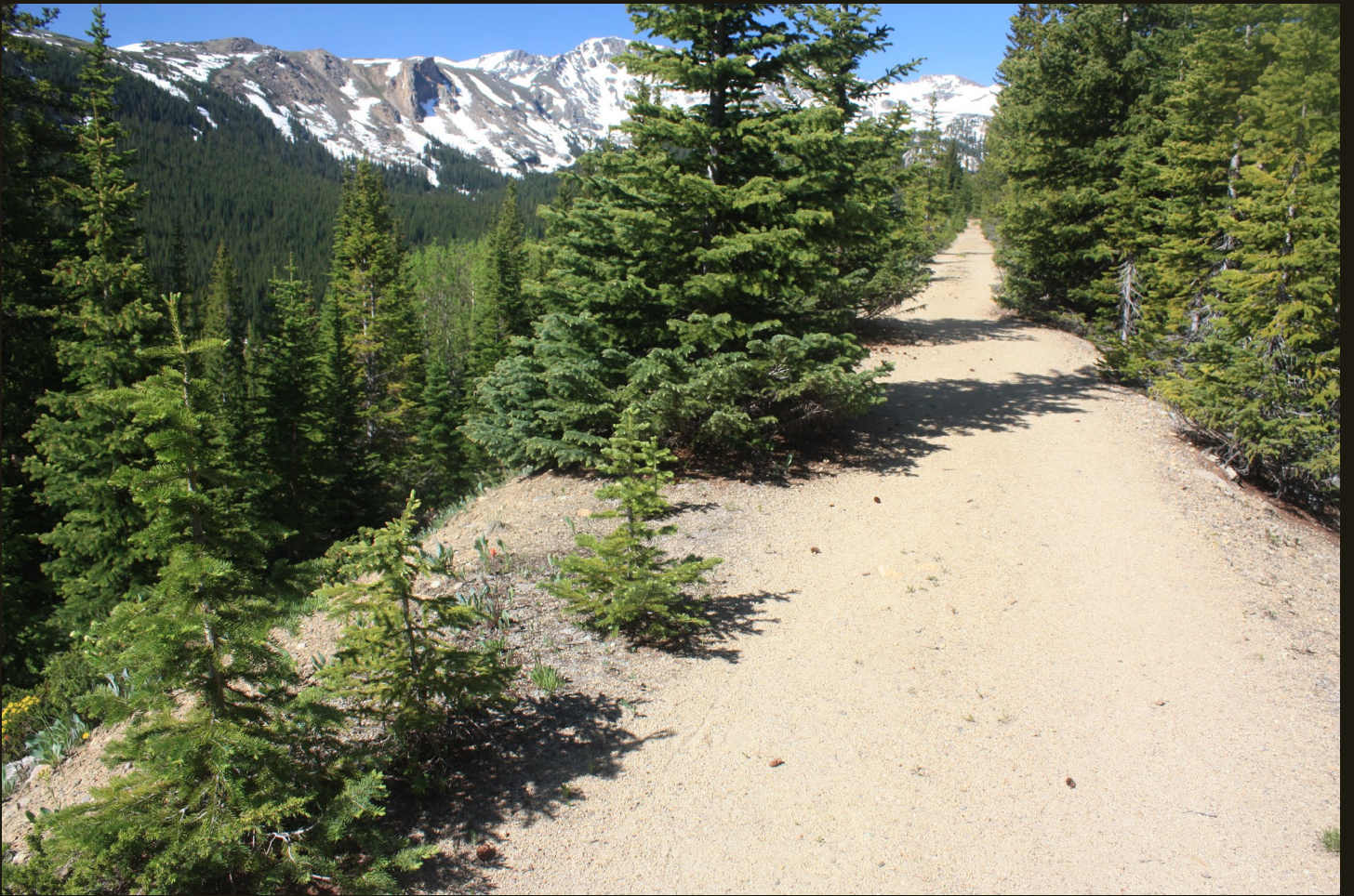
Westward view of a straight section of the grade on the CM ascent to the Hagerman Tunnel.
