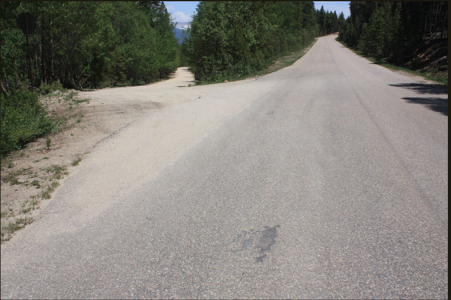
The road to the left in this eastward view is the CM grade down to Turquoise Lake. The main road is Forest Road 105, which follows the CM grade west from this point toward Hagerman Pass.
