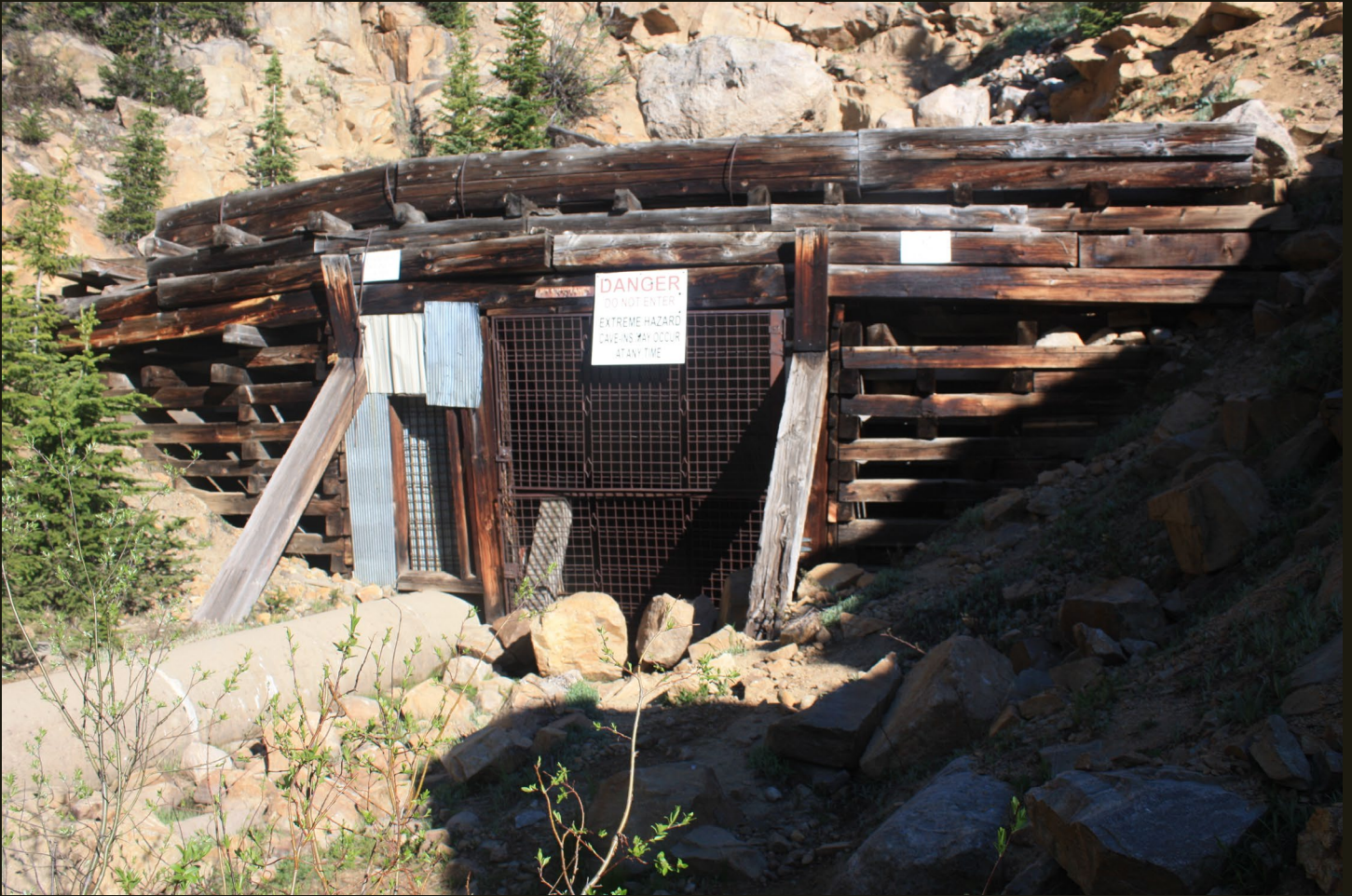
The CM built two summit tunnels for its crossing of the Continental Divide at Hagerman Pass. The first tunnel was the Hagerman Tunnel, completed in 1887 during the original construction of the road. In 1891, it was replaced by the lower and longer Busk-Ivanhoe Tunnel, whose east portal is shown here.
