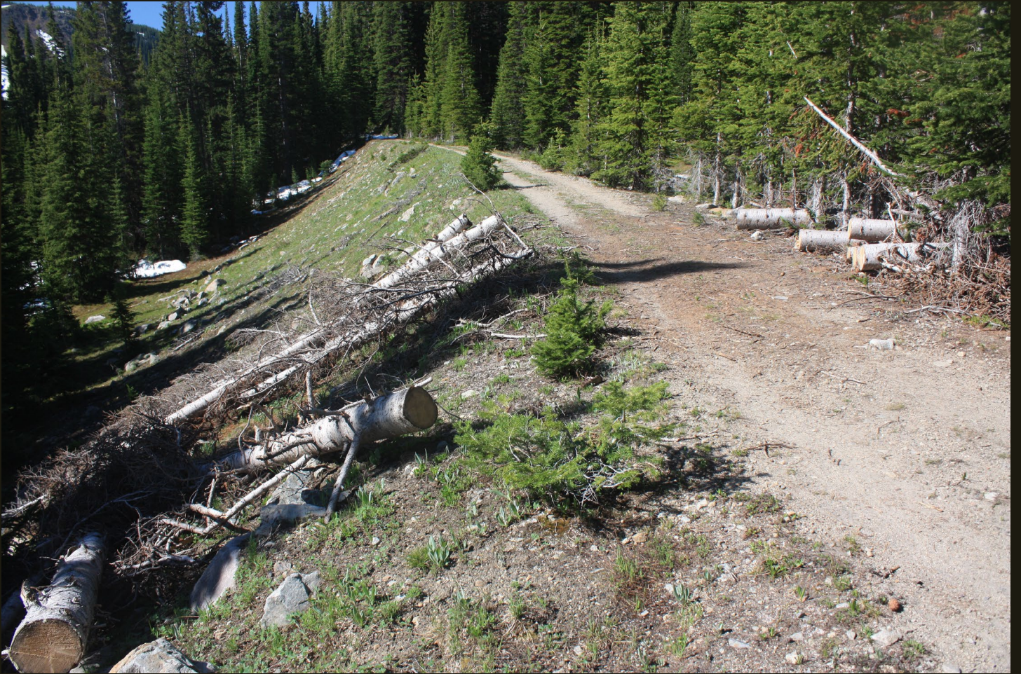
A fill grade on the CM ascent to the Hagerman Tunnel.
