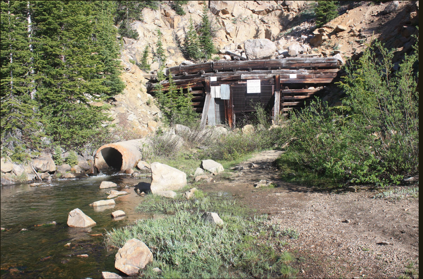
Groundwater flows out of the Busk-Ivanhoe Tunnel.
