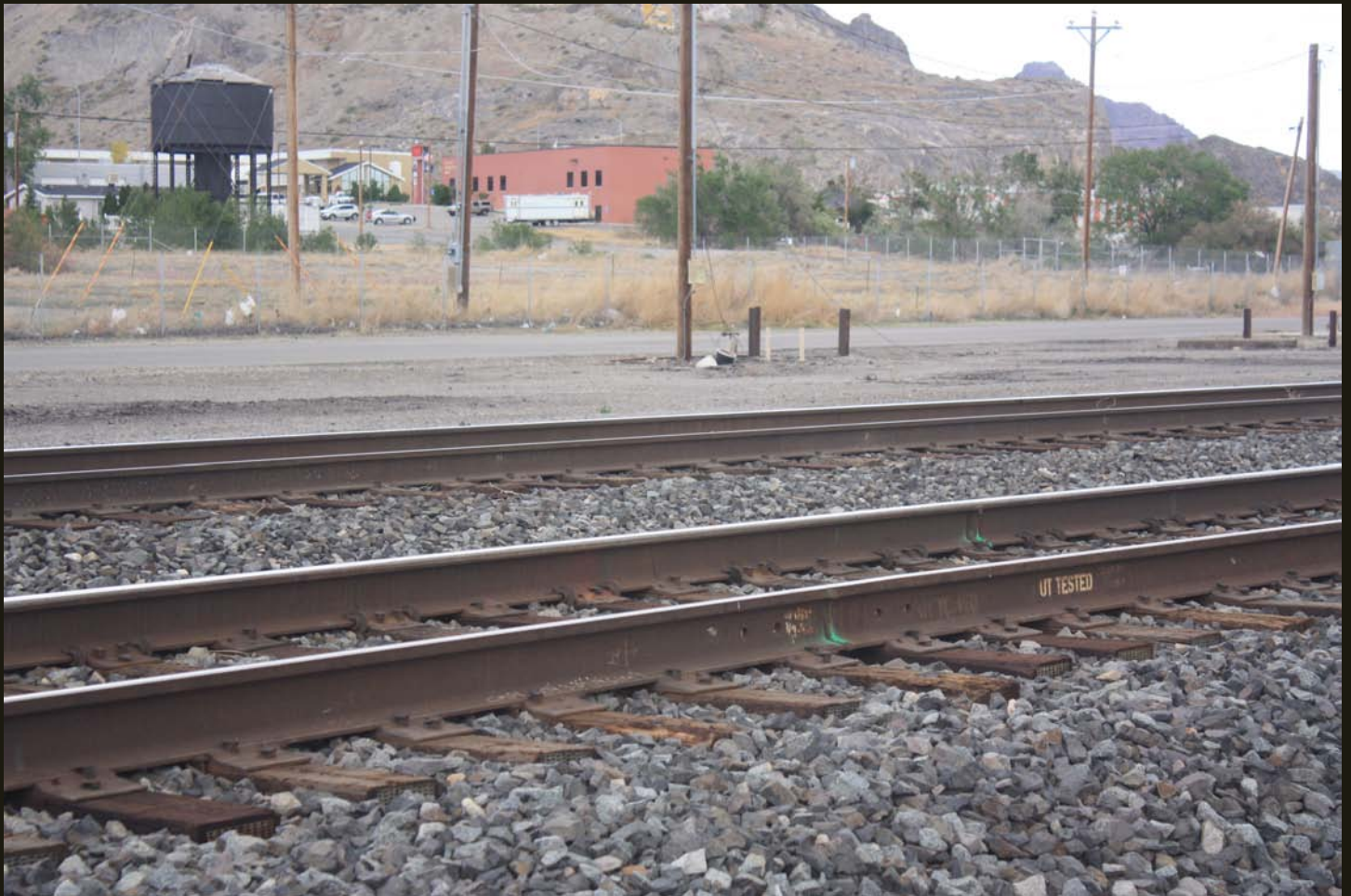
Northward view of the WP (1909) at the same location as previous. The location of the former roundhouse is just out of the image to the left and its foundations are still evident in satellite photos, but I didn't know to look there when I visited. I did manage to find the water tank.
