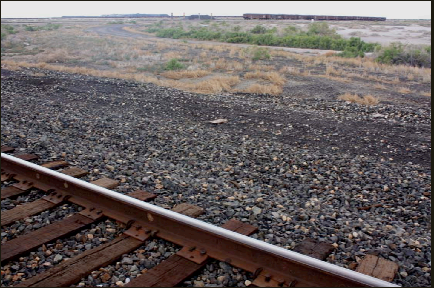
Southeastward view of the WP (1909), 300 feet west of the previous location. The same cars are on the spur to the evaporite mineral facility, the southernmost WP track is in the foreground, and the abandoned west branch of a wye is evident between the two.
