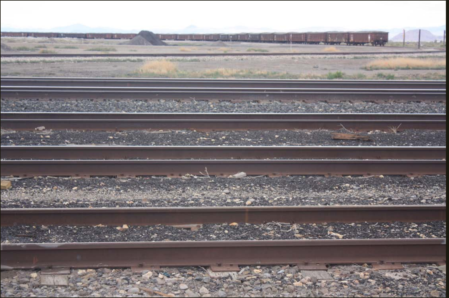
Southward view of the WP (1909) yard (now Union Pacific) east of Wendover. The cars are on the spur to the evaporite mineral facility. The curved section of the spur, beyond the 5 straight tracks in the foreground, was once the east branch of a full wye (the west branch has been abandoned). The closer cars on the right are on track that heads south and the more distance cars are on track that curves to due east in the far left distance.
