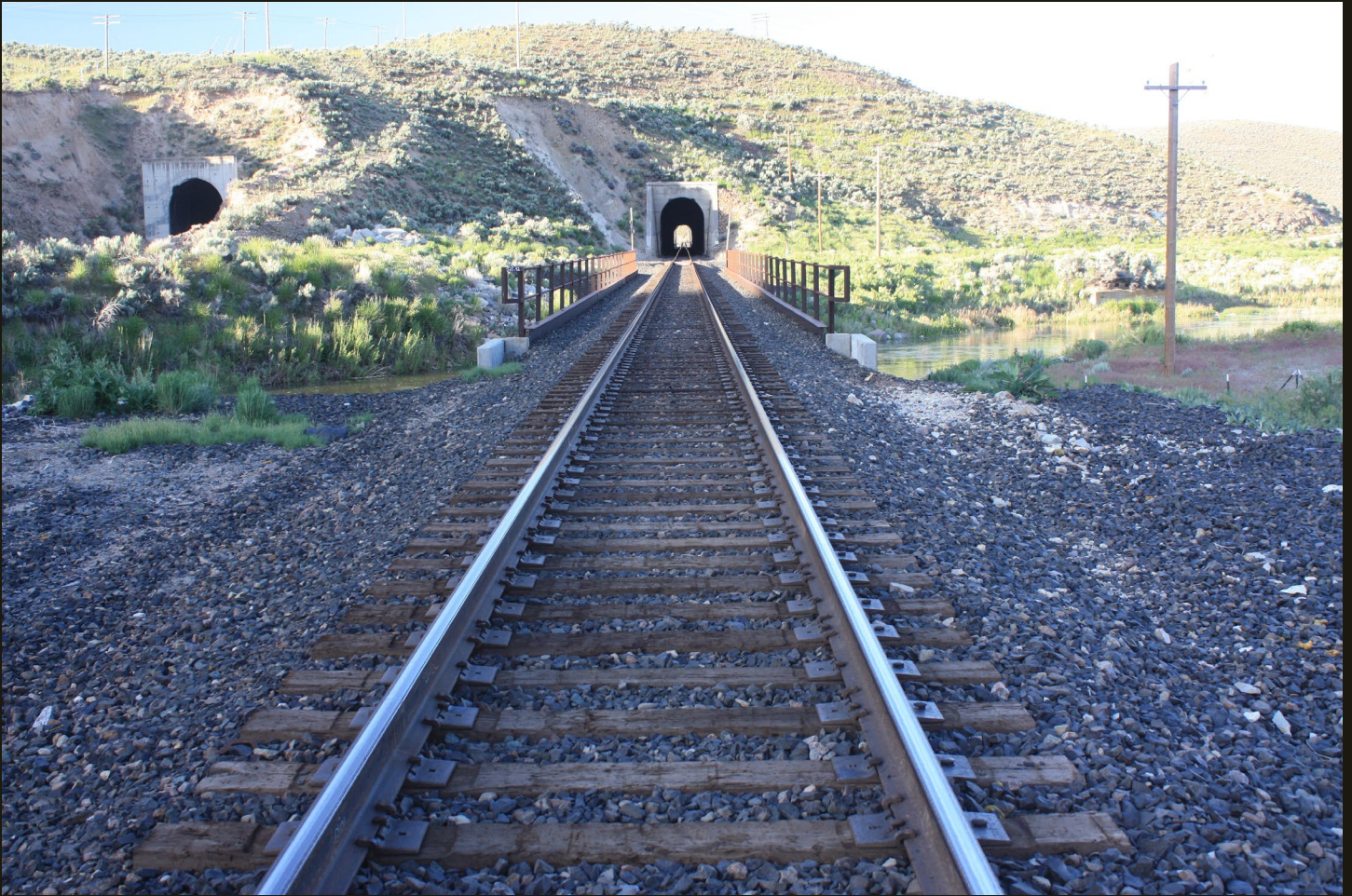
South-southwestward view 700 feet east-northeast of the previous location, at the same location as the locomotives in the previous photo. We are looking straight through the SP tunnel and all the trackage in this view is on the 1901-1903 realignment. The WP (1909) tunnel is to the left. The bridge in the foreground crosses to the northwest side of the Humboldt River, but the WP (1909) stays on the southeast bank.
