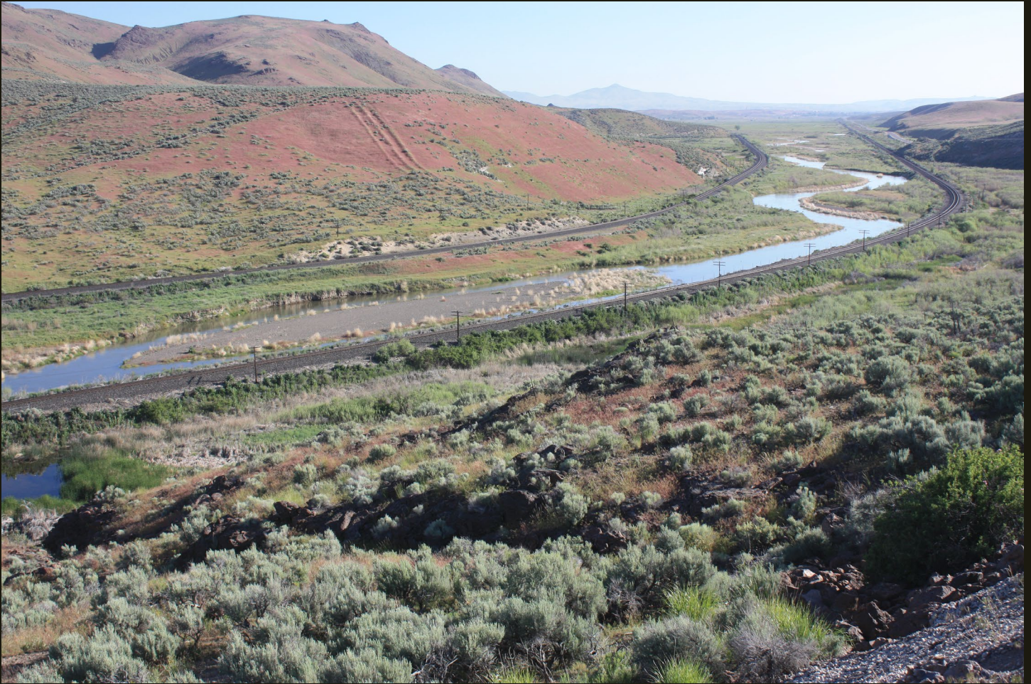
Northeastward view 2 miles northeast of the previous location. The CP (1869) is on the far bank of the Humboldt River and the WP (1909) is on the near bank. The CP (1869) is on its original alignment in the left part of the picture, but the straight segment just beyond the first curve to the left originally curved farther left to follow the base of the slope; the SP straightened this segment during its 1901-1903 realignment program. Both railroads are now UP.
