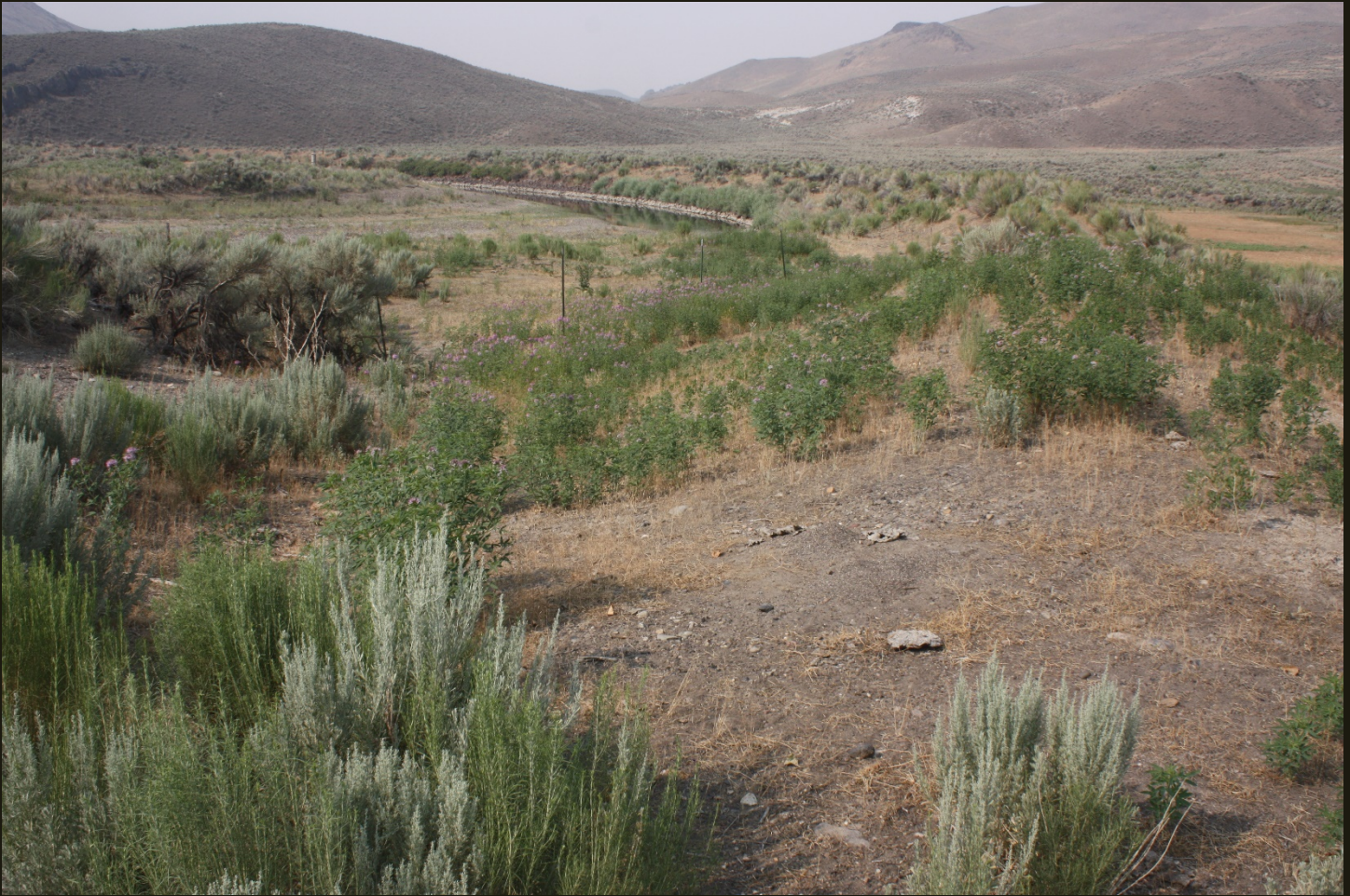
Southwestward view 1,400 feet northwest of the previous location. The viewer is on the original CP (1869), which bends to the left with the Humboldt River; note the rock embankment on the left (east) side of the fill grade to prevent erosion of the embankment. Although there is no evidence today on the ground or in satellite imagery, the E&P (1875n) grade was across the river in the left part of the photo and ran toward the viewer on a bridge across the river and crossed the CP (1869) track just about where the viewer is standing.
