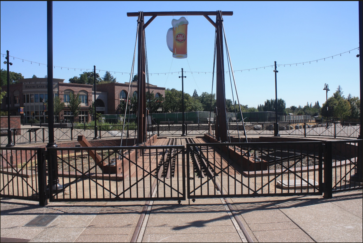
Southwestward view of the Folsom turntable, a few steps southwest of previous location. There was no turning wye at the Folsom end of track, which necessitated a turntable. The depot and end of track are behind the viewer. The track in the foreground leads back to the switch to the mainline in the previous photo (behind the viewer). A clockwise turn of the turntable of about 30 degrees aligns the turntable track with the continuation of the siding for the turntable on the other side.
