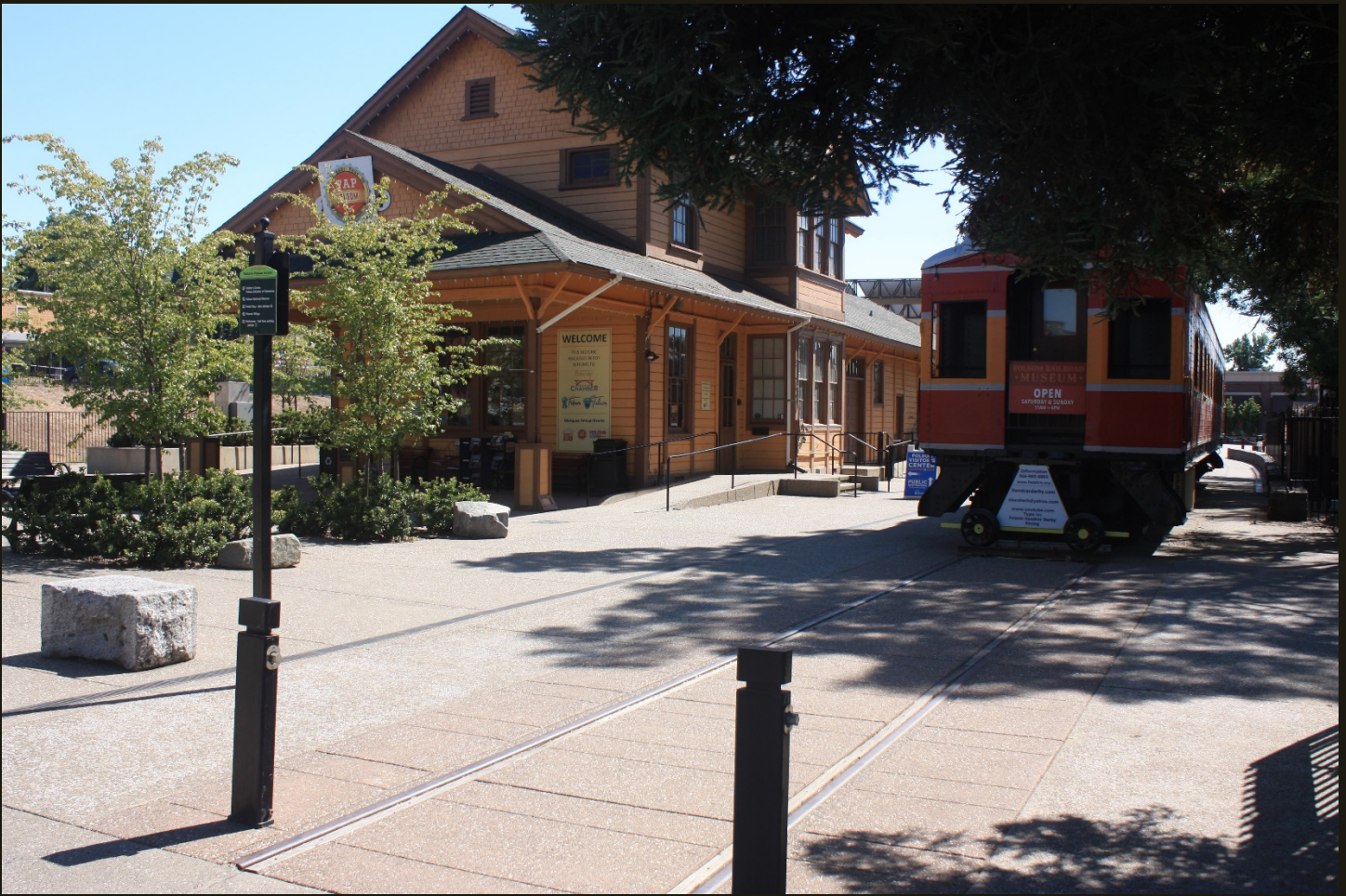
Southward view of the SV (1856) end of track (left foreground), same location as previous. The train depot on the left was first built in 1909 and enlarged in 1916. A vintage passenger car adorns the tracks.
