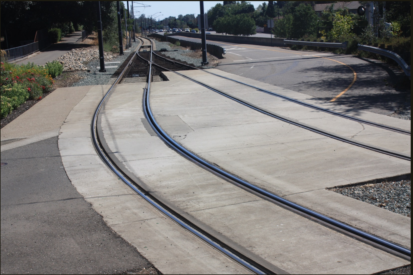
Southward view just steps south of the previous location. The straight track in the middle distance projects northward (toward the viewer) to the SV (1856) alignment in the previous photo and thus is on the SV (1856) alignment. The tracks are the Sacramento Regional Transit District's Gold Line commuter train. The curve in the foreground leaves the historic alignment and leads to a 400-foot track on a new alignment for Gold Line passenger loading.
