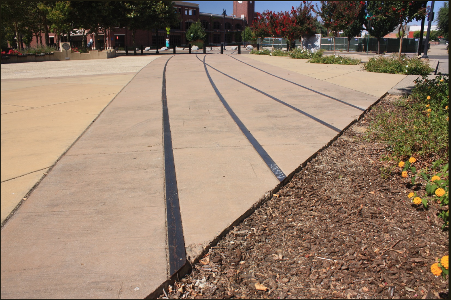
Northeastward view 300 feet southwest of previous location; the brick building in the distance is the same one that truncates the two sidings in the previous photo. Two tracks converge toward the viewer but are cut off before the switch to make way for a planter and the Gold Line. The track on the left is the mainline and the track to the right is the siding for the turntable. This is the south end of the renovated historic district and the end of track of the first railroad in the Southwestern U.S., as modified by the CP and SP over more than 150 years and as represented today by these tracks.
