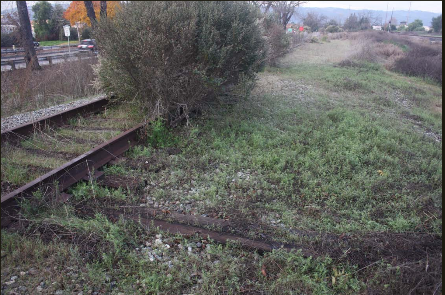
Westward view of track on the WP (1869) grade; note the long tie in the foreground, indicative of a former switch, possibly associated with the wye for the SP San Ramon Branch (1909). WP (1909) main line in the right distance.
