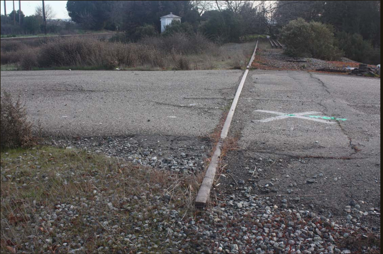
Eastward view of the west end of remnant track on the WP (1869) grade. WP (1909) main line in the left distance. Same octagonal structure is the same one as in the previous photo.
