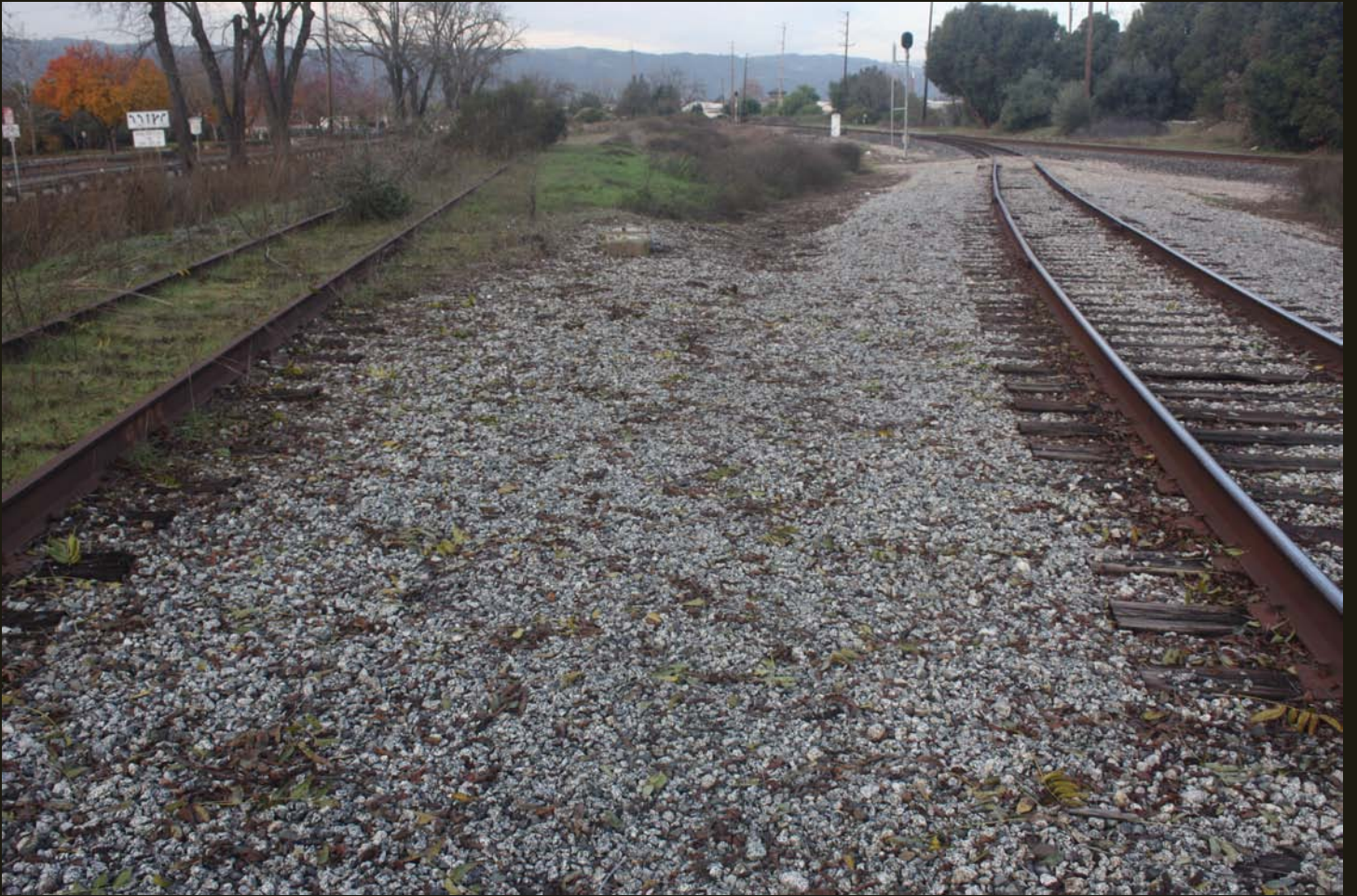
Westward view at the same location as previous. The curved track to the right is a siding of the WP (1909), which merges with the main line in the right distance. The straight rusty track on the left is on the WP (1869) grade.
