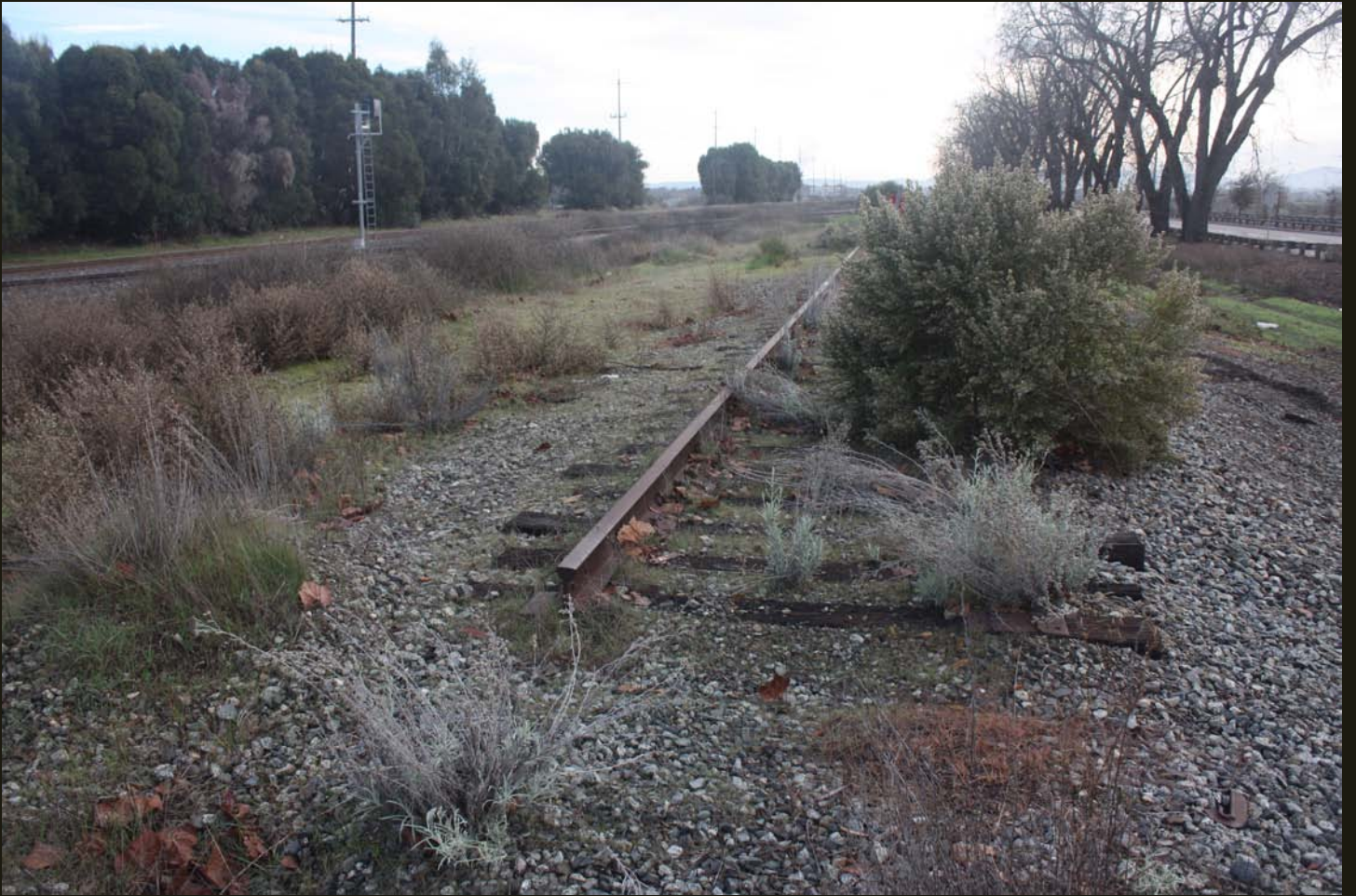
Eastward view of partially removed track on the WP (1869) grade. WP (1909) main line in the left distance.
