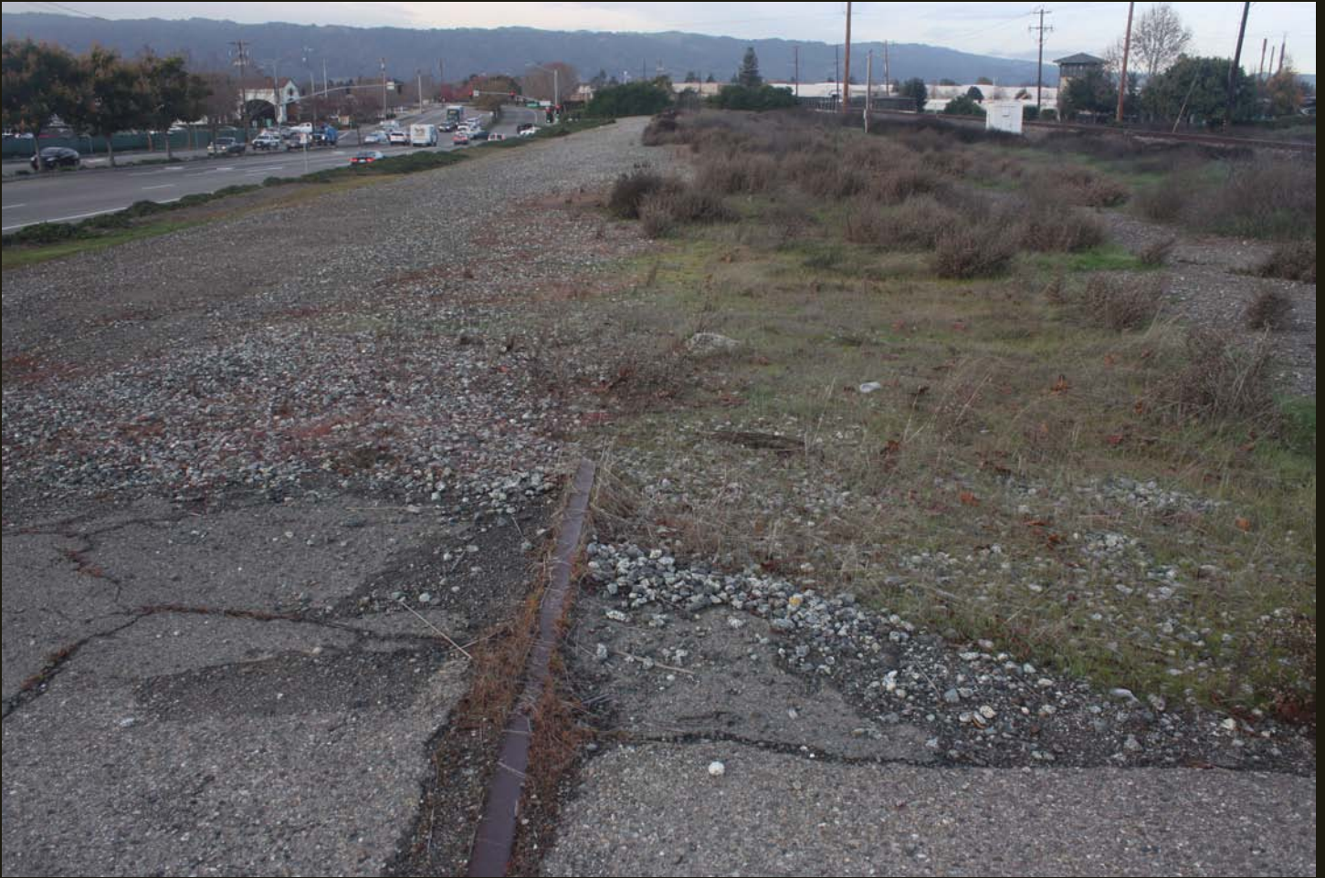
Westward view of the west end of remnant track on the WP (1869) grade, same location as previous photo. WP (1909) (now UP) main line in the right distance.
