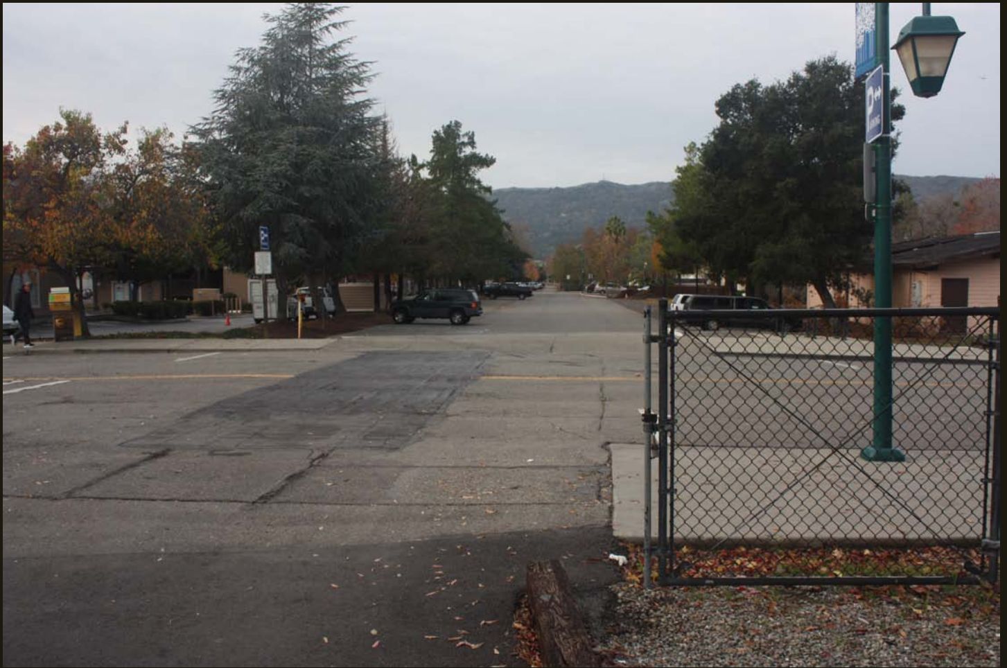
Southwestward view of the WP (1869) grade, now an alley, just south of the Pleasanton station. The asphalt patch in the street is likely where tracks were removed in 1979. The tracks pick up again on the WP (1869) grade about 2 miles southwest of this location.
