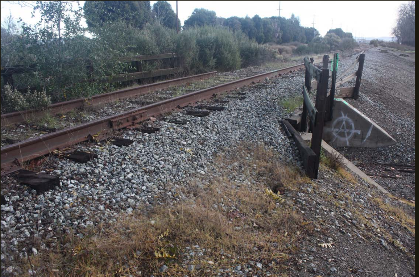
Eastward view of WP (1869) tracks and a culvert.
