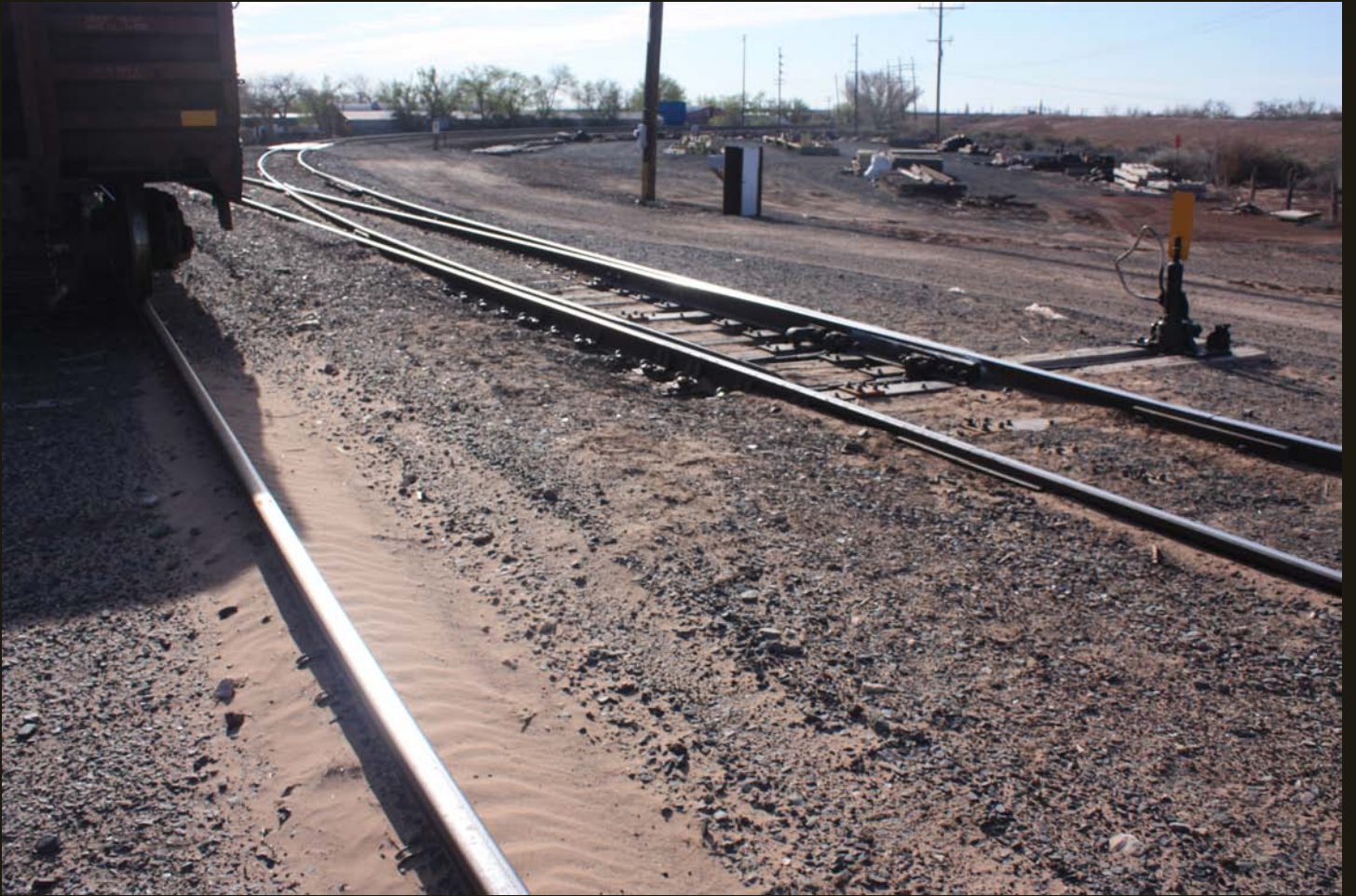
The switch for the Apache Railway connection to the AT&SF (now BNSF) mainline at Holbrook.
