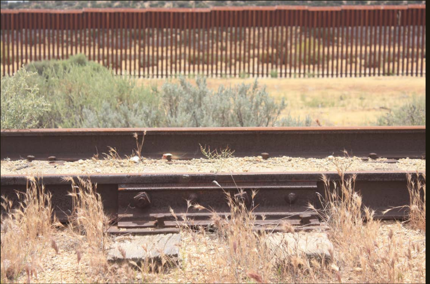
Bolted rail on the SD&A and the Border Fence.
