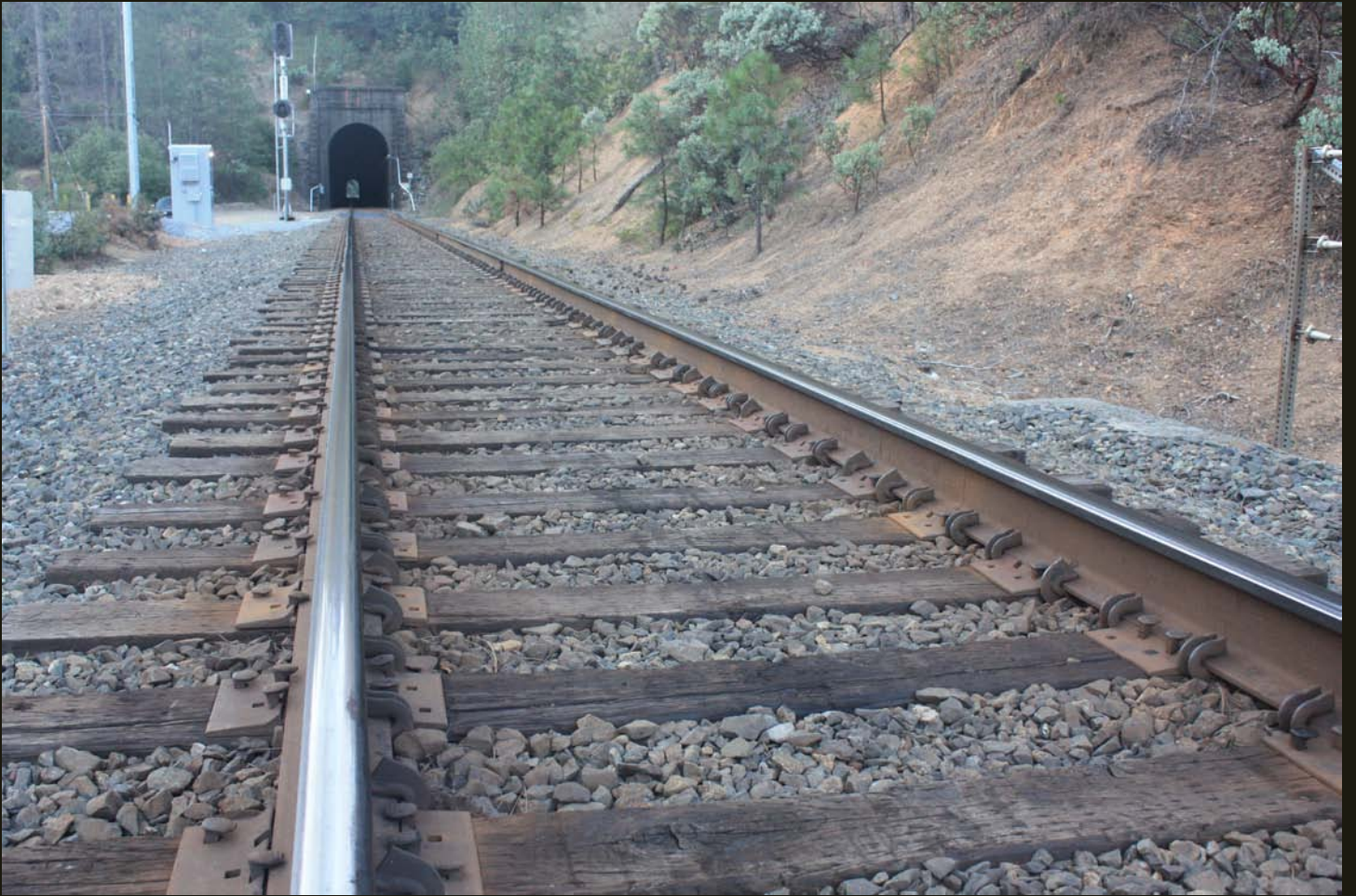
Same location as previous but turned around (looking south) to view one of several tunnels required for the C&O/SP Shasta Lake re-alignment.
