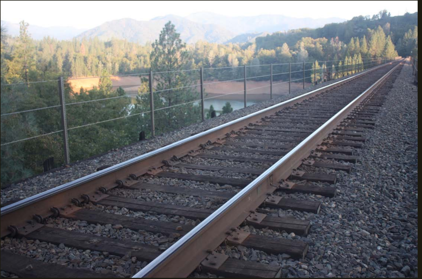
Northward view of the same bridge.
