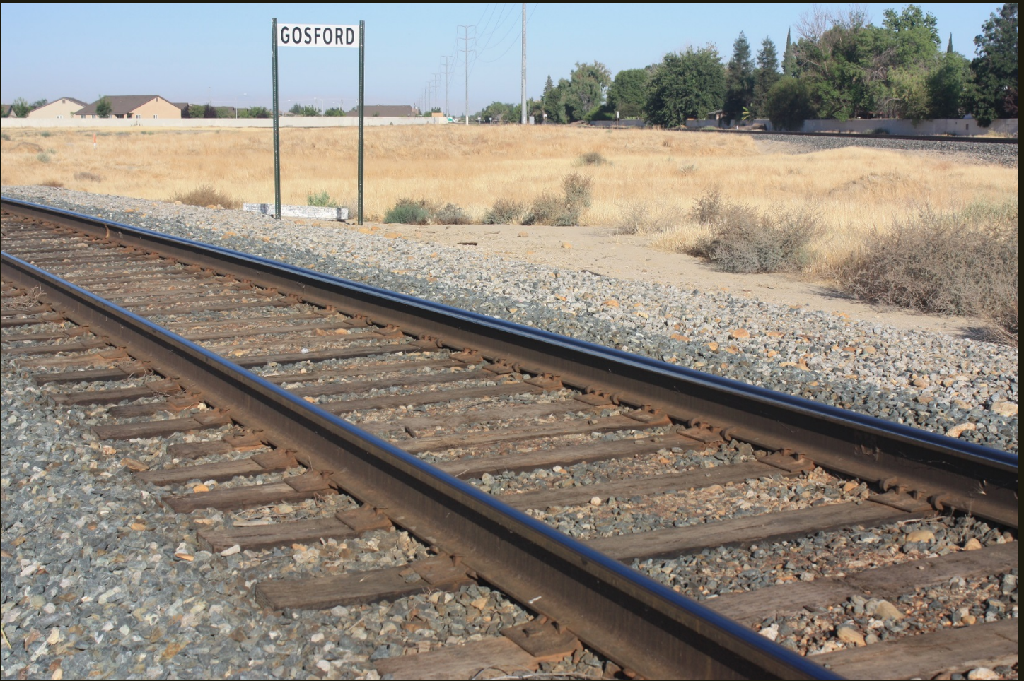
Westward view of the junction at Gosford, 200 feet south of the previous location. The curved track in the foreground is the east branch of the wye for the SW (1909). The curved fence line that encloses the residential area behind the "Gosford" sign is behind the west branch of the wye. The track in the right distance is the MS (1893).
