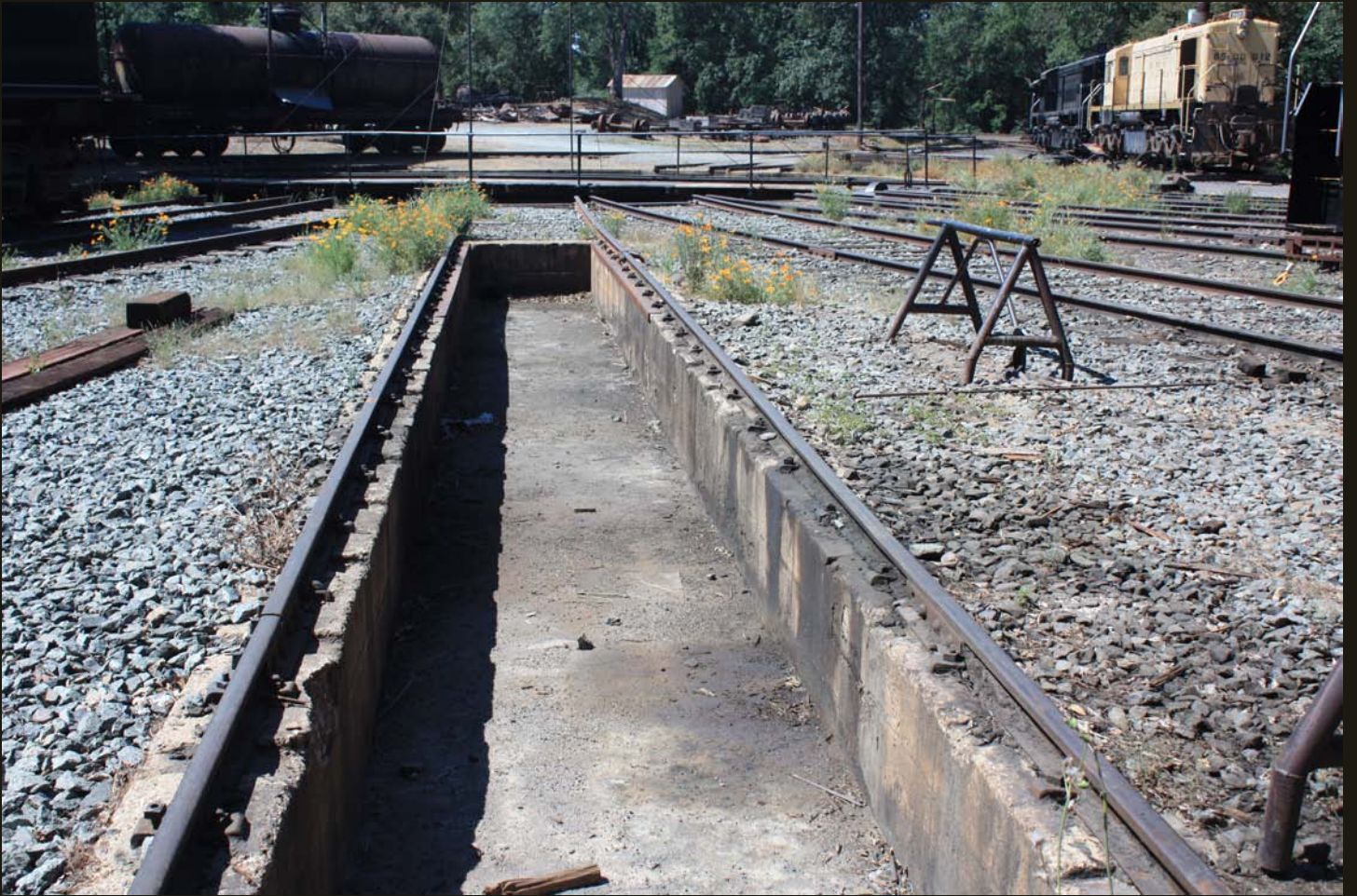
Jamestown maintenance facilities.
