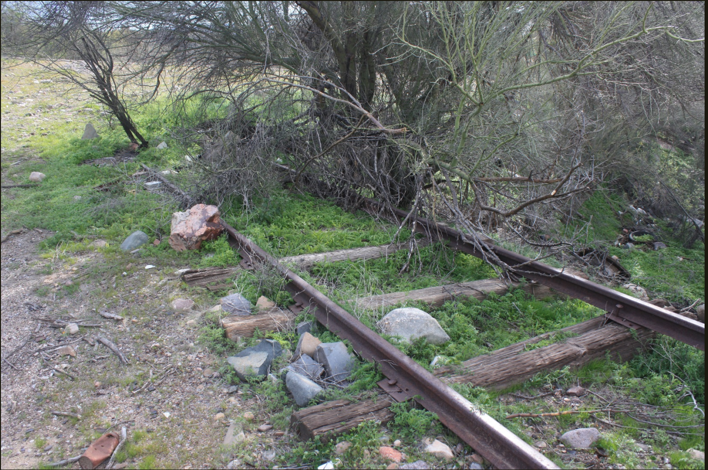
Eastward view of the end of track of the siding for the loading ramp, 250 feet east of the loading ramp. There is no evidence of the siding east of this point.
