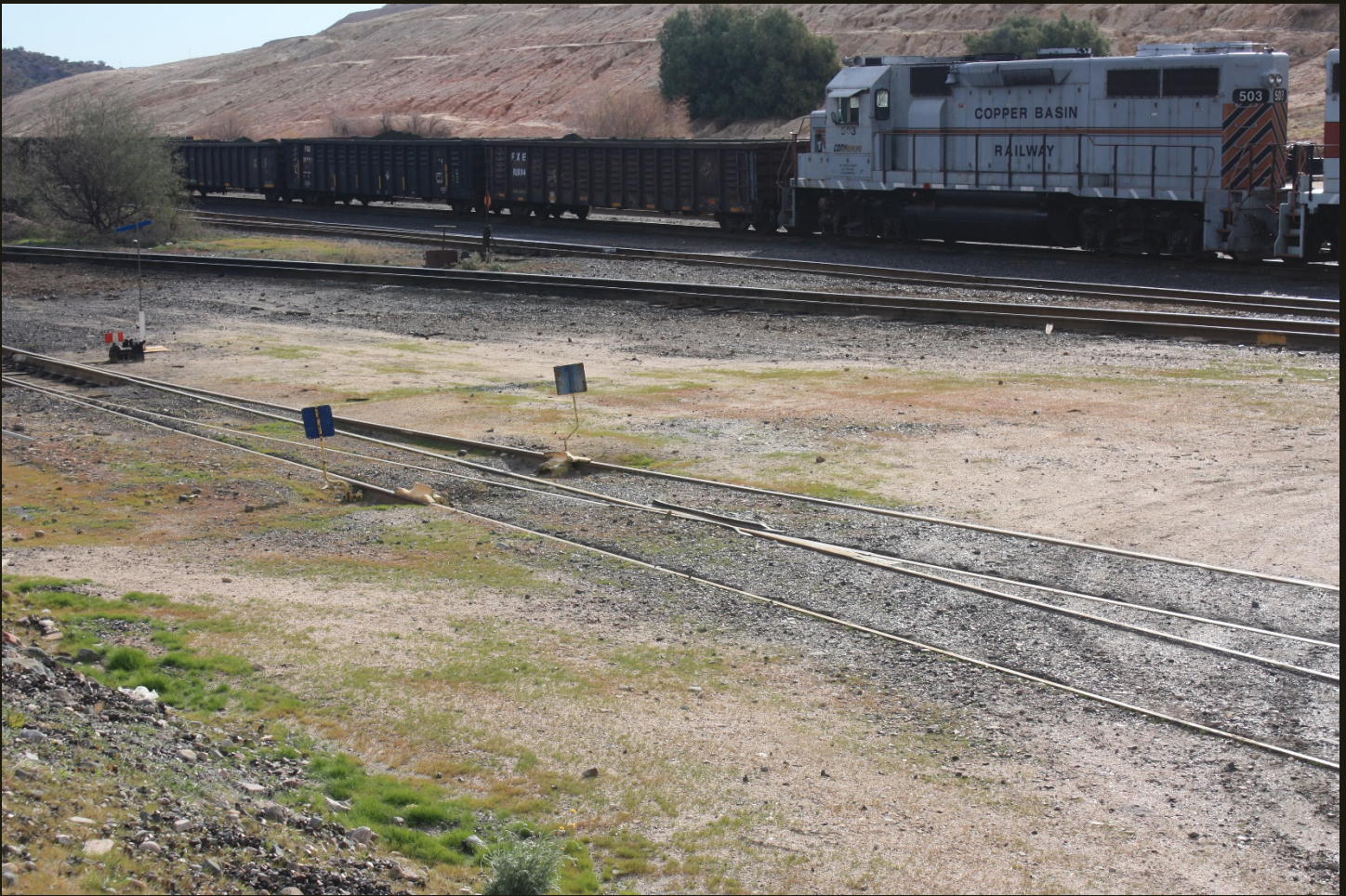
Southward view at Hayden Junction, a few steps north of the previous location. The same locomotives are on the P&E (1904) mainline with same siding parallel to it. The closer track, curving away from the mainline, is the 1911 R&GV spur to the Hayden smelter. The closest track leads to the locomotive maintenance facility and in this view splits into two tracks to enter the two doors for the facility.
