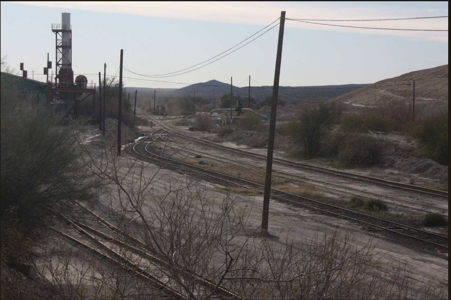
Southeastward view from the same location. The track on the left and in the foreground is the P&E (1904). It is splitting into two tracks that lead to a rolling stock facility that is obscured by the bush on the far left (it is visible in the next photo). The track on the right with two sidings is the SMA (1955); the closest siding is a short spur that ends just to the right of this photo (thus it is not within the previous photo). Note the smokestack between the two railroads.
