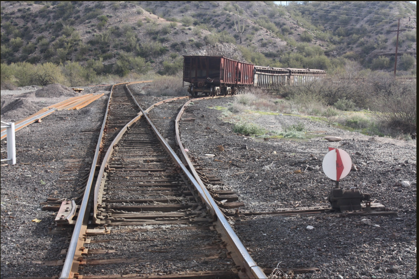
Eastward view 1911 R&GV spur to the Hayden smelter, same location as previous. The track that splits off to the right is a 1,000-foot spur for car storage. The DOT crossing sign (the 1911 R&GV spur crosses Arizona Highway 177 at this location) identifies this railroad as the CB "Hi-Line," which is apparently the CB's name for the higher-elevation spur to the smelter.
