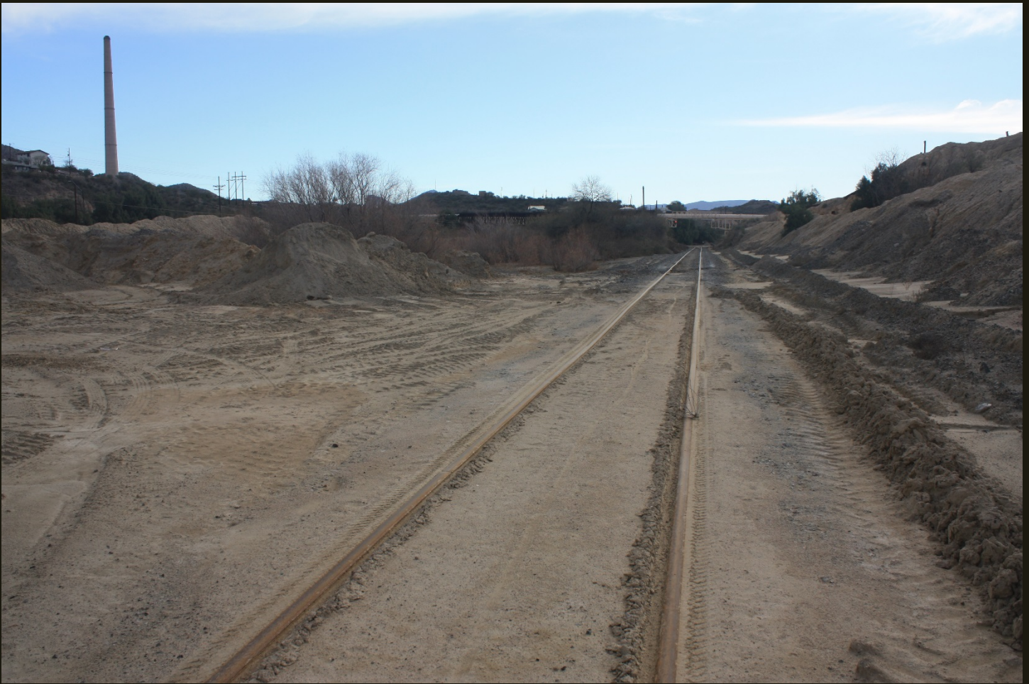
Southeastward view of the P&E (1904), same location as previous. Tailings that have washed onto the tracks and then cleared away are piled up on the left. The smokestack on the left is the Hayden smelter; the stack is located at the end of the 3-mile spur to the smelter. Note the conveyance piping over the track in the distance.
