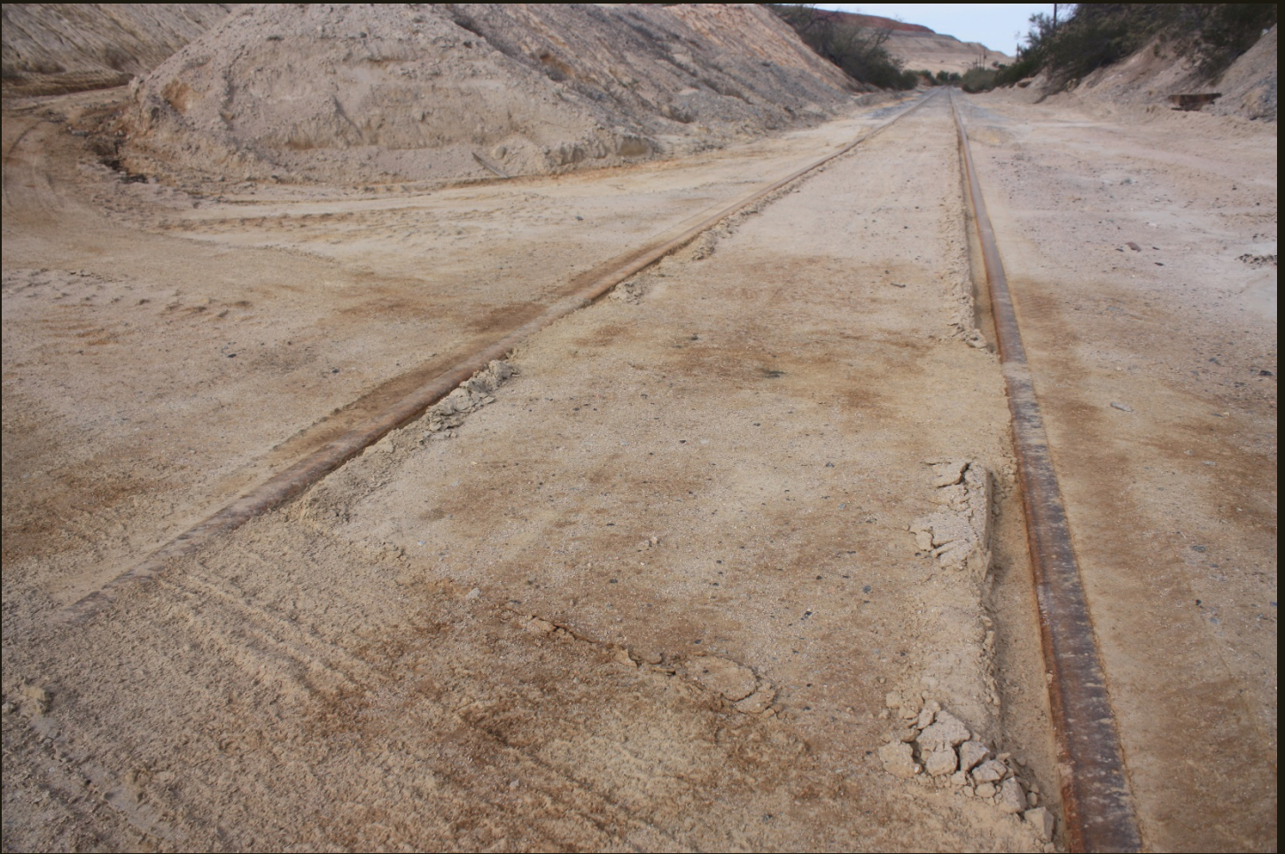
Now we are one mile southeast of the previous location looking northwestward at the P&E (1904). The slope to the left is the same tailings pile that surrounds the open pit mine; tailings have washed down onto the tracks but the CB keeps the tracks clear.
