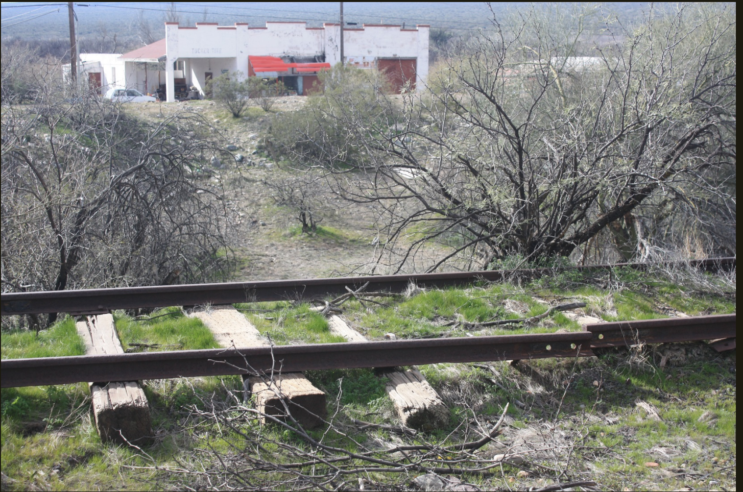
Southward view of the siding for the loading ramp, same location as previous. The P&E (1904) grade is evident in front of the building with the red awnings.
