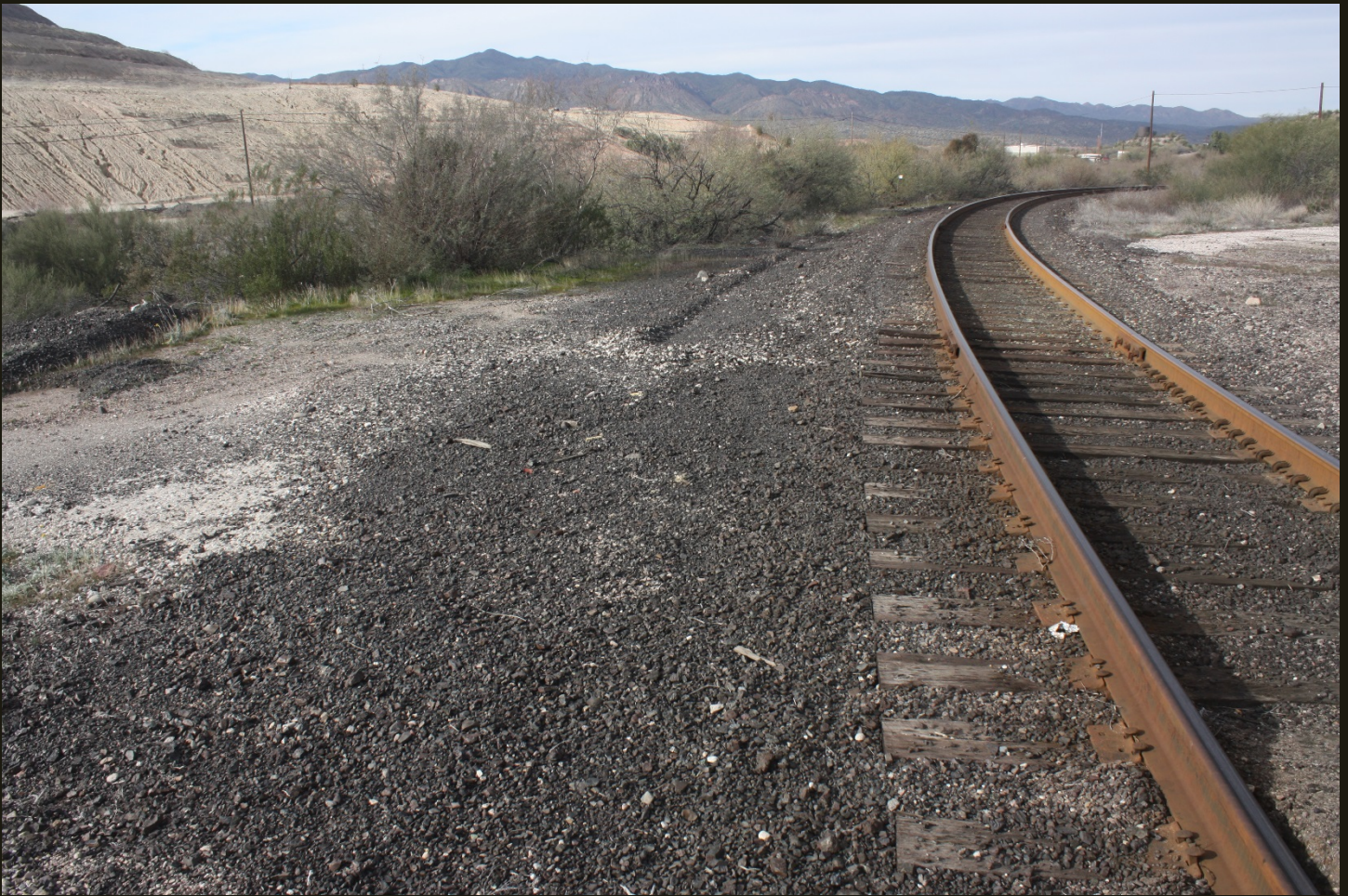
Westward view of the 1911 R&GV spur to the Hayden smelter, 1,500 feet east of the previous location. The more prominent white building in the right distance is the CB locomotive maintenance facility and the smaller buildings to its right are the CB headquarters. The P&E (1904) mainline is not quite visible at the base of the tailings pile to the left, but it is clear in this view that the spur to the smelter is at a higher elevation as it climbs off the floor of the Gila River Valley to the Hayden smelter.
