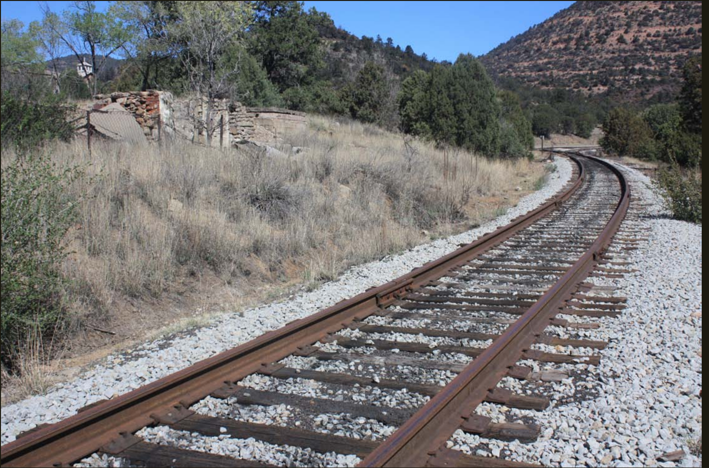
Northward view of the inactive SC&N branch at the abandoned town of Fierro, with a defunct loading facility to the left.
