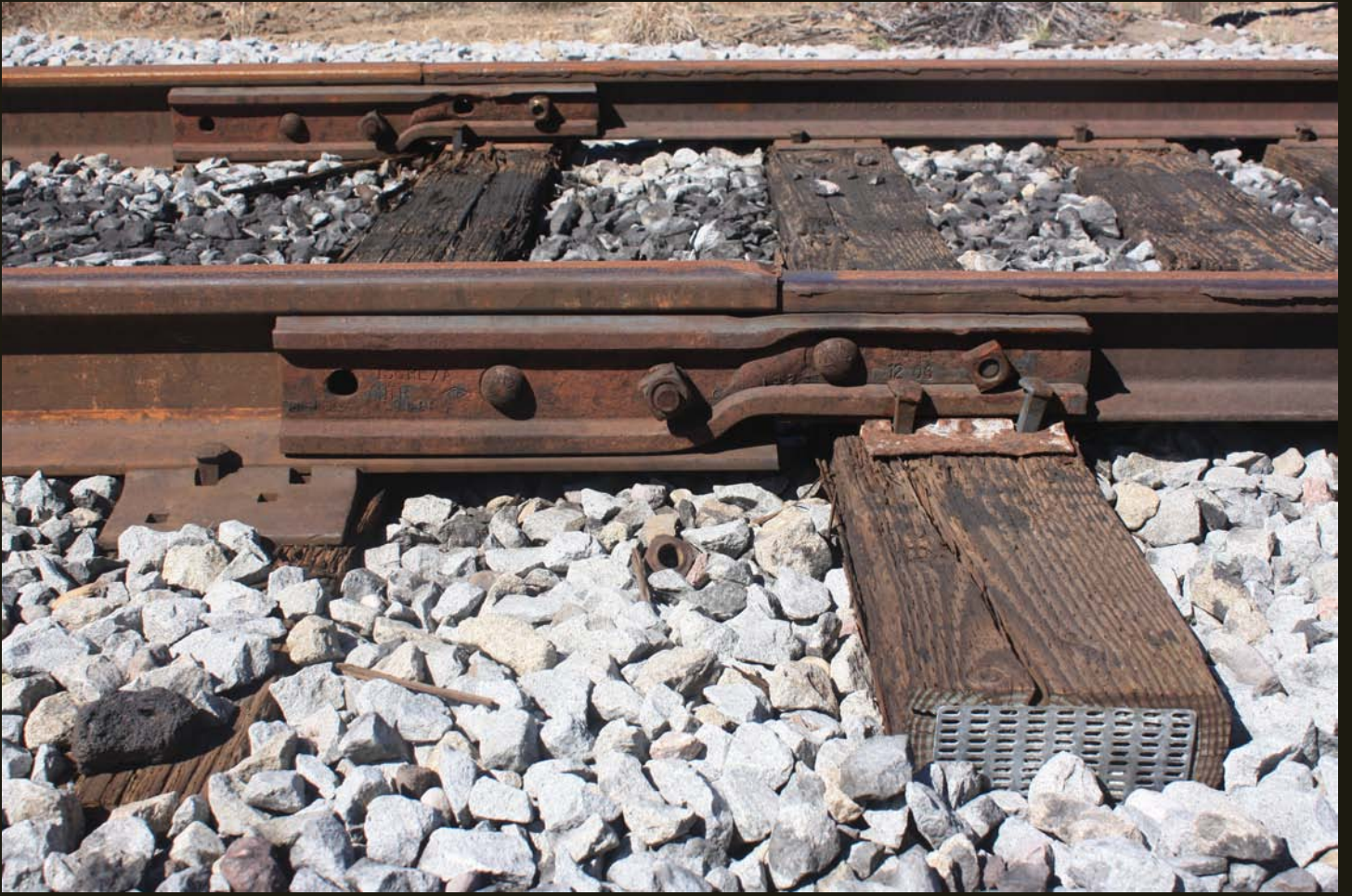
Change of rail weight at the SC&N Fierro siding.
