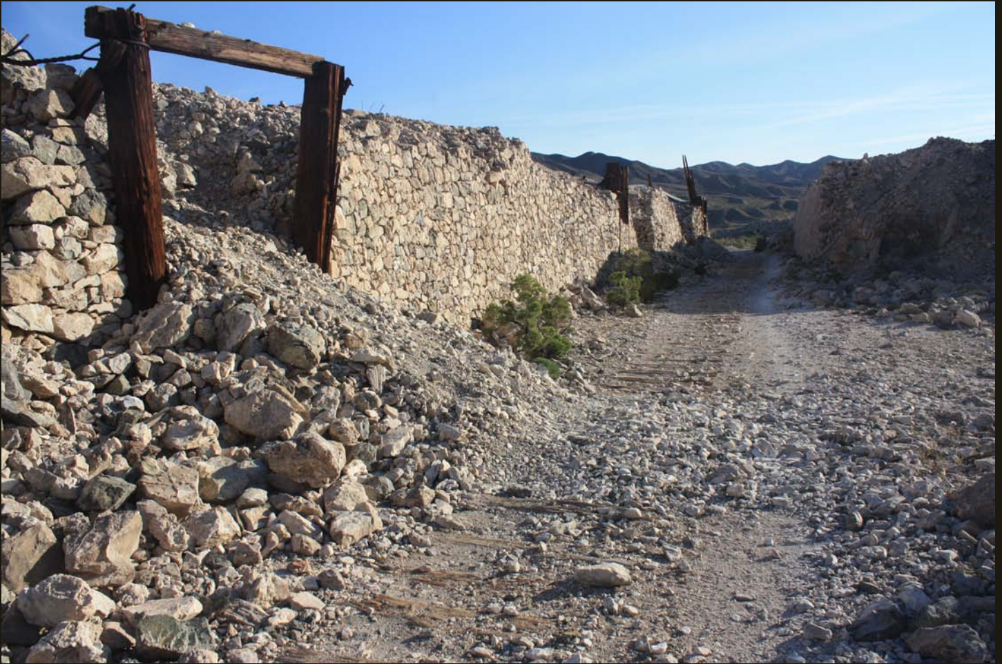
At the east end of Afton Canyon, an abandoned mining operation once had a loading facility with some sort of rail spur, as indicated by the ties. This rail grade goes from this loading area a few hundred yards to the SPLA&SL mainline, which is out of sight in the distance.
