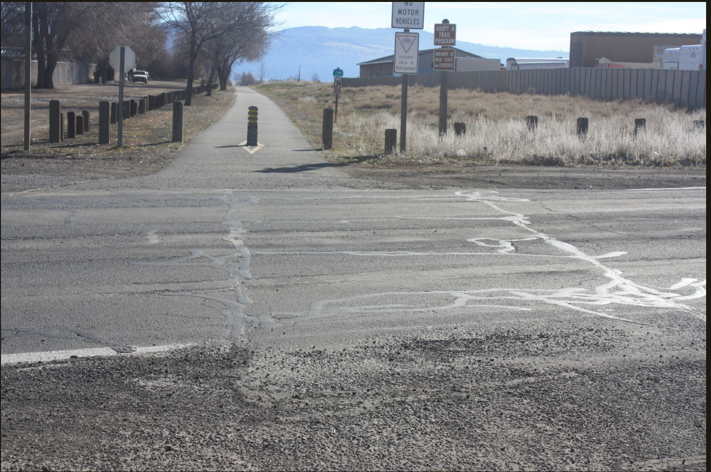
Eastward view of the OC&E grade, now the OC&E Woods State Trail, at the same location as previous photo. Note pavement patching where rails were removed.
