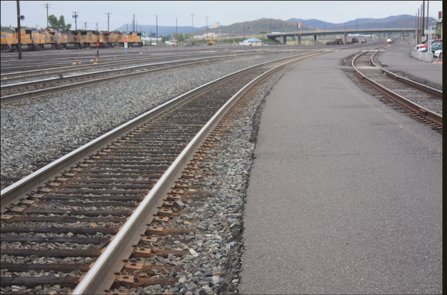
Southward view of the Klamath Falls rail yard, steps from the depot.
