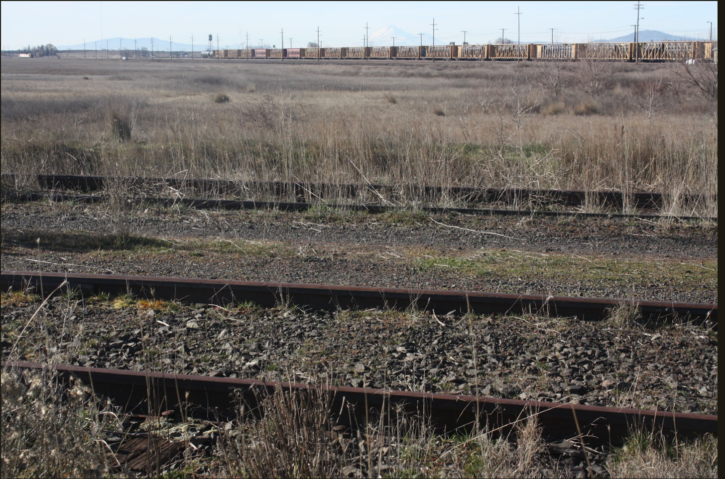
Southwestward view of the OC&E abandoned tracks and the active C&NE (1912) with stored cars for lumber products.
