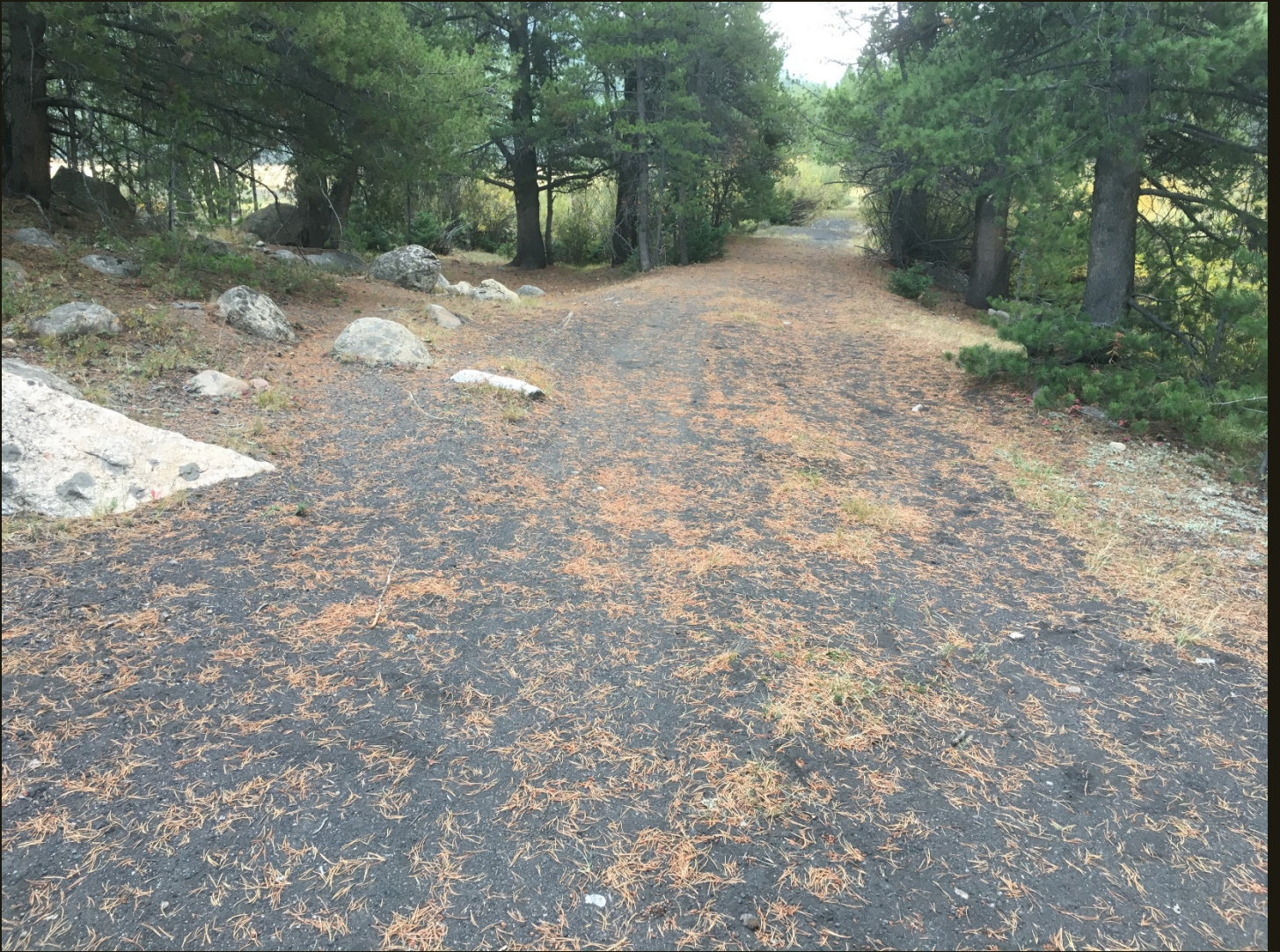
Southeastward view of the west branch of the wye from the same location as previous.
