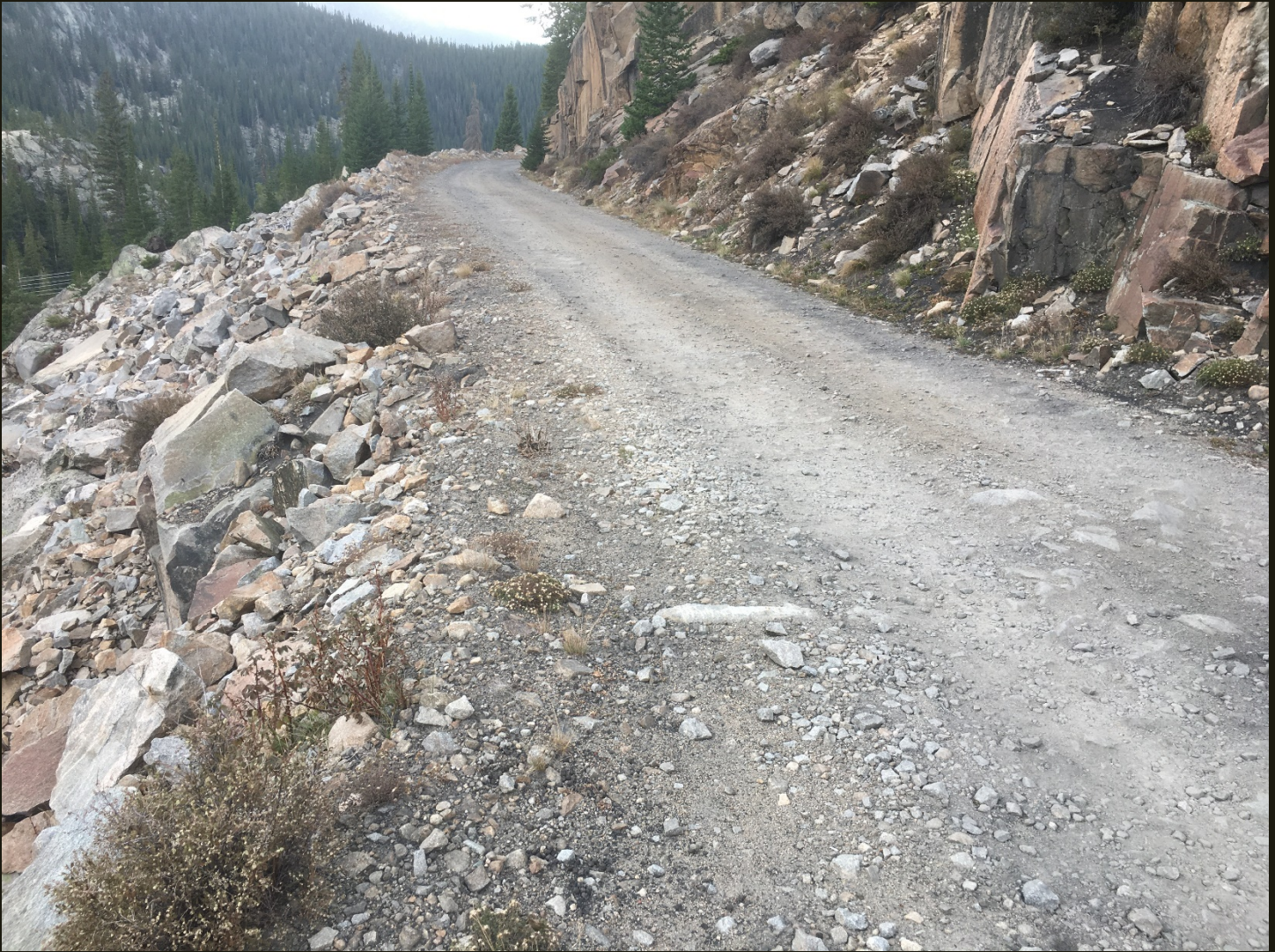
Westward (downgrade) view of a cut grade for the CM (1888) 3,500 rail feet east of the previous location. The valley to the left is Ivanhoe Creek, a tributary of the Fryingpan River.
