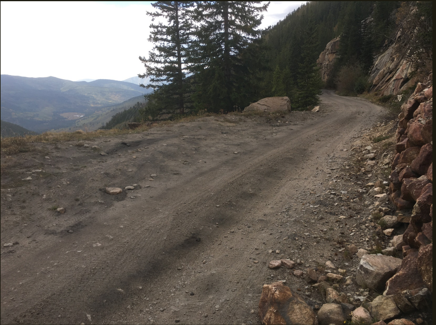
Westward (downgrade) view of a cut grade for the CM (1888) 4 rail miles southeast of the previous location. The valley to the left is the Fryingpan River; from here it is easy to see how much elevation has been gained.
