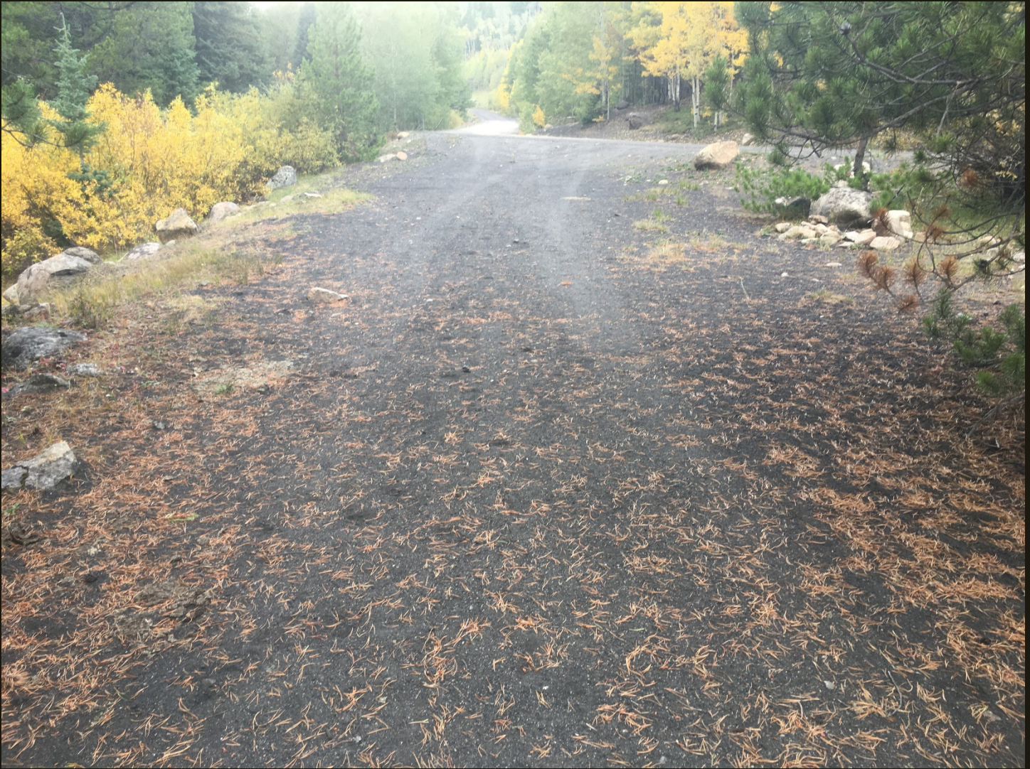
Northwestward view of the CM (1888) 1.25 rail miles upgrade from the previous location. The well graded road in the distance that goes out of the frame on the right is the CM mainline. We are looking downgrade, having made another U turn since the previous location (there, northwest was upgrade). The gravel opening in the foreground is the west branch of a wye.
