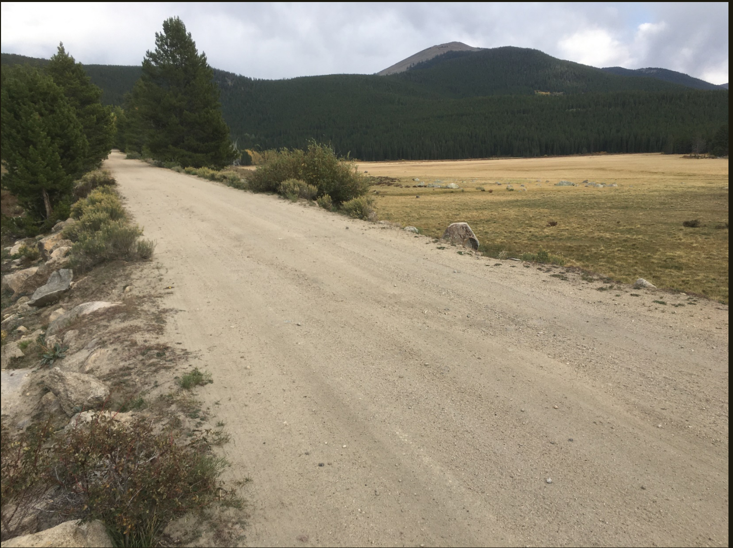
Eastward view of the CM (1888) at the same location as previous. The CM (1888) crosses Sellar Meadow via a significant fill grade. The continuation of the route is visible as the cut grade that climbs the wooded slope beyond the meadow.
