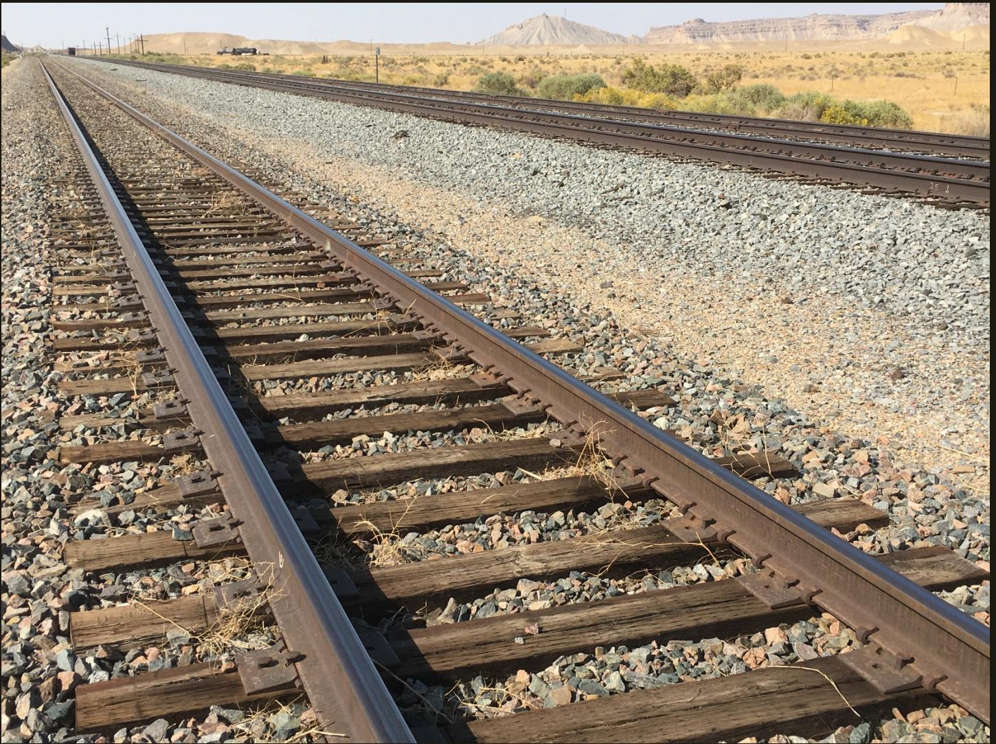
Westward view at the same location as previous. The Cane Creek Branch (1963), which is the welded track in the foreground, runs parallel to the mainline for 1,200 feet.
