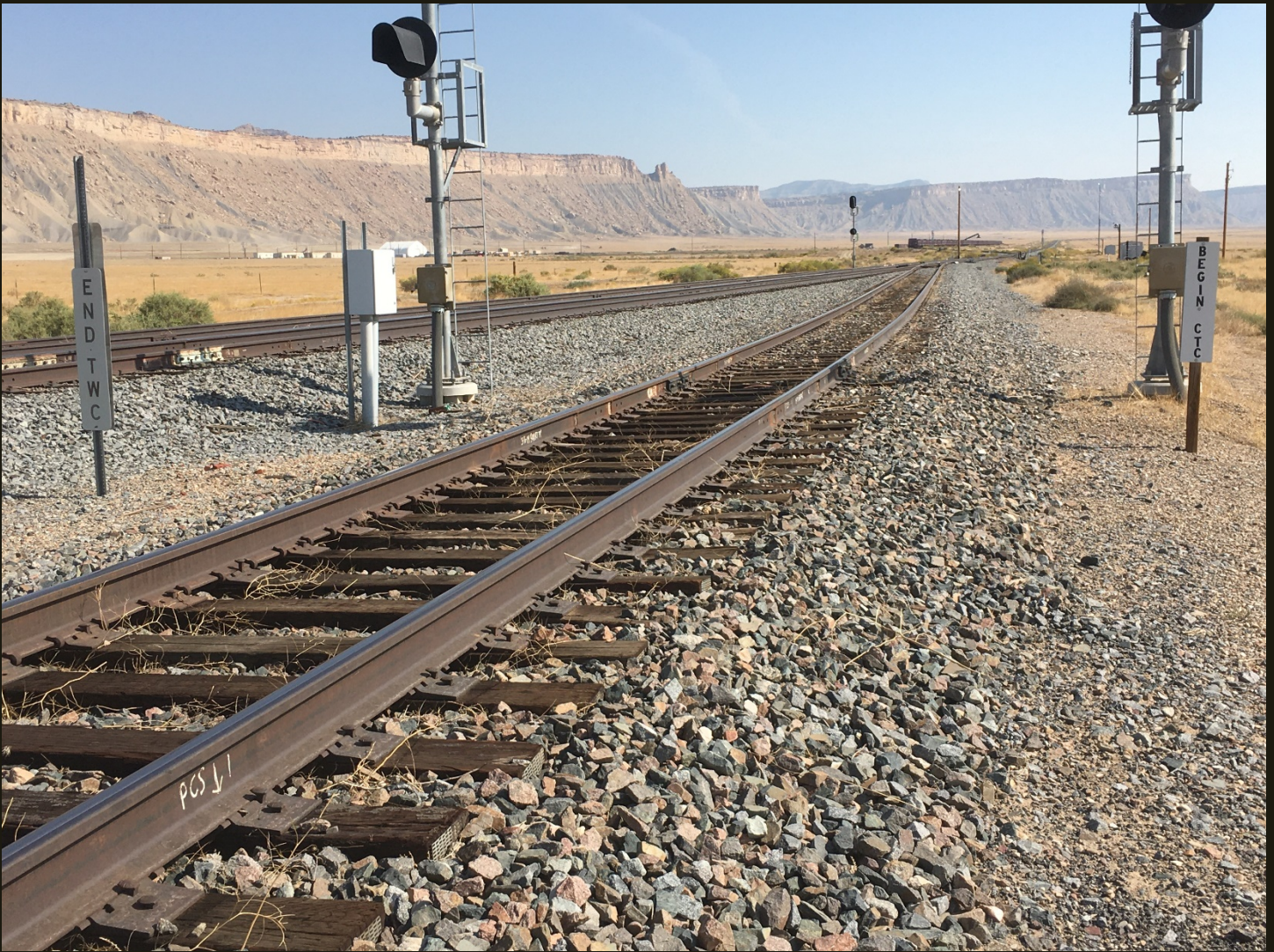
Eastward view 300 feet West of the previous location. The tracks are, from right to left, the D&RGW Cane Creek Branch (1963), which joins the D&RGW (1883n) mainline in the distance, and the rusty siding on the far left.
