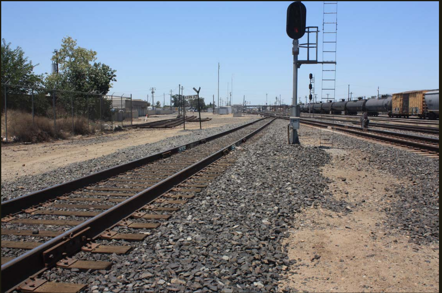
Westward view of the MS line (left) and the SP (now UP) Bakersfield yard with stored oil tank cars. Note the older bolted track of the MS.
