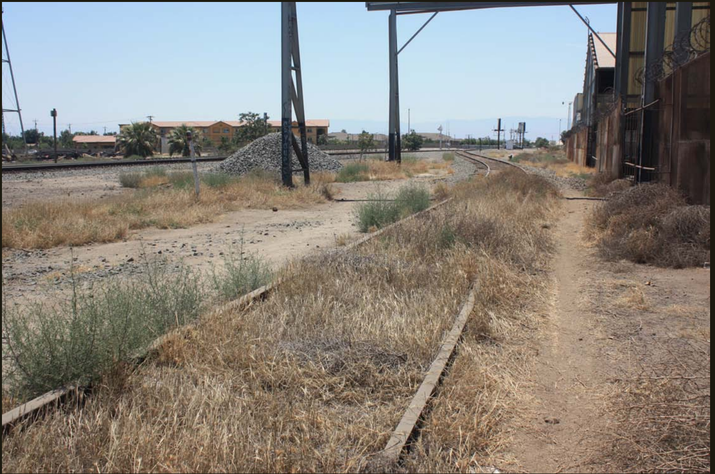
Southward view of an abandoned siding on the MS line, just south of the wye with the SP (now UP).
