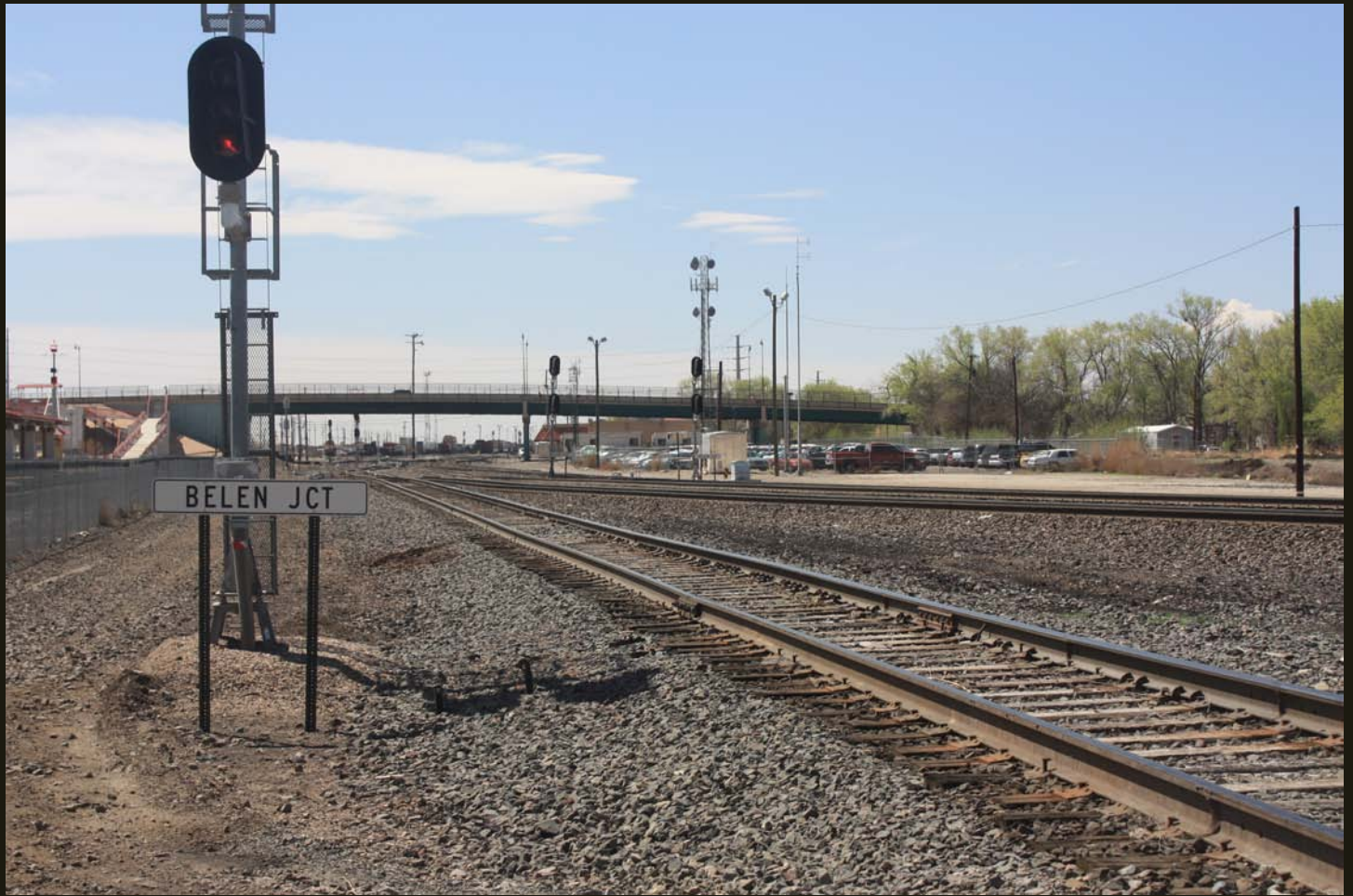
Southward view at same location as above, where the 1881 AT&SF Rio Grande-El Paso line is the bolted track in the center, the ERNM comes in from the right, and the Amtrak siding is across the fence on the left.
