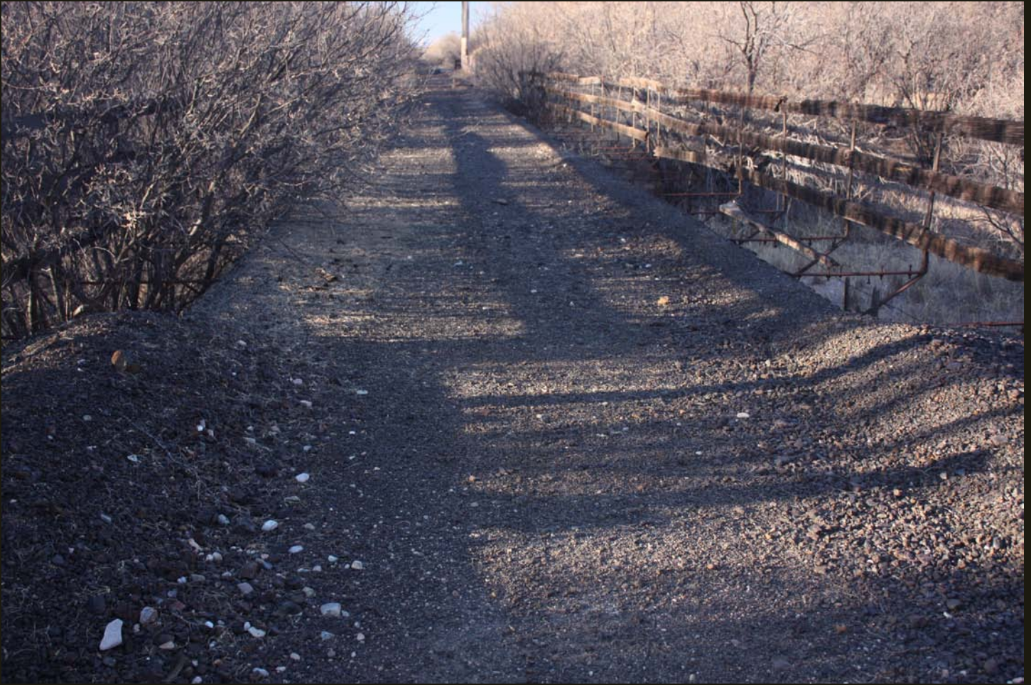
Northward view of the SP&SW grade the on the A&SE (1889) alignment where it crosses a small wash about 500 feet southwest of Fairbank. Note the black slag ballast from the Bisbee mines, typical of EP&SW construction.
