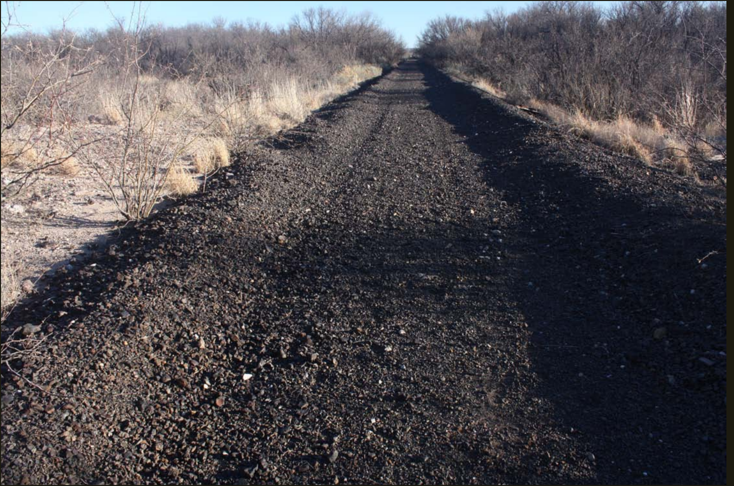
Southward view of the SP&SW/A&SE (1889) grade, same location as previous.
