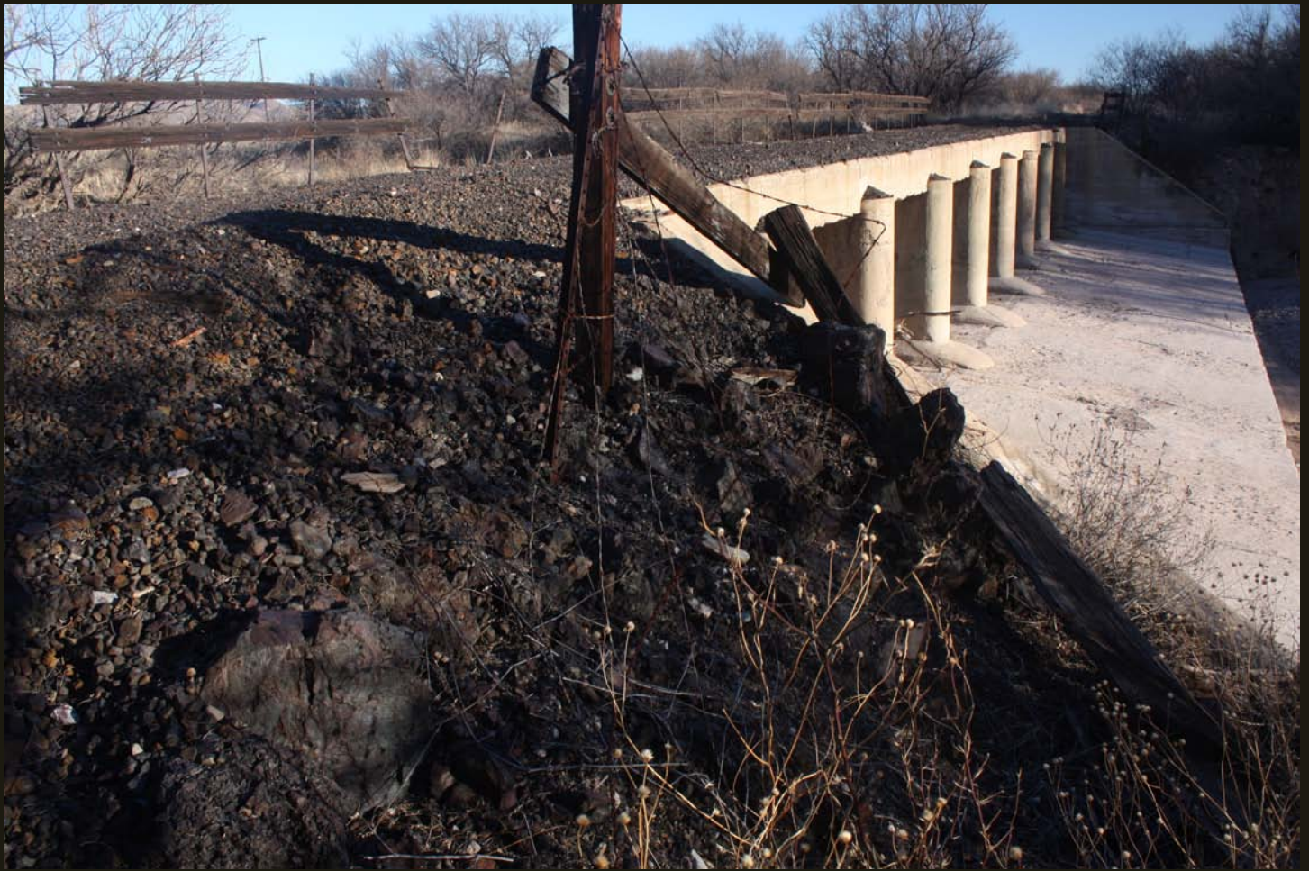
Southward view of the SP&SW/A&SE (1889) grade 600 feet south of the previous location and 1,000 feet south of Fairbank. A concrete bridge carries the grade over Walnut Gulch, which enters the San Pedro River a quarter mile west (right) of this location. The EP&SW Tombstone Branch (1903) generally follows Walnut Gulch from Fairbank to Tombstone.
