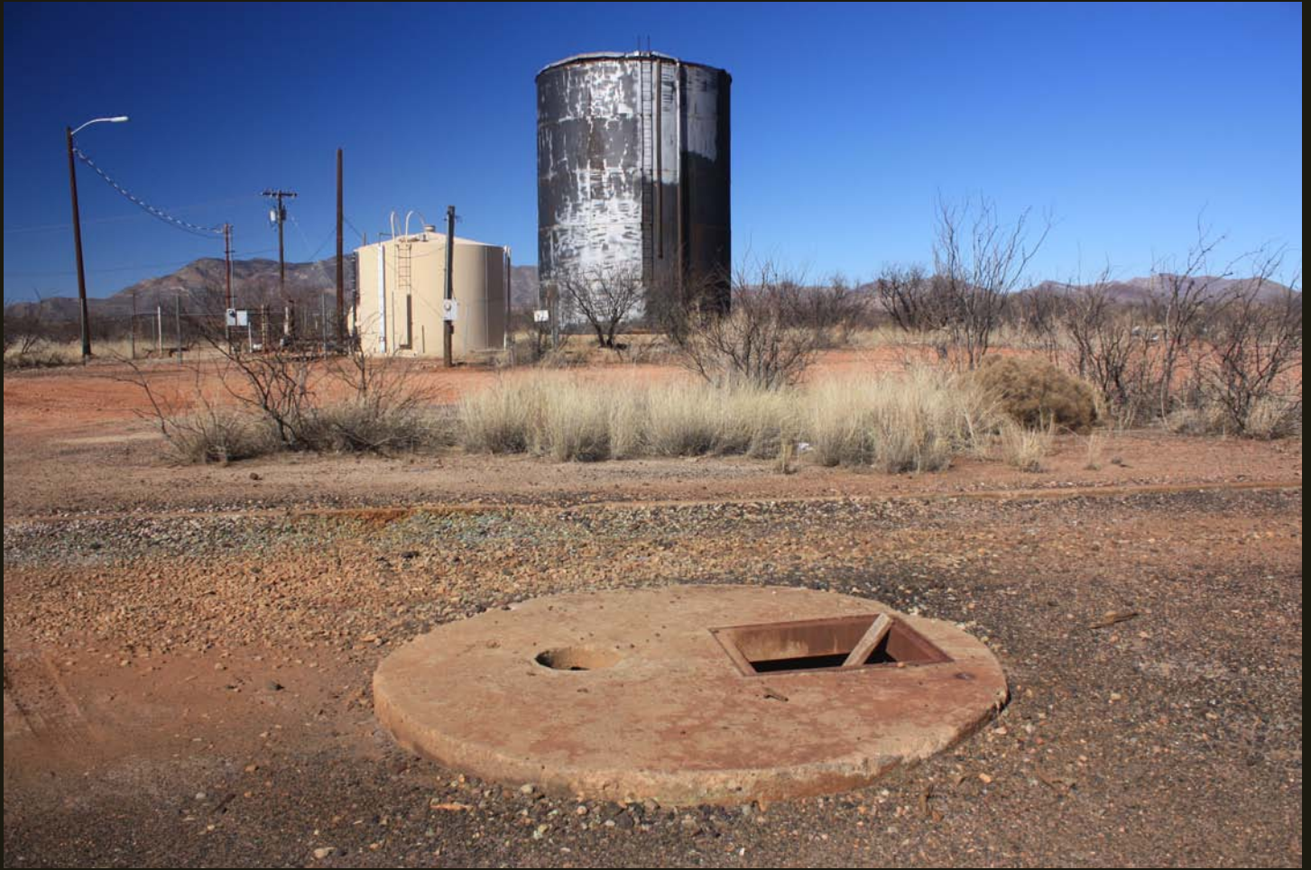
Northward view of the abandoned yard is Bisbee Junction. Same water tank as before. Old curbs and covered vaults raise more questions than they answer.
