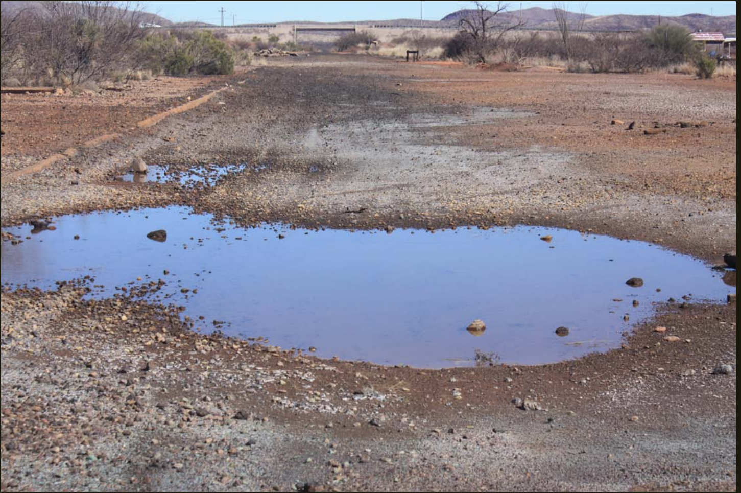
Eastward view of the east end of the abandoned yard at Bisbee Junction. This is the point at which the EP&SW commenced its eastward construction to El Paso in 1901 and is likely when the wye was laid out. Note the bridge that separates the EP&SW (1904) railroad grade from that of South Bisbee Junction Road.
