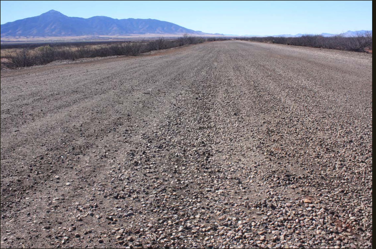
Westward view from the west end of the abandoned yard at Bisbee Junction. This is on the EP&SW (1904) re-alignment.
