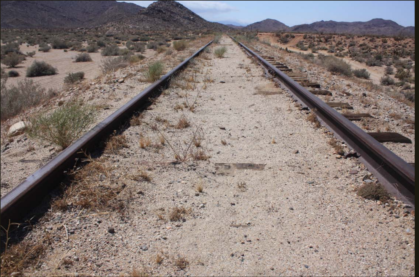
Westward view of the SD&A at Dos Cabezas.
