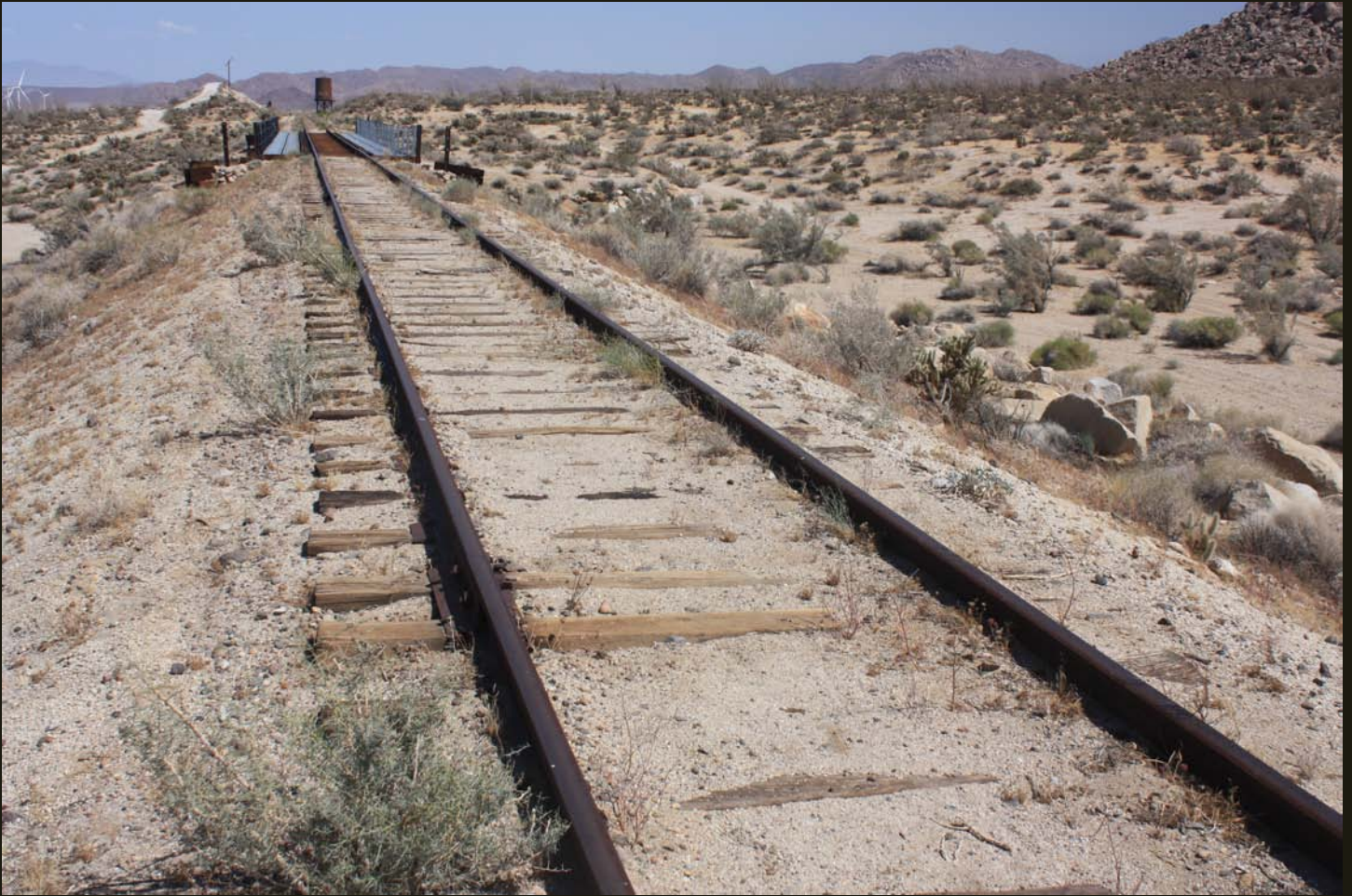
The water tower and trestle at Dos Cabezas, which is at the end of a four-wheel drive road.
