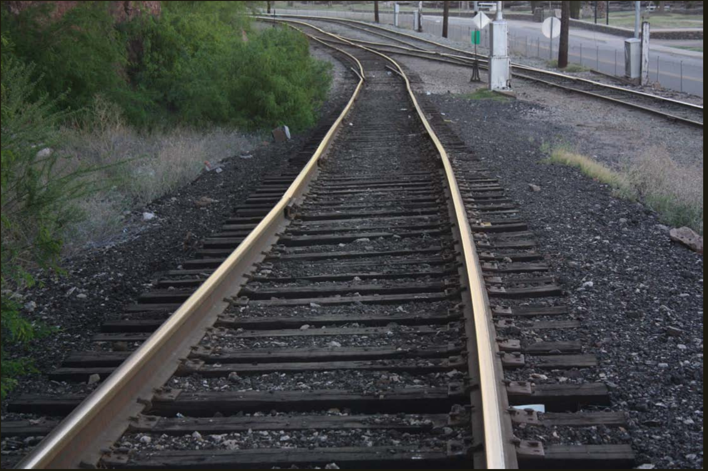
Another northward view of the connection between the MS (foreground) and the A&NM. Note the open switch that goes nowhere; I guess this is intended to derail a runaway train before it plunges into the highway.
