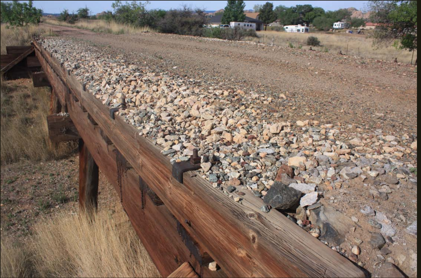
Southward view of the small SFP&P bridge over a gulley at Granite Dells. The tracks were removed in 1984.
