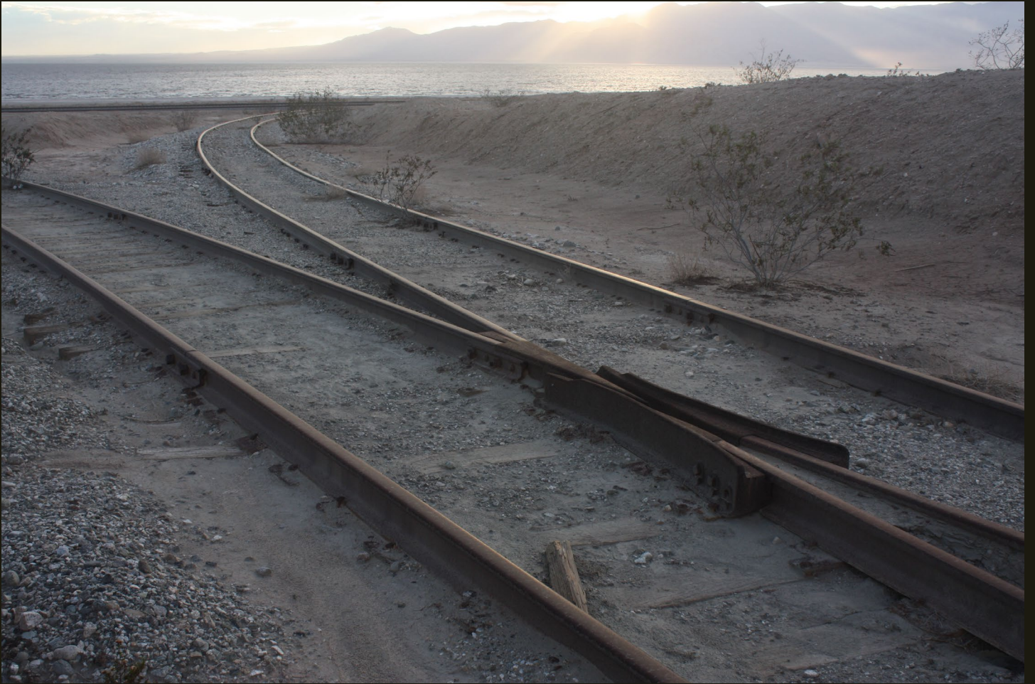
Northwestward view of the Ferrum turning wye.
