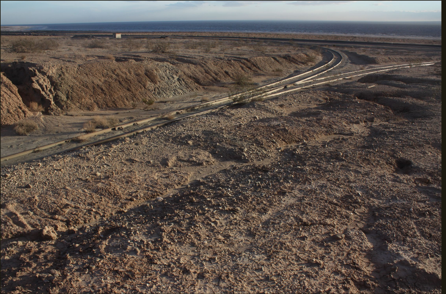
Southwestward view of the Ferrum turning wye.
