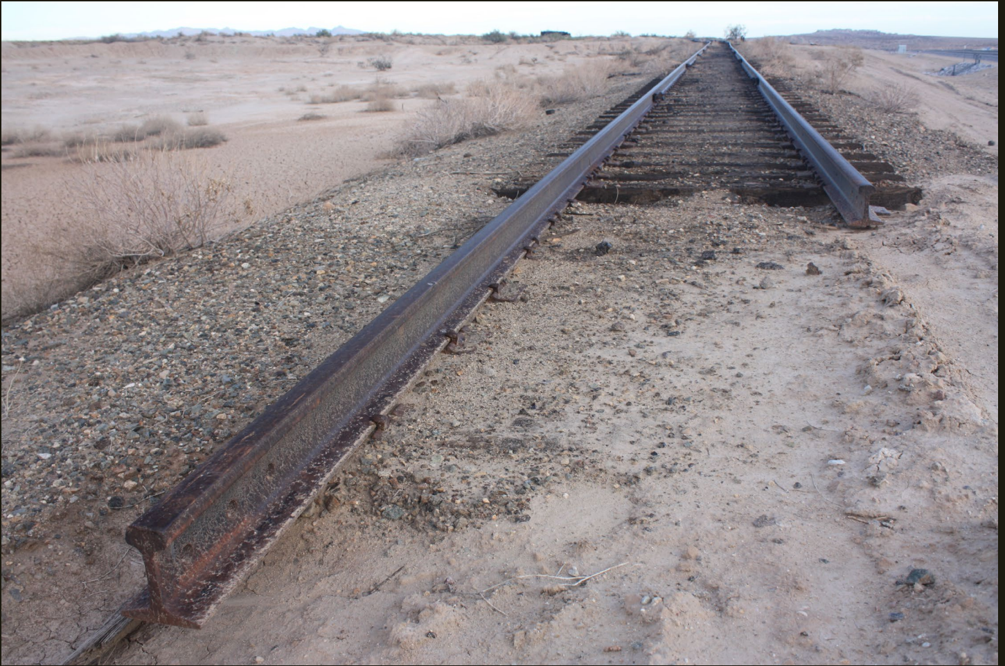
Southeastward view of the EM (1948) mainline as it enters Ferrum, same location as previous.
