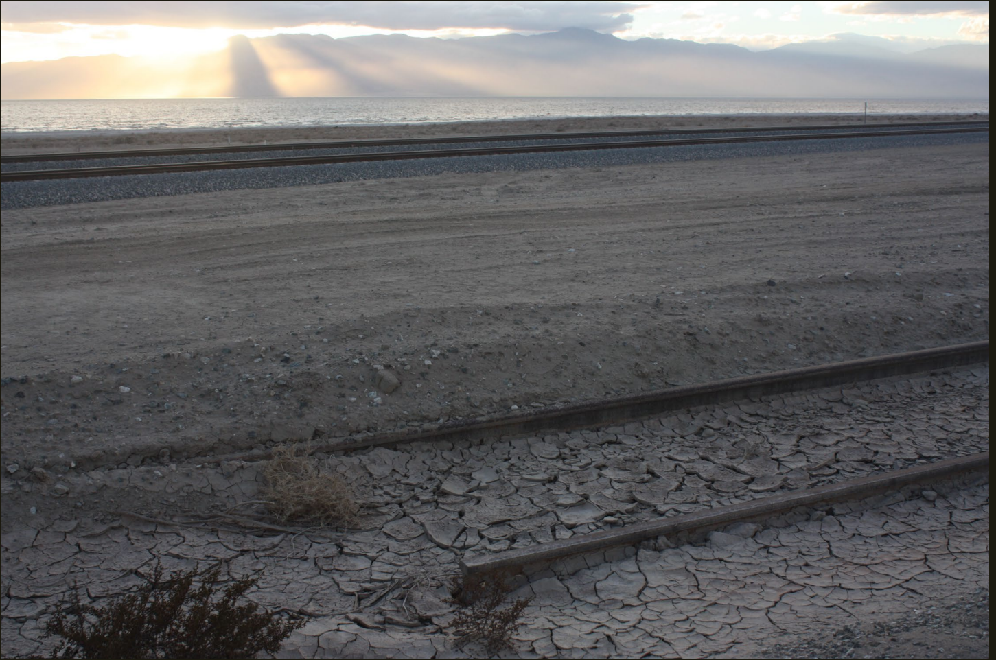
Northwestward view of the double-tracked SP Sunset Route (1906) mainline and the Salton Sea beyond. The track in the foreground is the southern branch of a turning wye for the EM (1948), which once connected to a siding. Ferrum was the location of a five track yard that once existed in the dirt area between the SP mainline and the wye. As of 2016, all the sidings have been removed but the wye is still in place, as seen here.
