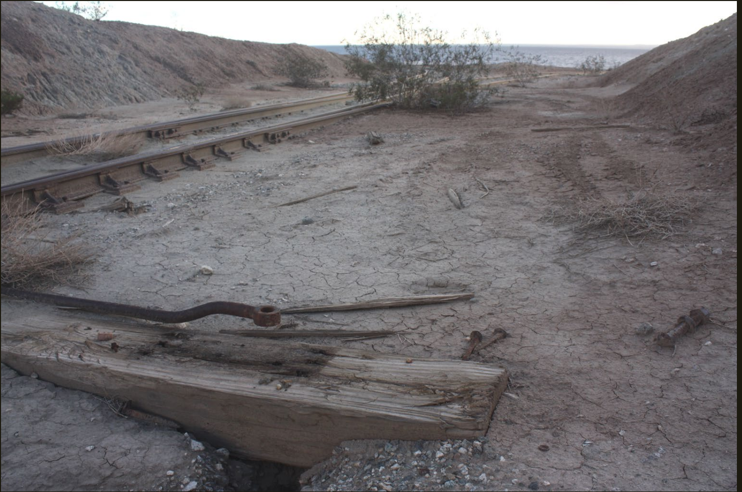
The switch at the tip of the Ferrum turning wye; note missing lever.
