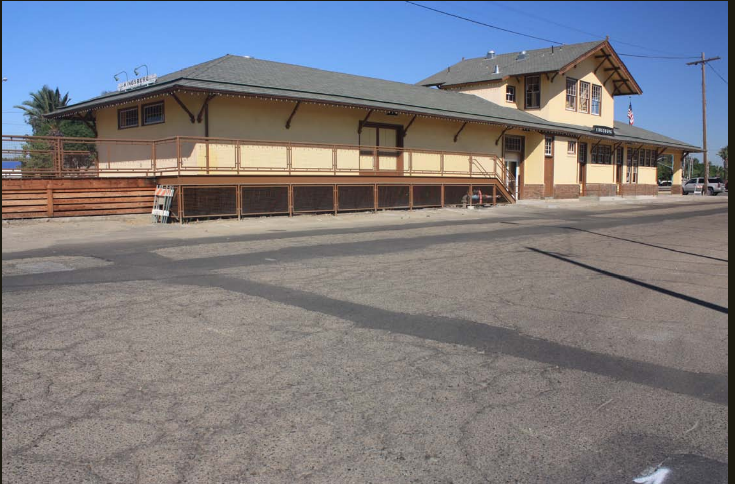
Street side of the Kingsburg Depot.
