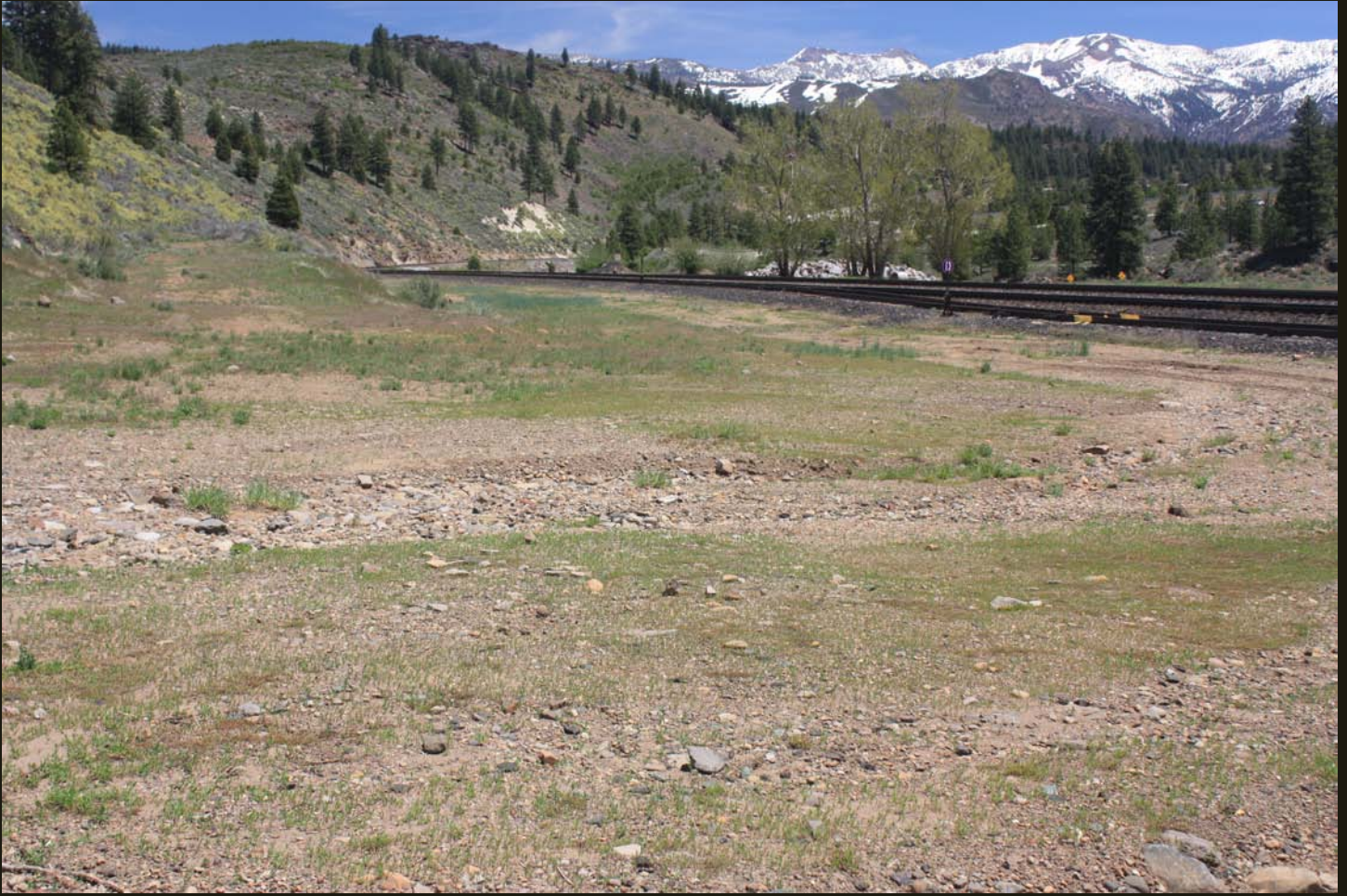
Closer eastward view of the switch to the SP ice spur and the B&L (1901) cut grade (far left) leading to a switchback. The snowcapped Carson Range in the distance diverts the Truckee River and the CP alignment due north for 10 miles, before turning east along the north side of the range toward Reno. Lake Tahoe, the source of the Truckee River, occupies the south (left) end of the intervening Valley.
