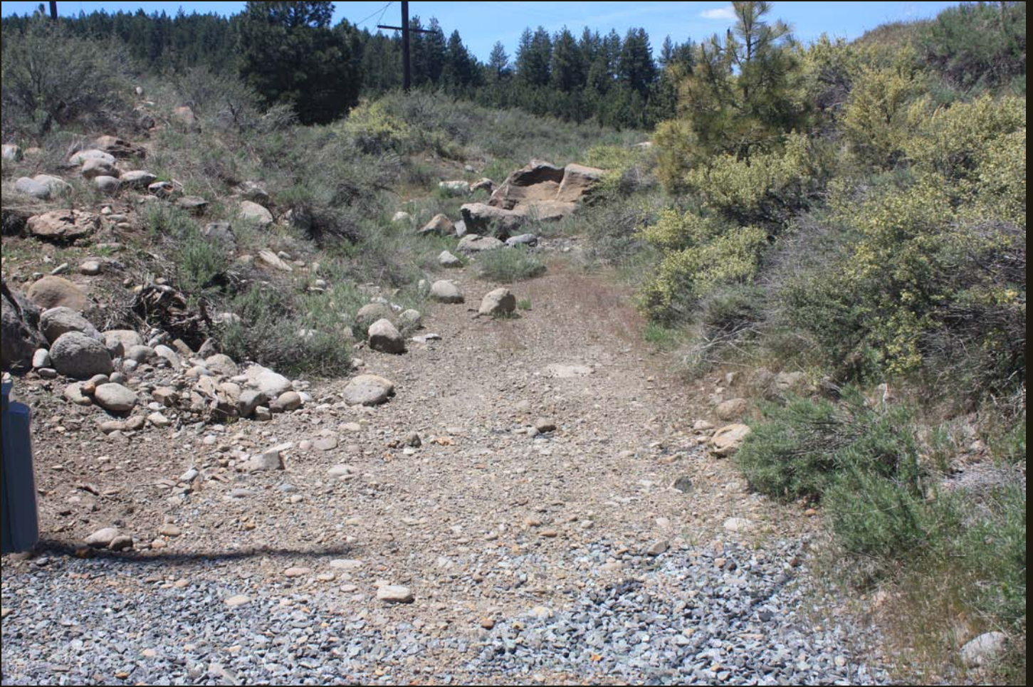
Northwestward view at the same location as previous. The SP ice spur began curving to the north in the gravel area in the foreground and through a shallow cut grade beyond.
