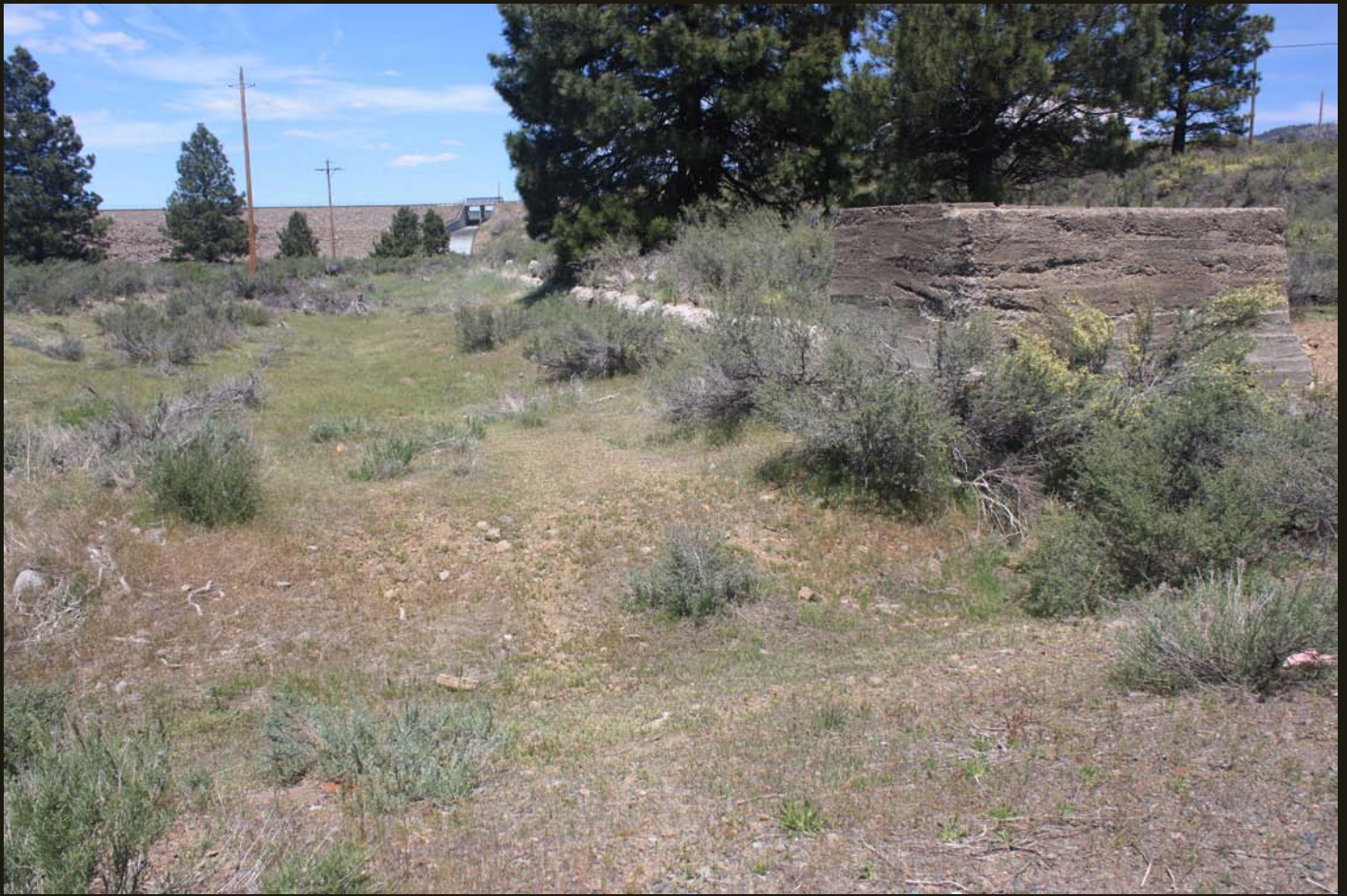
Northward view of the SP ice spur, which ran just to the west (left) of the foundations of an ice house in a slight cut grade. The ice ponds and north end of the spur were inundated by Boca Reservoir, whose dam across the Little Truckee River and spillway are visible in the distance. This foundation is 400 feet north of the CP/SP/UP mainline.
