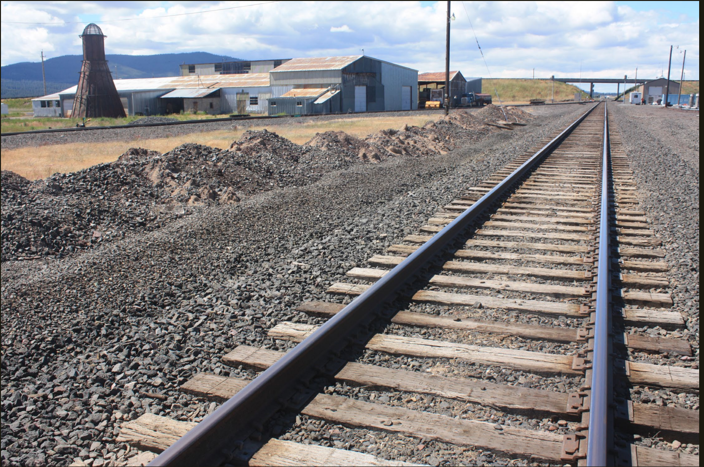
Southward view of the GN-WP Inside Gateway (1931) at Nubieber, same location as previous. Note the Nubieber siding converges with the mainline in the distance, where California Highway 299 crosses over the railroad grade, and lumber processing facilities are along the siding to the left (east).
