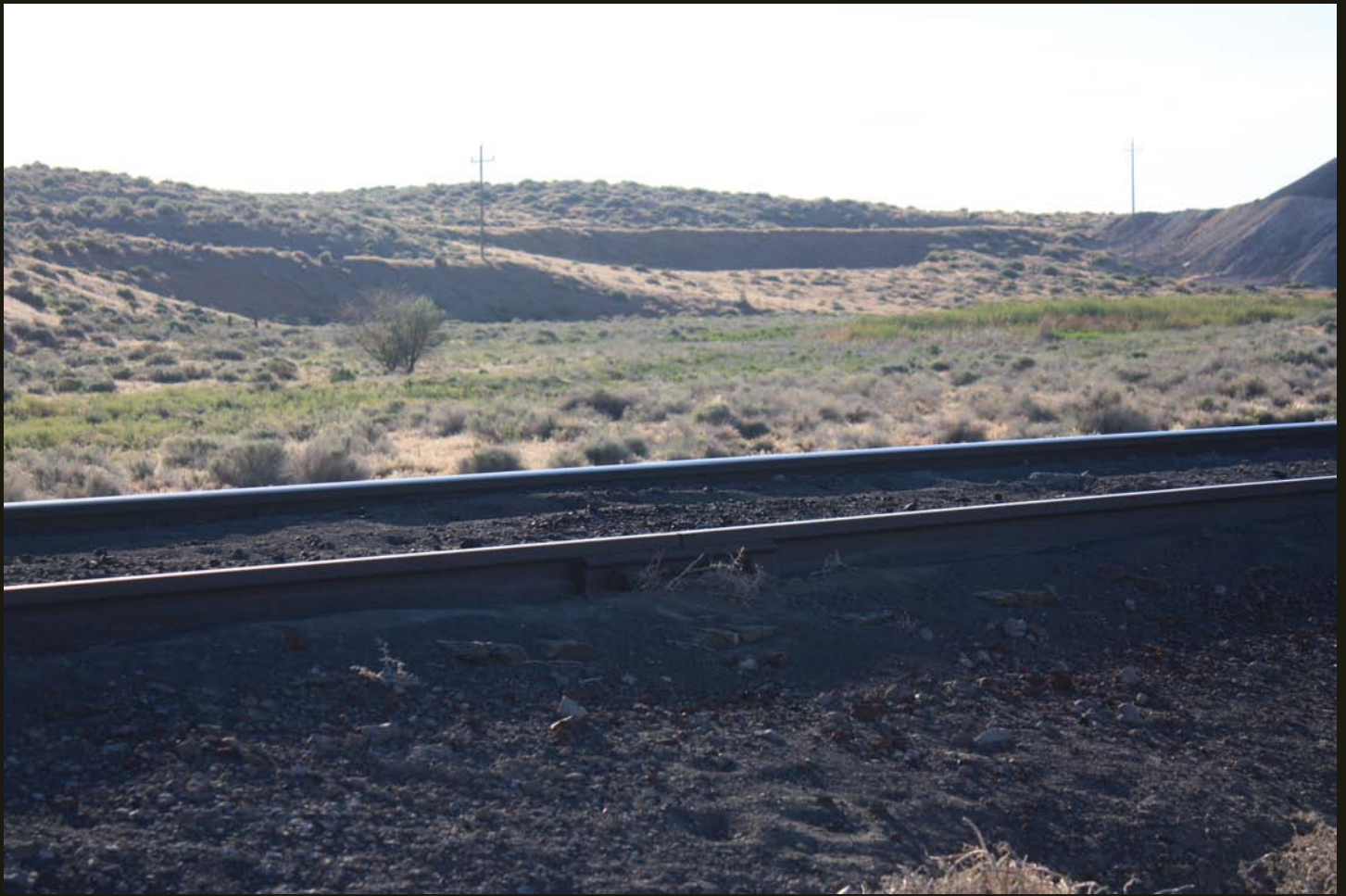
Eastward view of the F&L (1914), 2,000 feet southeast of the previous location, one mile southeast of the bridge, and 0.8 mile from the SP (1902) re-alignment. There is a major fill grade in the center distance and a tailings pile from the cement plant at the far right. The fill grade is not the CP (1869); instead, it is a temporary, one-mile-long connection from the CP (1869) to the SP (1902). It was built in 1902 and abandoned in 1906.
