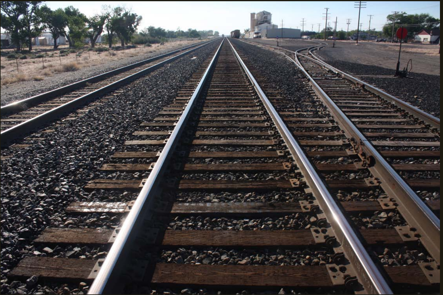
Southeastward view of the SP (1902) re-alignment at Fernley, same location as previous. The two straight tracks are the SP (1902). The track in the far right foreground is the same track that is in the left foreground of the previous photo; this track leads to sidings for the Celite Corporation, a current or recent rail customer. Note the very flat topography of the Lake Lahontan lake bed.
