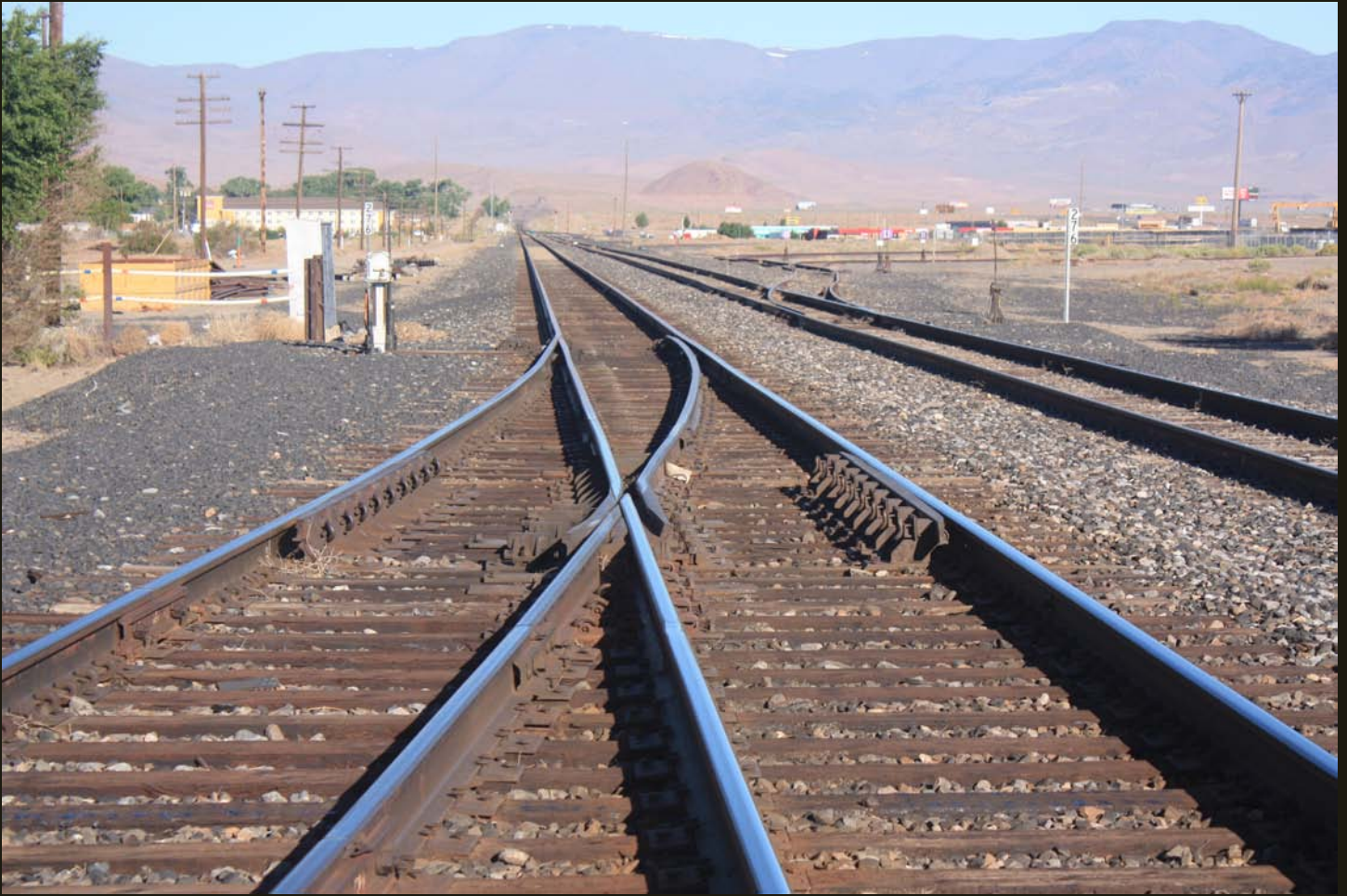
Northwestward view of the SP (1902) re-alignment (now UP) at Fernley, just east of the F&L (1914) wye. The two straight tracks are the SP (1902). The branch in the left foreground leads to sidings south of the mainline. The first switch on the right-hand track leads to two industrial spurs and beyond that is the switch to the east branch of the F&L (1914) wye, which is barely visible, and beyond that is the west branch of the wye, which is even less visible. The 8,000-foot peaks of the Pah Rah Range, another Basin and Range normal fault, still have some snow in late May.
