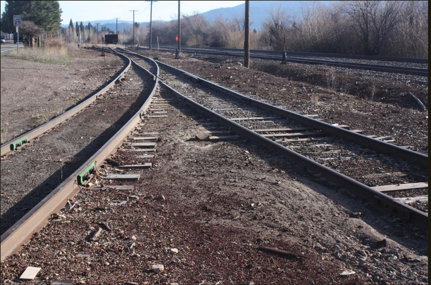
Switch and siding for the MR junction with the C&O (now Union Pacific) mainline, which is in the distance across a ditch.
