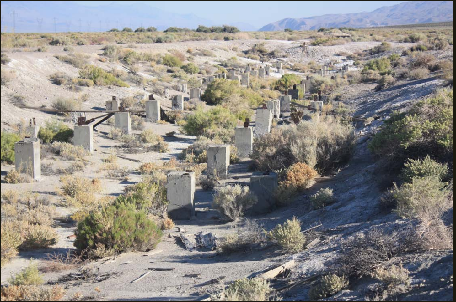
Northward view of foundations for the Owenyo Transfer Trestle, built in a basin at the south end of Owenyo. The standard gauge SP Jawbone Branch (1910) ran through the un-vegetated area on the far side of the basin and the narrow gauge C&C/N&C/SP ran just to the right of the photo. The trestle was used to transfer freight standard- and narrow-gauge rolling stock.
