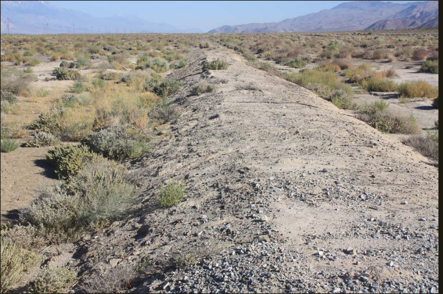
Northwestward view of the C&C/N&C/SP fill grade north of Owenyo, same location as previous.
