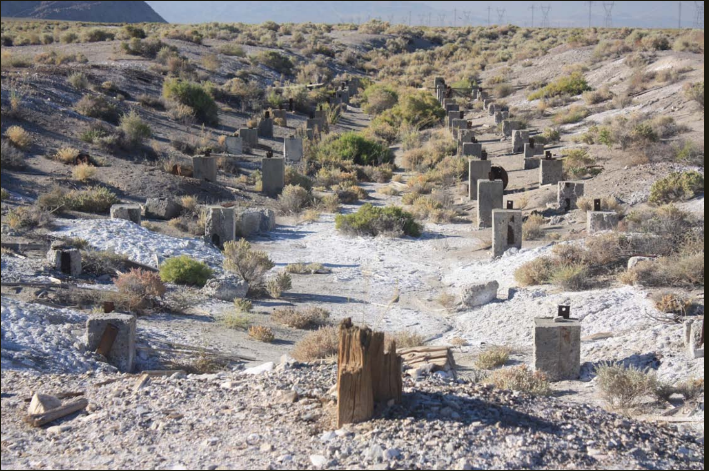
Southeastward view of the Owenyo Transfer Trestle. The standard gauge SP Jawbone Branch (1910) ran on the right (west) side of the basin and the narrow gauge C&C/N&C/SP ran to the left.
