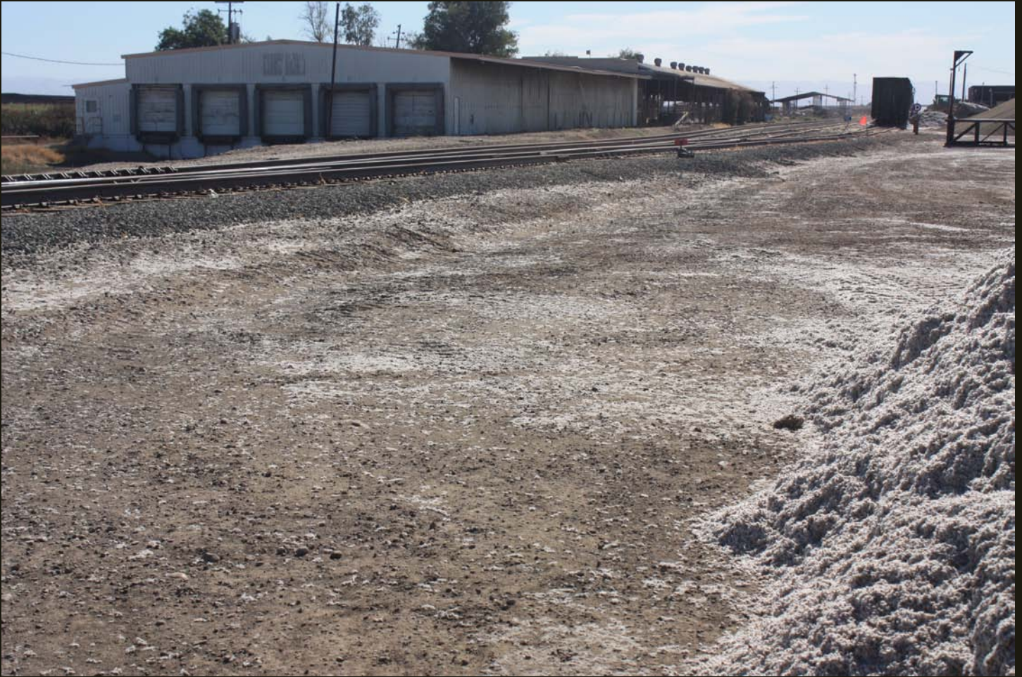
Westward view of sidings and loading facilities on the SW, which built through here in 1901, just west of the Connor 90. Note piled cotton in right foreground.
