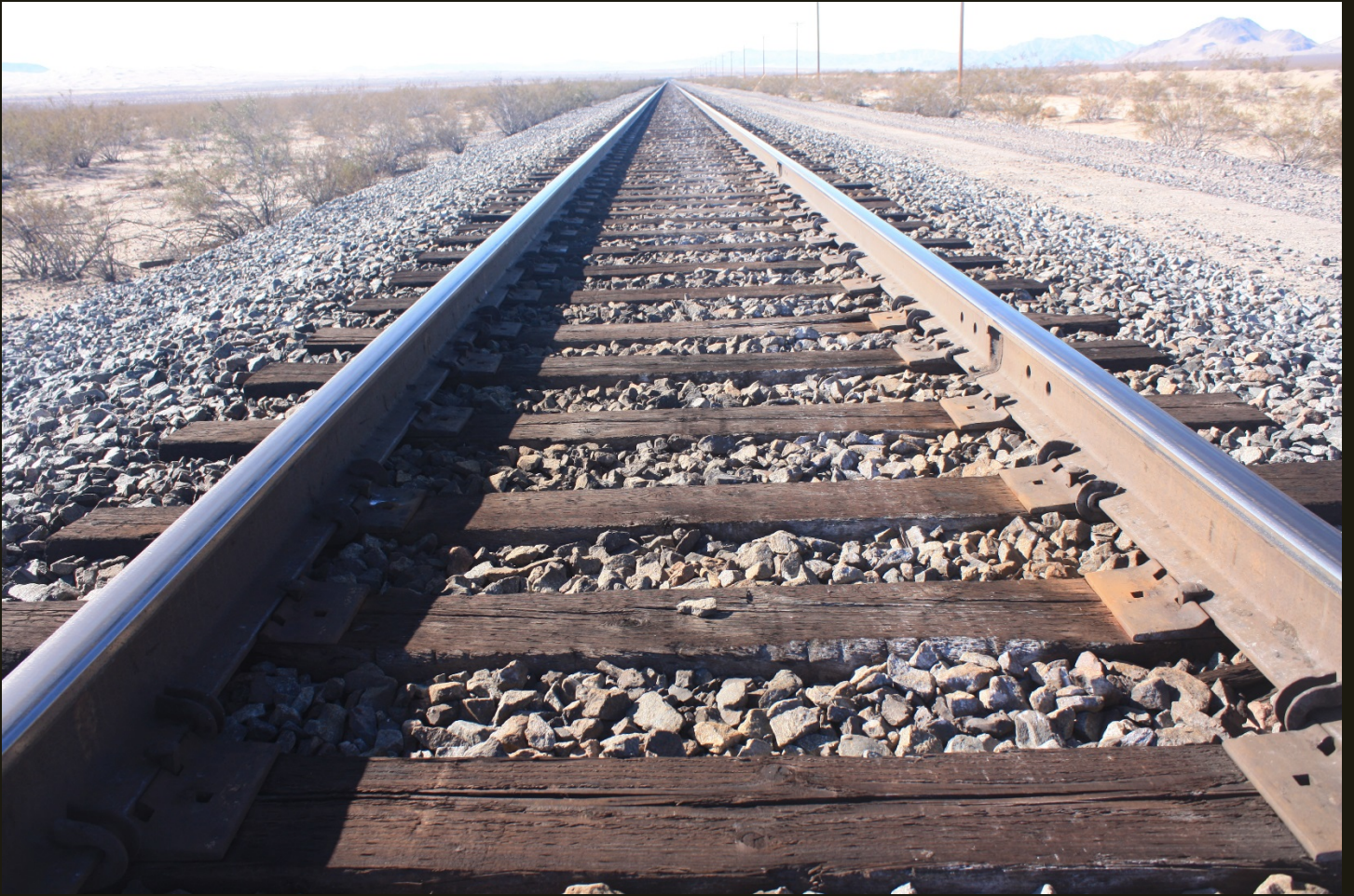
Southwestward view of the SPLA&SL (1905), same location as previous.
