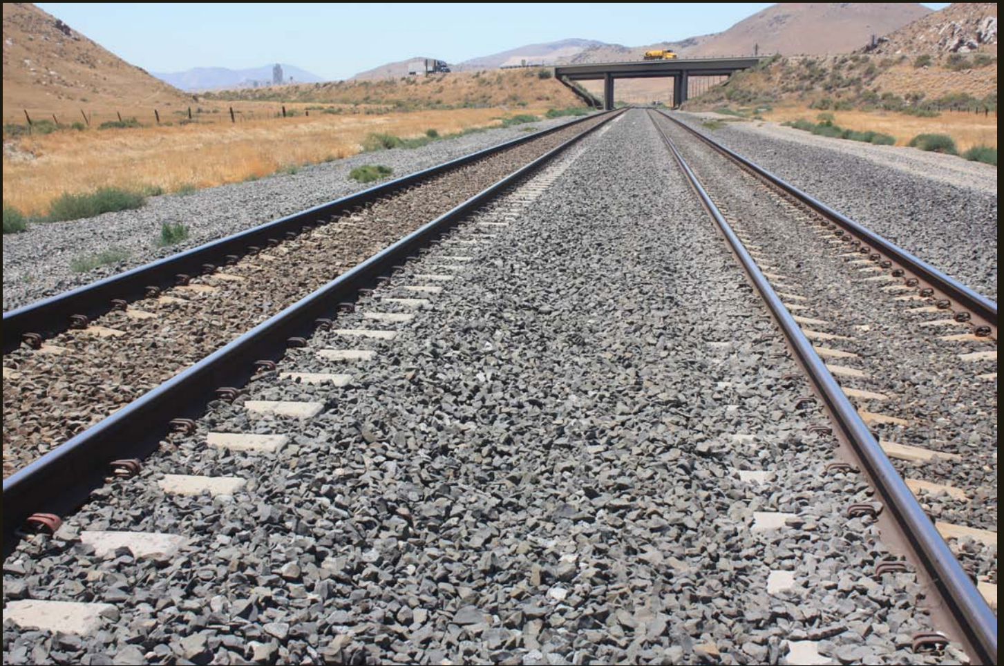
Eastward view of the SP (now UP) mainline, 3 miles east of the Tehachapi Depot. The overpass is at the point where the Tehachapi Valley lake bed is being captured by this dry creek, which the route follows eastward into the desert.
