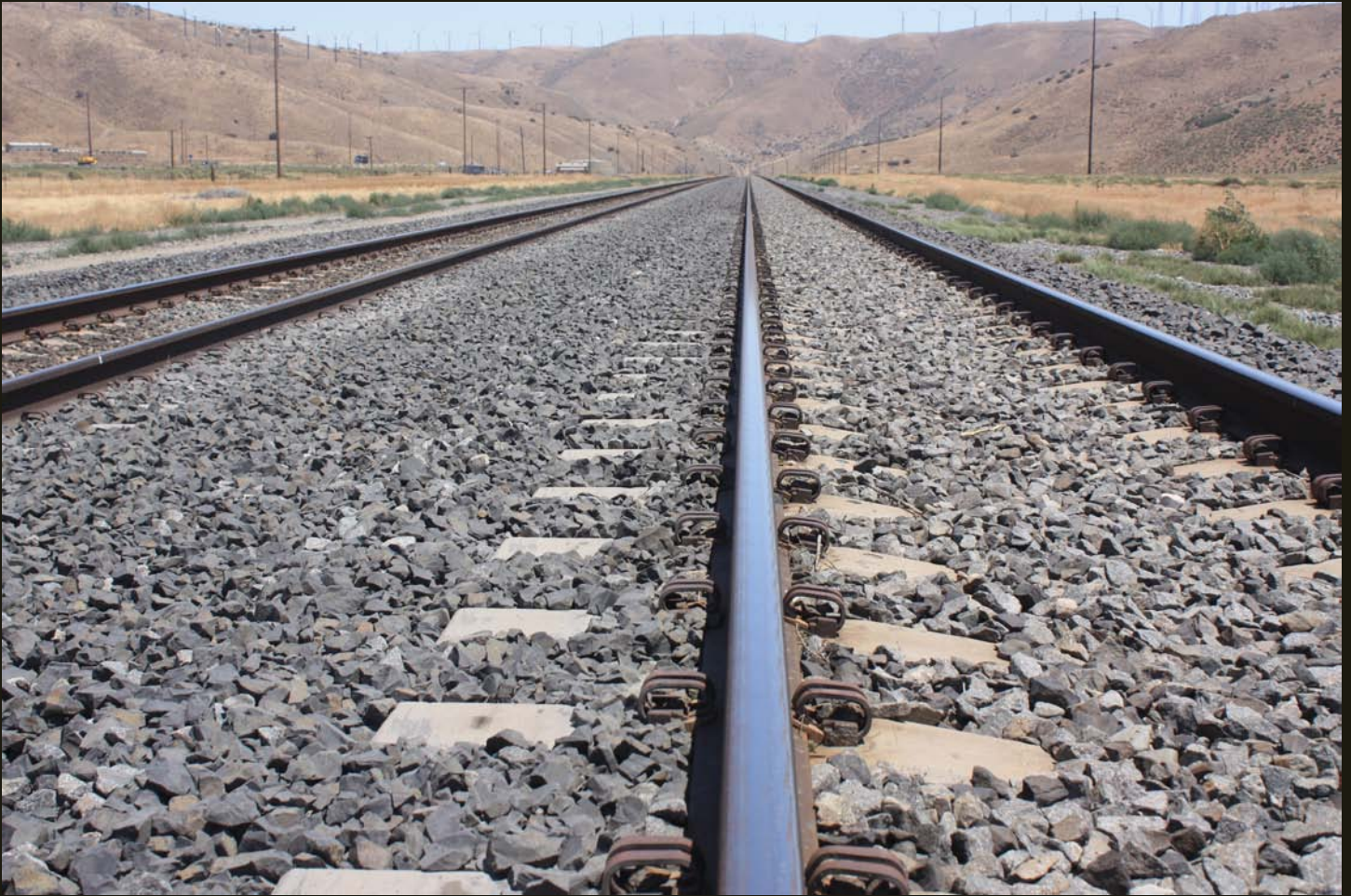
Westward view at same location as previous. Note the flat topography of the dry creek, much easier building than the west slope. A few miles farther east, the grassland gives way to Joshua Tree desert in the rain shadow of the Pacific Crest.
