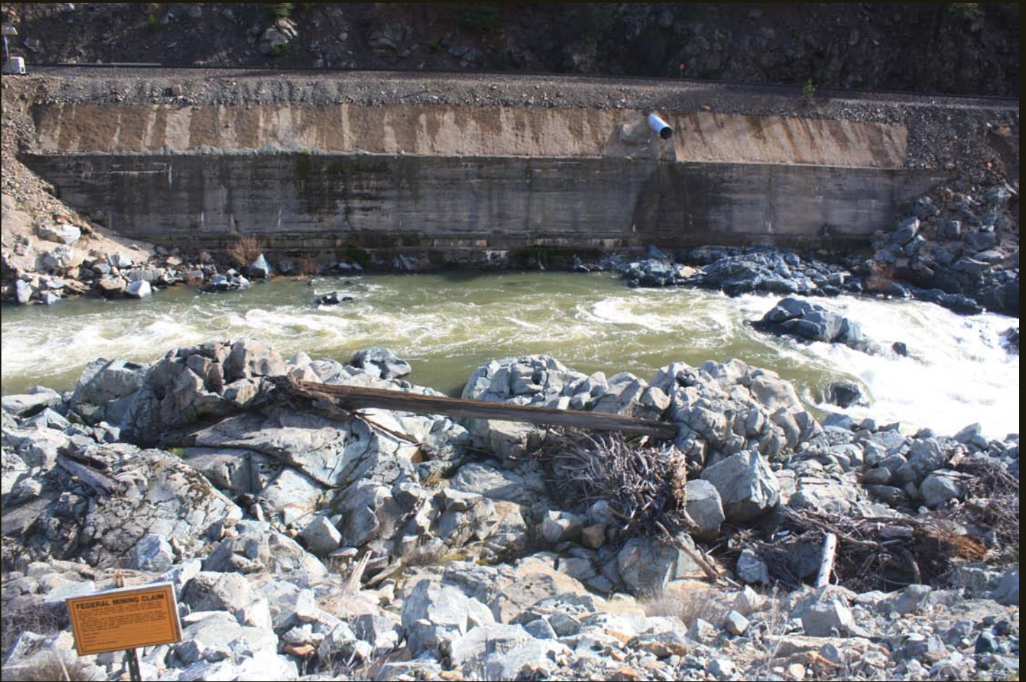
In narrow part of the canyon, the WP built a concrete retaining wall to carry the grade between the river and a vertical wall of rock.
