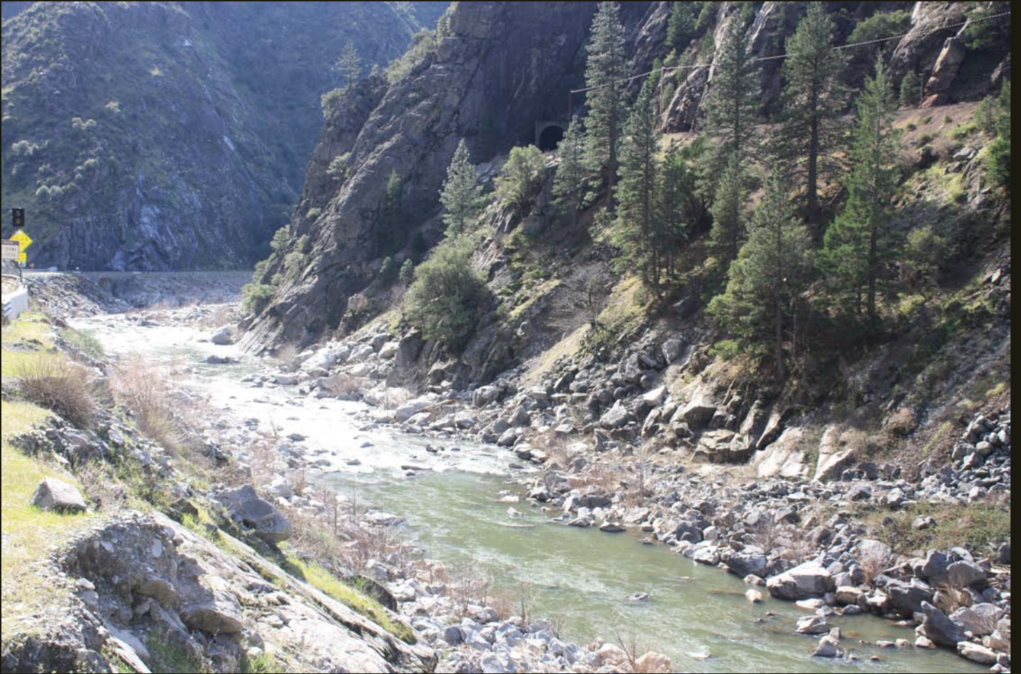
One of 34 tunnels on the Feather River Route. California Highway 70 on the left bank.
