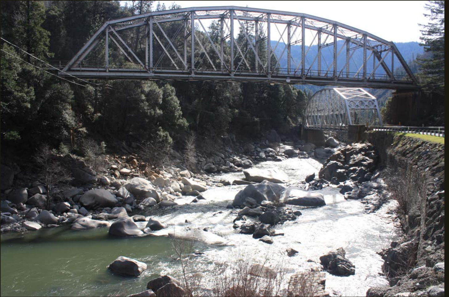
Dual steel truss bridges over the North Fork Feather River near Storrie, with the WP in foreground and California Highway 70 on the right.
