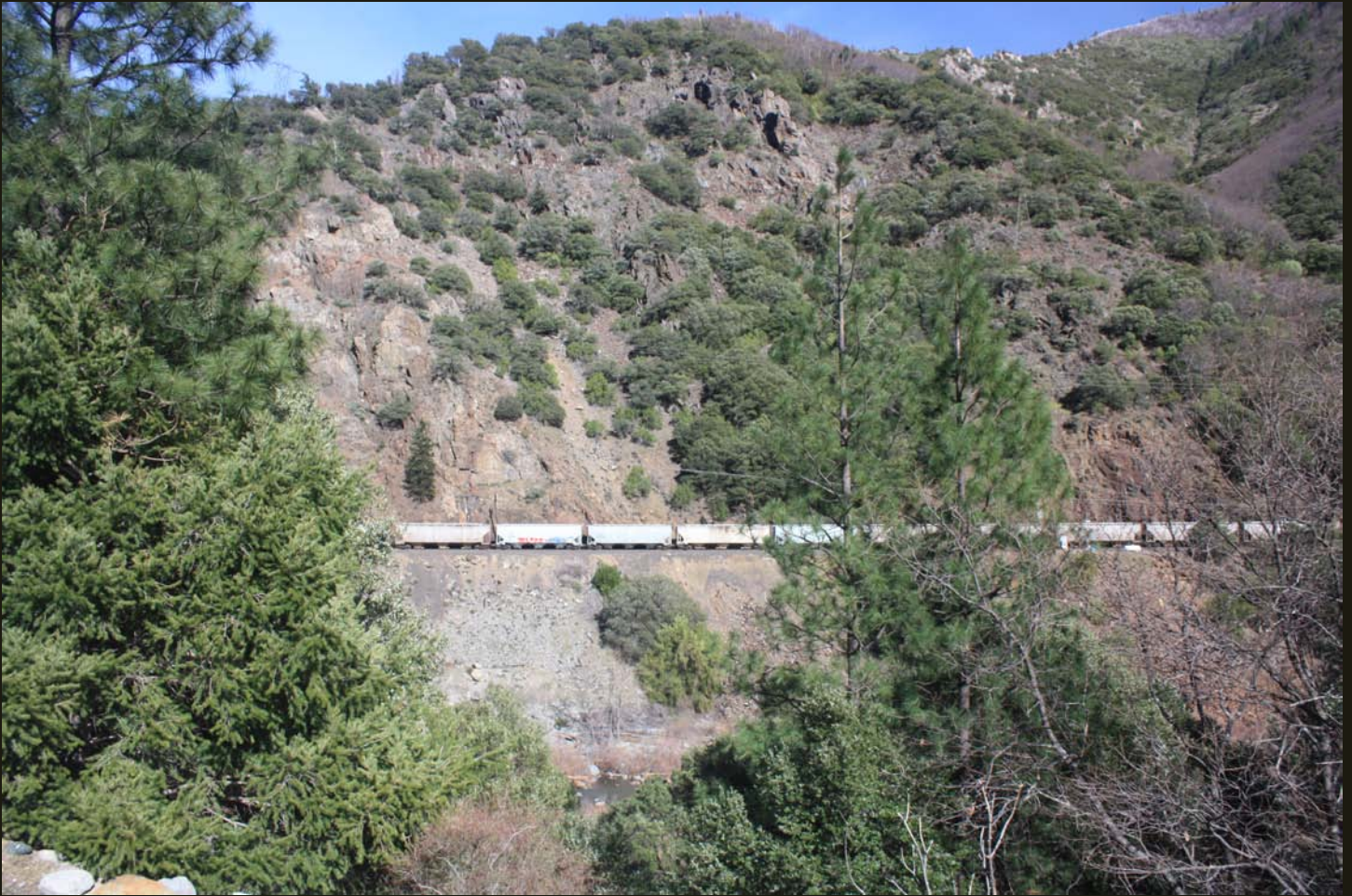
WP climbs the canyon wall to maintain the grade.
