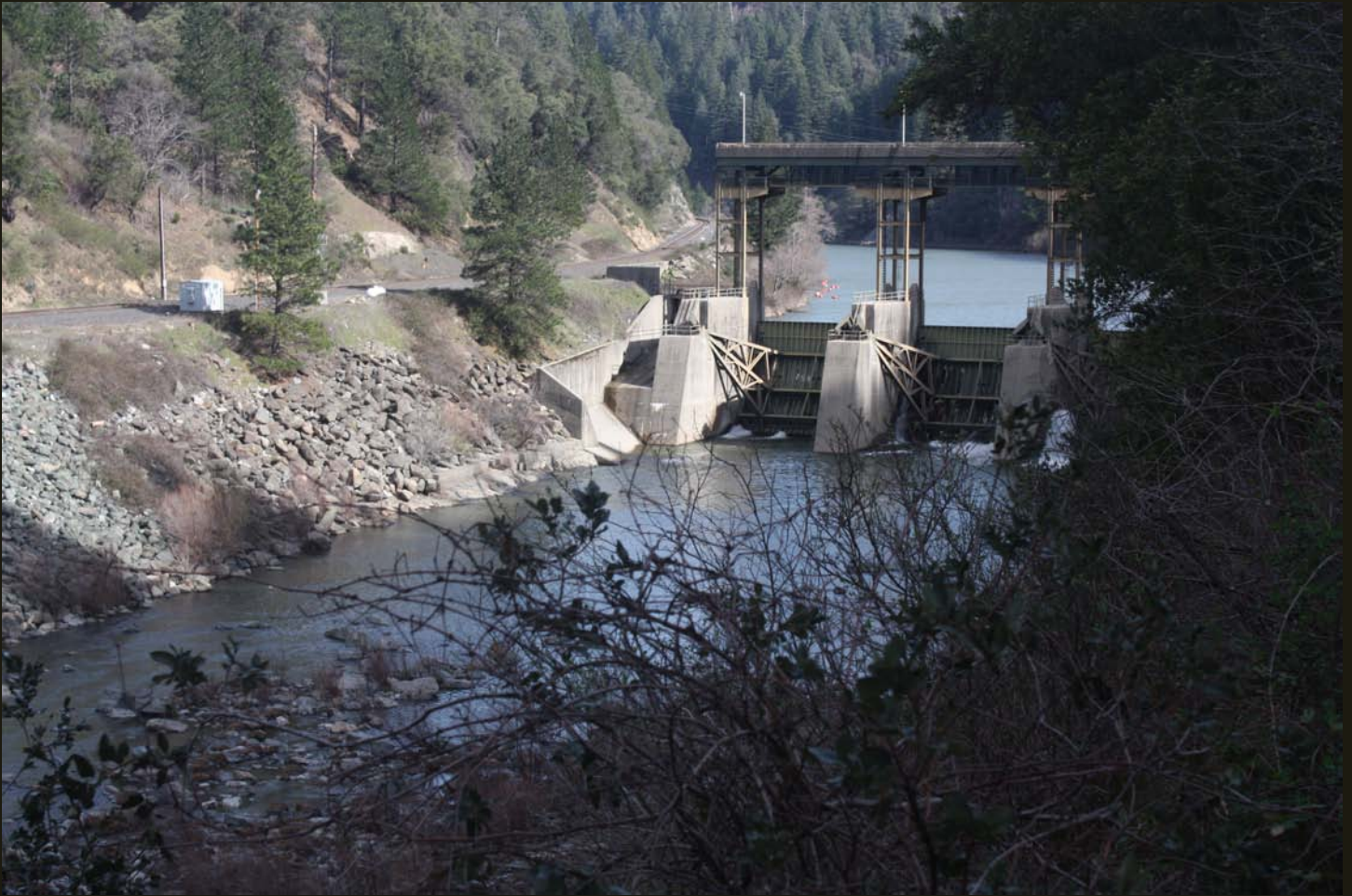
There are several small diversions of the North Fork Feather River for hydroelectric generation; the WP grade on the left (northwest) bank.
