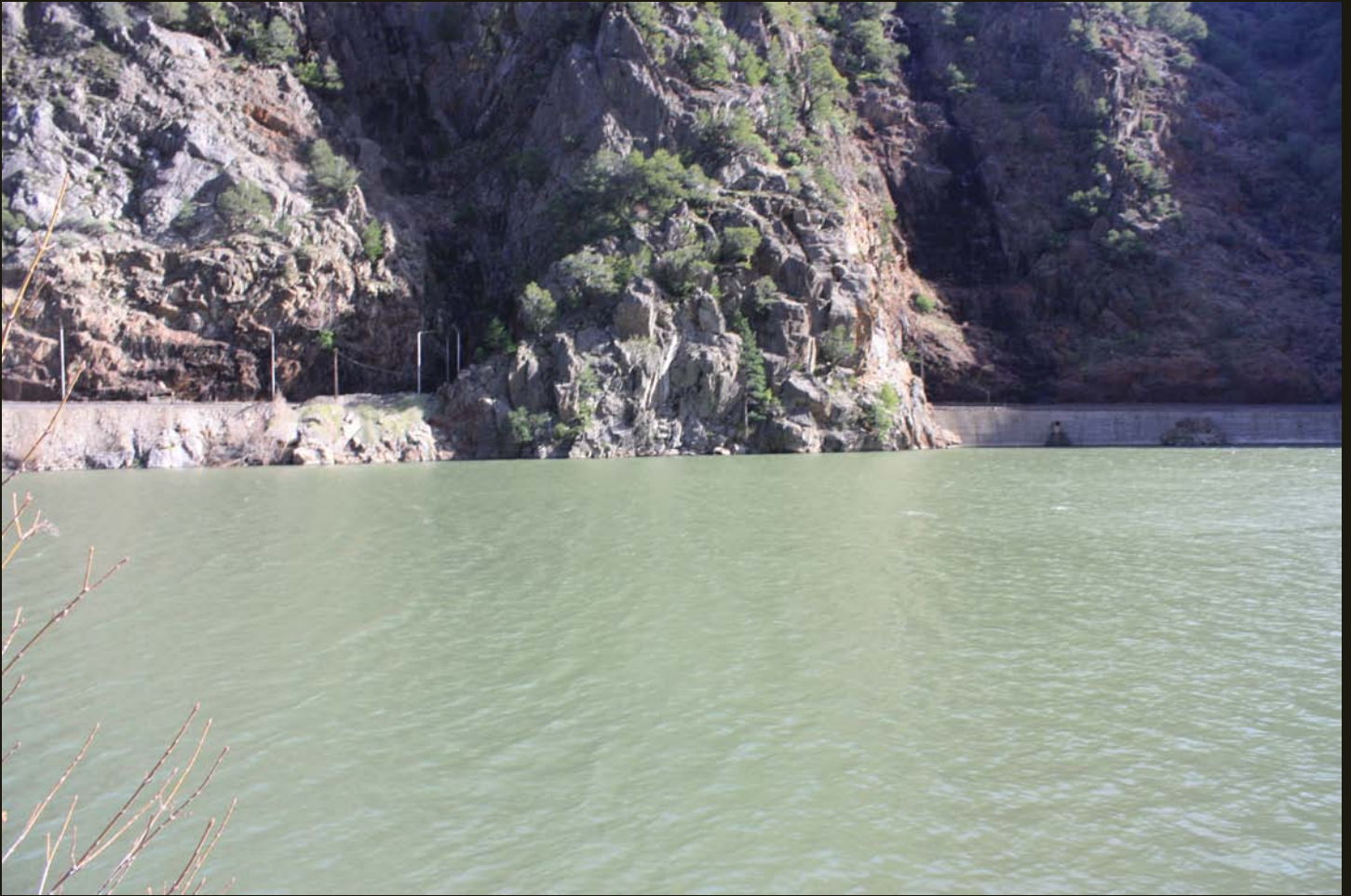
Small tunnel where the WP grade is just a few feet above the water level of Rock Creek Reservoir, where the North Fork Feather River is diverted for hydroelectric generation.
