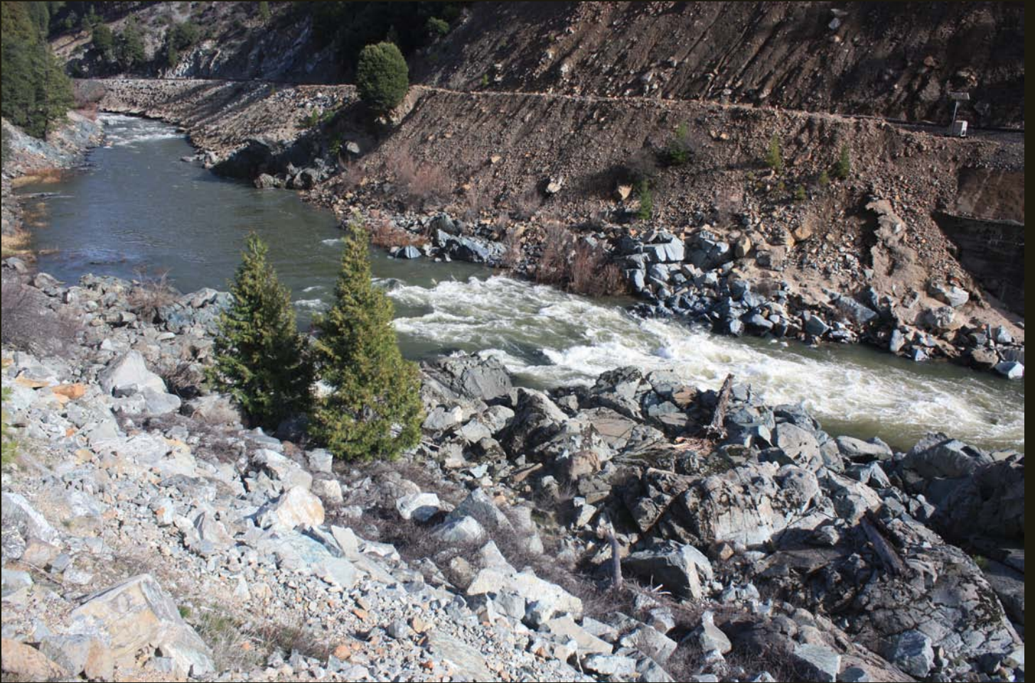
Cut and fill grade across a landslide.
