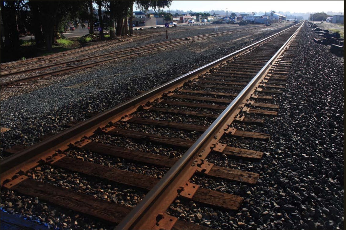
Southward view at the same location as previous. The SP (1901) mainline is on the right, several sidings are on the left. I believe the depot was once in the flat area to the left (east) of the sidings, just beyond the eucalyptus trees.
