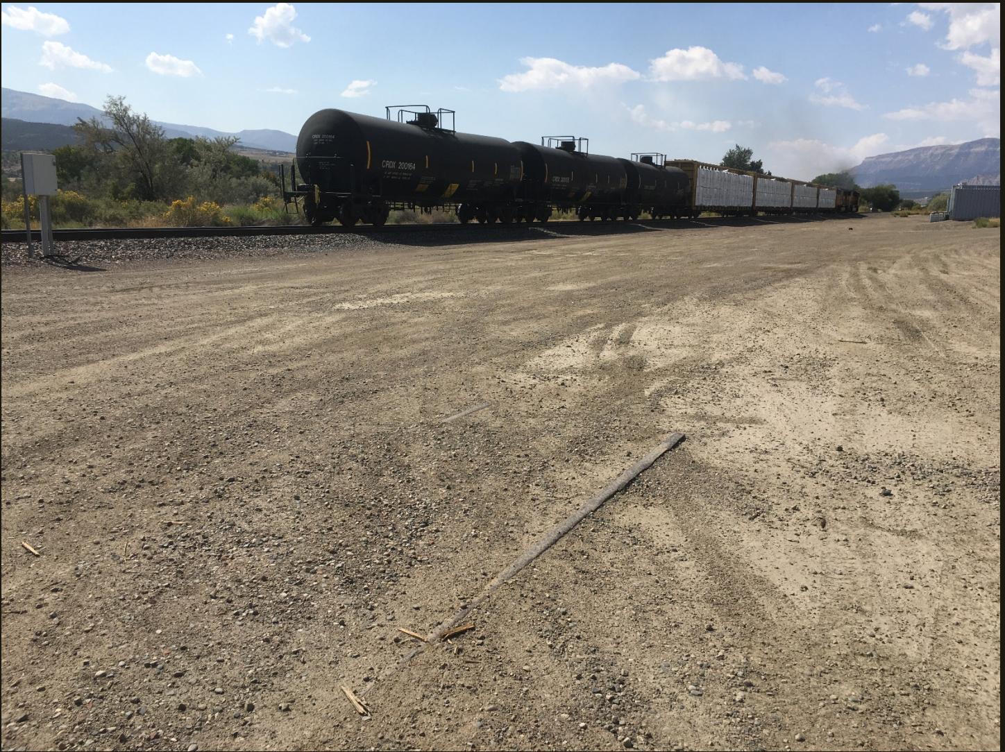
Southwestward view of some old rails (foreground) and a train coming through on the Rio Grande Joint Railway (1890), which is now on the Union Pacific's mainline through the Rockies via the Moffat Tunnel and D&RGW Dotsero Cutoff (1934). A 1952 topo map shows a siding at this location but all evidence of its connection to the mainline has since been obliterated.
