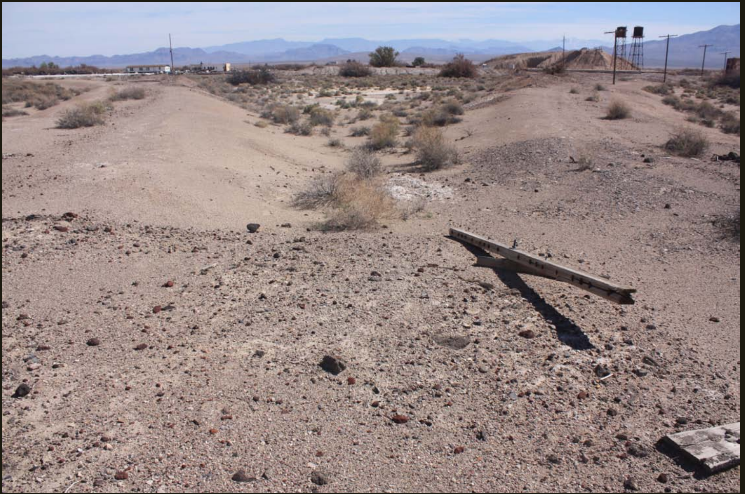
Eastward view of the western switch of the wye. Note the same loading ramp, water towers, and loading platform as before, visible in the right distance. A dual gauge switch, which is a very complex thing indeed, was once present in the immediate foreground.
