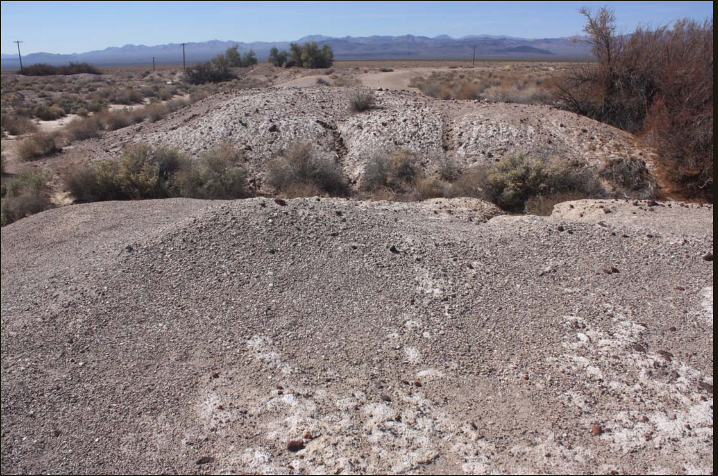
Southwestward view of the north arm of the wye, same location as previous. Note the breach in the fill grade in the foreground and the curvature to the right (west).
