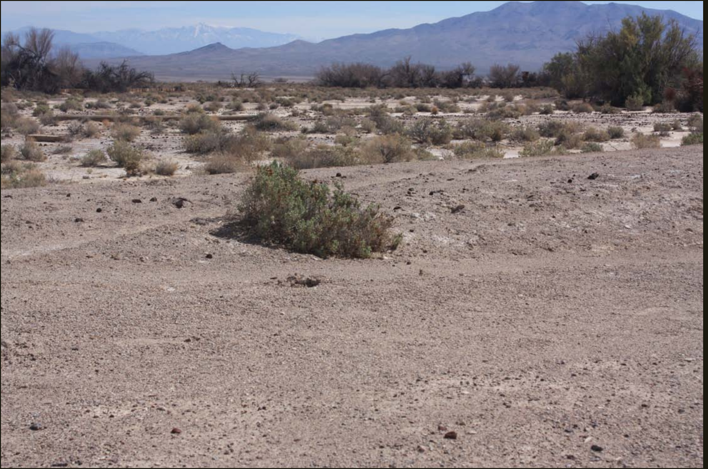
Eastward view of the T&T (1907) mainline at the switch for the narrow gauge siding. The straight T&T main line was built to standard gauge in 1907 and converted to dual gauge when the narrow gauge DV was completed in 1914. The nearly 12,000-foot Spring Mountains are visible in the distance, beyond which lies Las Vegas, Nevada.
