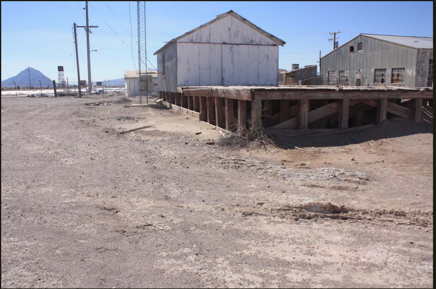
Southward view of a trackside loading facility just north of the wye and just west of the "D.V.R.R. TRACK SCALE" on the above map. Note the same water towers as before in the left distance.
