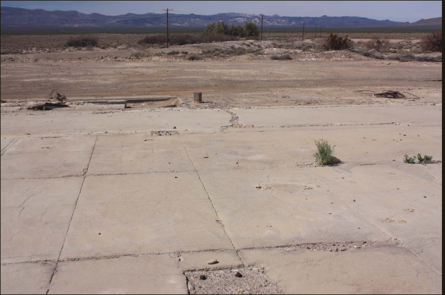
Westward view of the T&T (1907) from the same location as previous on the loading dock for the Pacific Coast Borax Company Crushing and Concentrating Plant. The two branches for the yew for the Ryan Branch are visible in the middle ground. The flat area between the loading dock and the yew once contained several sidings of standard, narrow, and dual gauge (see above map).
