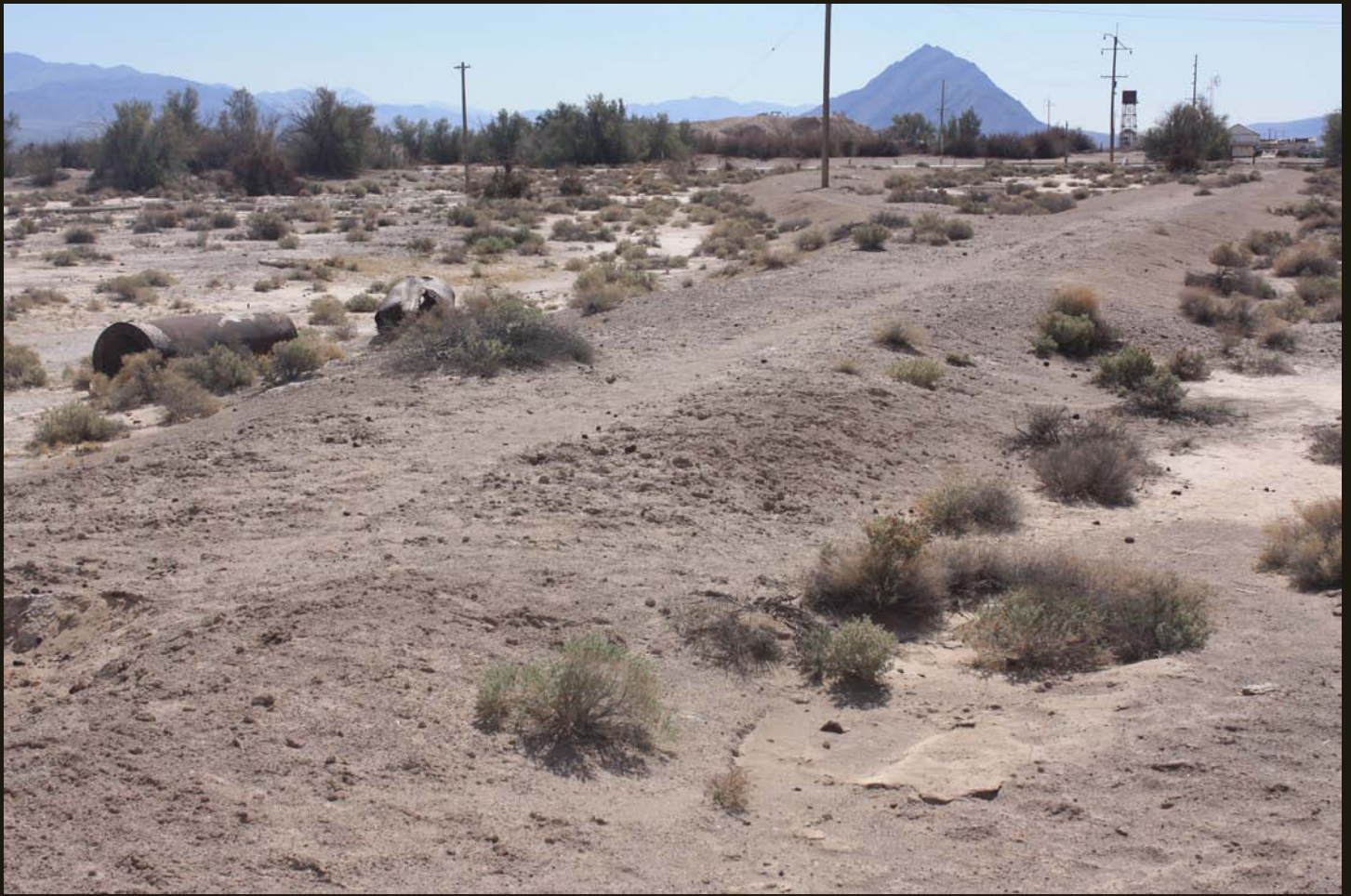
Southward view of the T&T (1907) mainline at the north end of Death Valley Junction, 200 feet north of previous location. Note the same water towers as before. The narrow gauge siding with the "D.V.R.R. TRACK SCALE" is clearly visible (nearest power pole is set into the narrow gauge fill grade). The straight T&T main line was built to standard gauge in 1907 and converted to dual gauge when the narrow gauge DV was completed in 1914.
