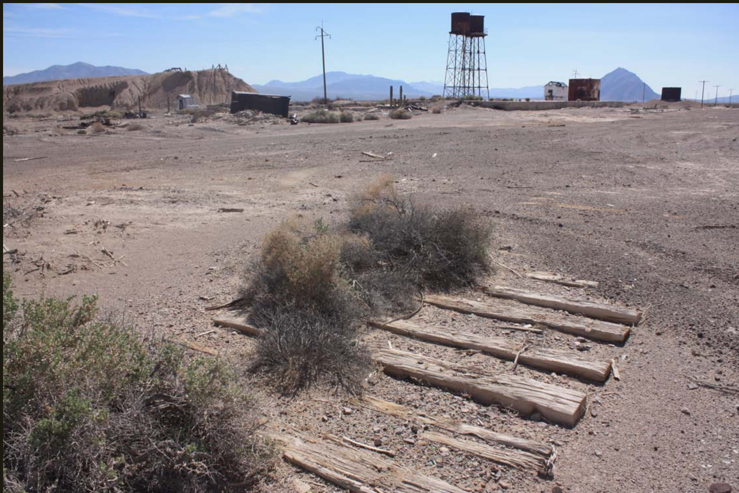
Southeastward view of the T&T (1907), with some ties still in place in the foreground. These ties are on the standard gauge siding between a narrow gauge DV siding the T&T the mainline, which according to the map was dual gauge within the map area. Note (from left to right) the same dirt-fill loading ramp, two water towers, loading platform, and two tanks as before.
