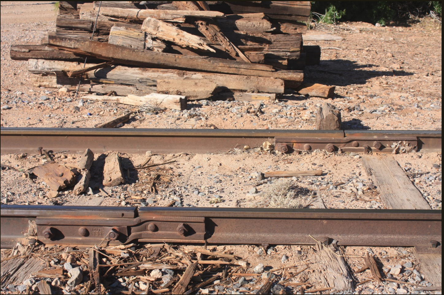
Southwestward view of the SPLA&SL St. Thomas Branch (1912), same location as previous. Note that the bracket connecting the rails is bent to accommodate rails of two different weights, the rail to the right being the lighter of the two rails.
