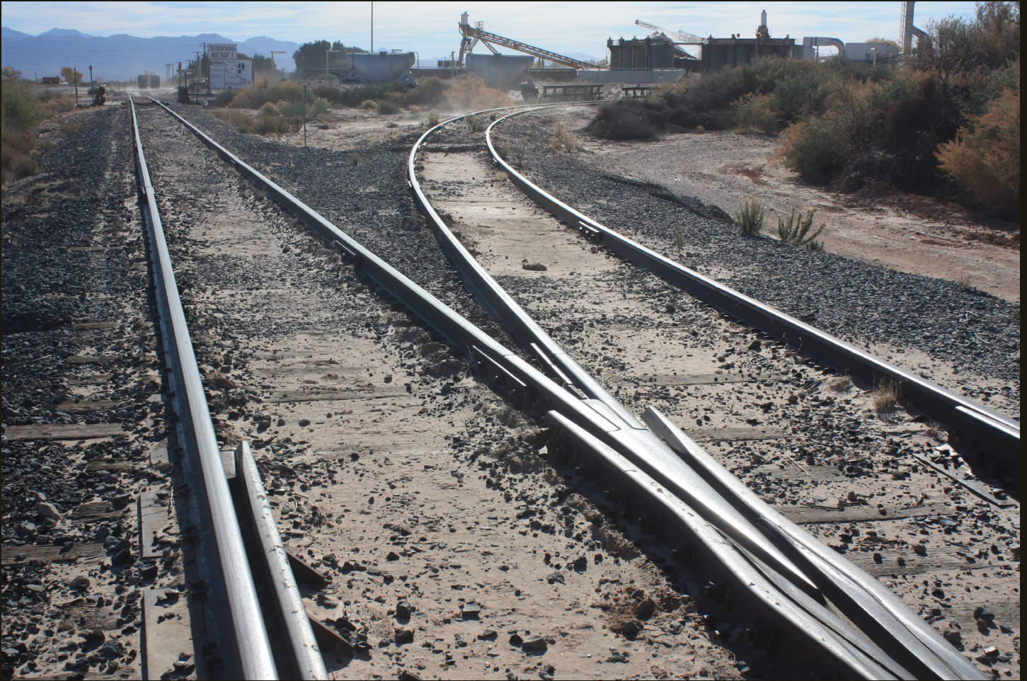
Southward view of the SPLA&SL St. Thomas Branch (1912), about a mile southeast of previous location. The track curving to the right is the north branch of a wye serving the Simplot Silica Products Inc. mine and silica plant which, according to its web site, has produced "high-quality silica sand...since 1927 and has the proven reserves to continue supplying you well into the future." Note the rail cars in the left distance; the south branch of the wye comes in just in front of those cars and the track ends just beyond them.
