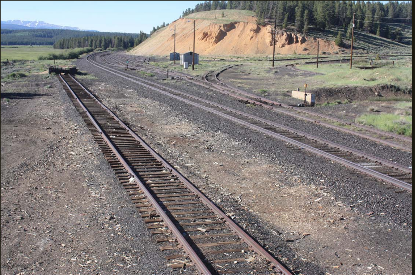
The D&RG reached Leadville in 1880. In this northward view 4 miles west of Leadville, the track in the right foreground and the branch to the right (east) together follow the general alignment of the 1880 D&RG narrow gauge Leadville Branch. The current mainline that disappears around the bend is the D&RG route that was completed over Tennessee Pass to Aspen in 1887. The floodplain of the Arkansas River is the green area in the left distance.
