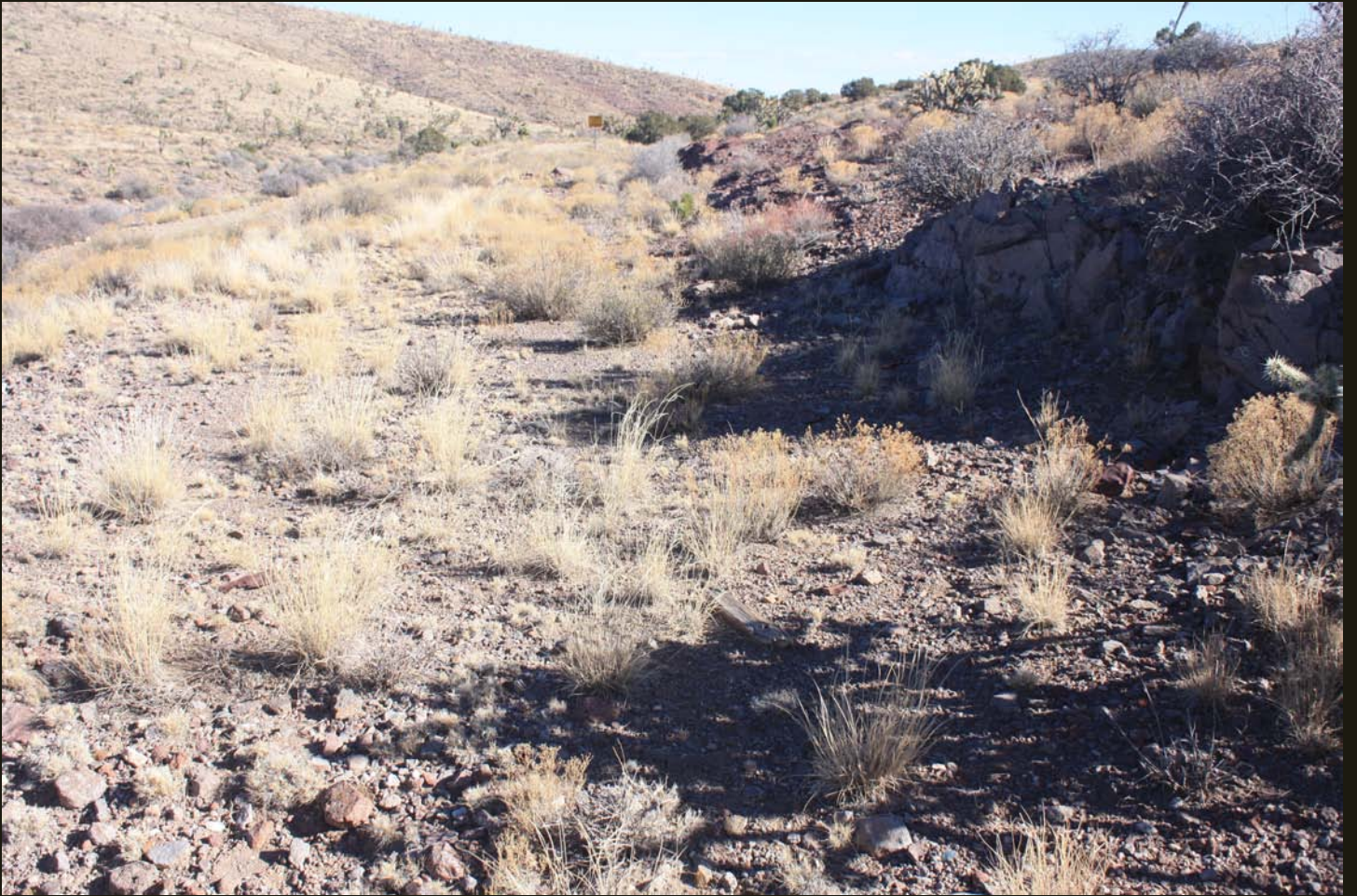
Eastward view of the cut grade of the B&S (1907) at Barnwell.
