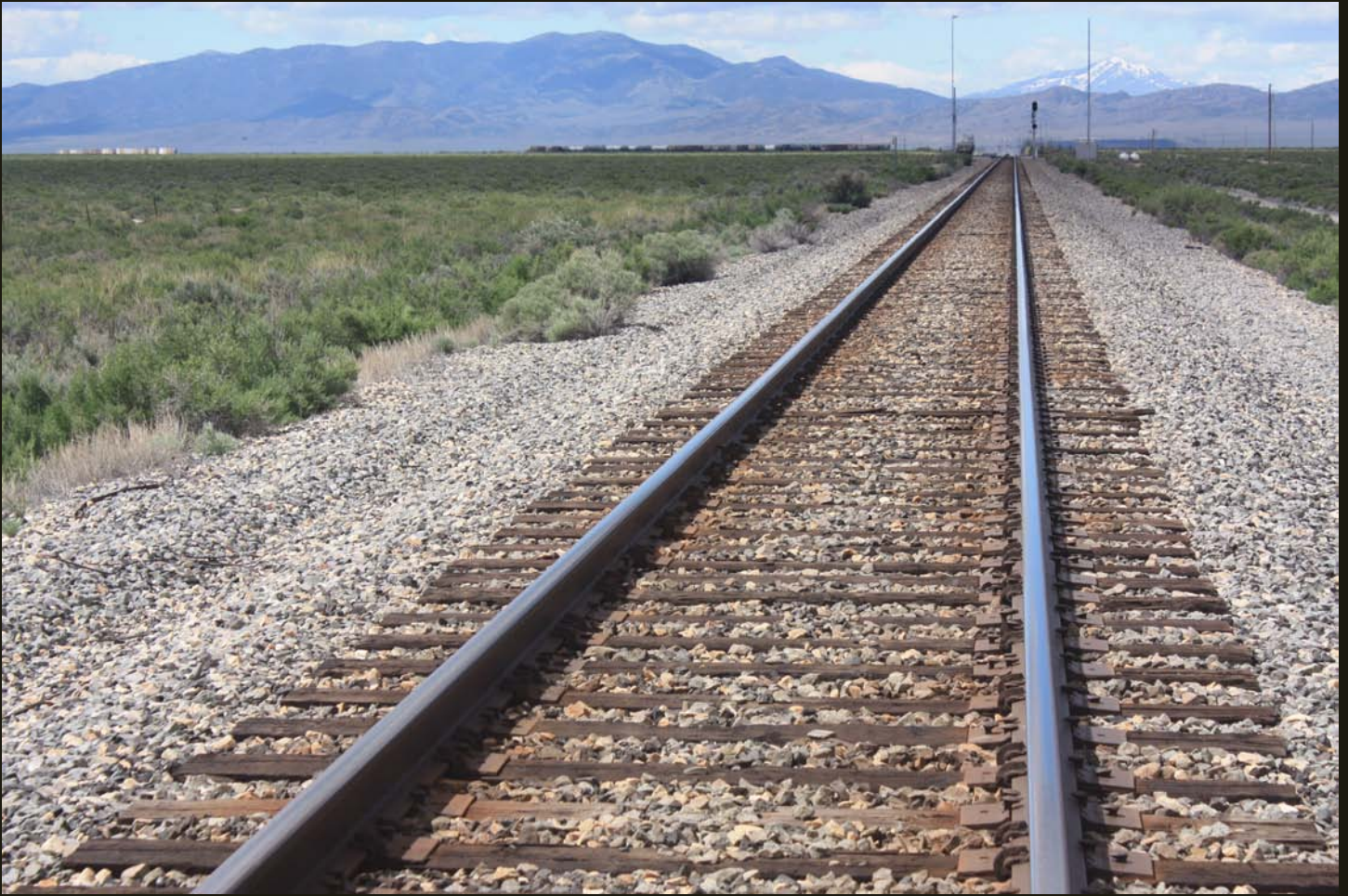
Southwestward view of the WP (1909), 2 miles northeast of Shafter, where the WP crosses the NN (1906). Note the two separate groups of cars stored on the NN south of Shafter (to the left of the WP alignment).
