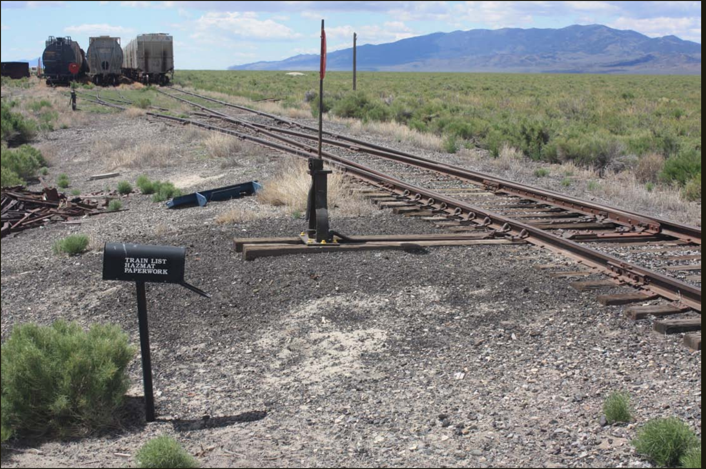
Southward view of the NN (1906), same switch as in the previous photo.
