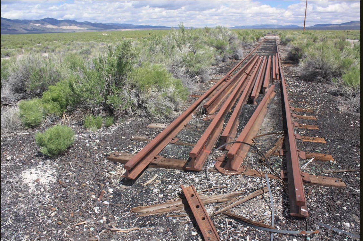
Northward view of the NN (1906) 120 feet north of the WP (1909). The removed rails are piled on the tracks.
