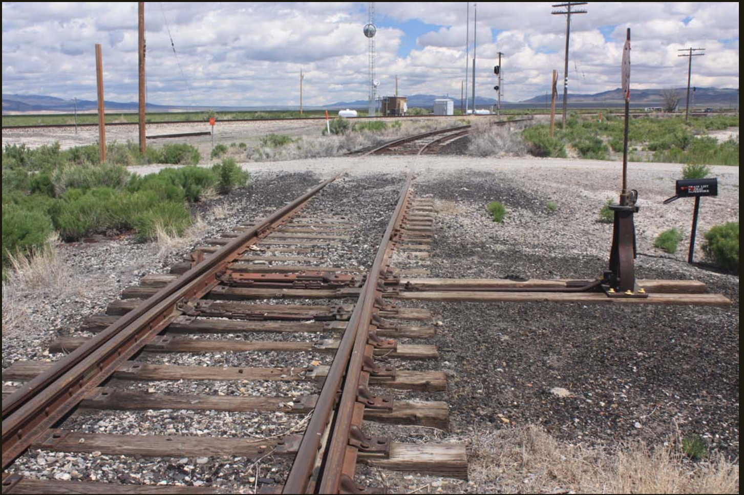
Northward view of the NN (1906) at Shafter. The switch in the foreground, which leads to the stored cars behind the viewer, is on the original NN grade, but beyond the switch the curved track is later (1996?) connecting track. The original NN went straight between the two buildings.
