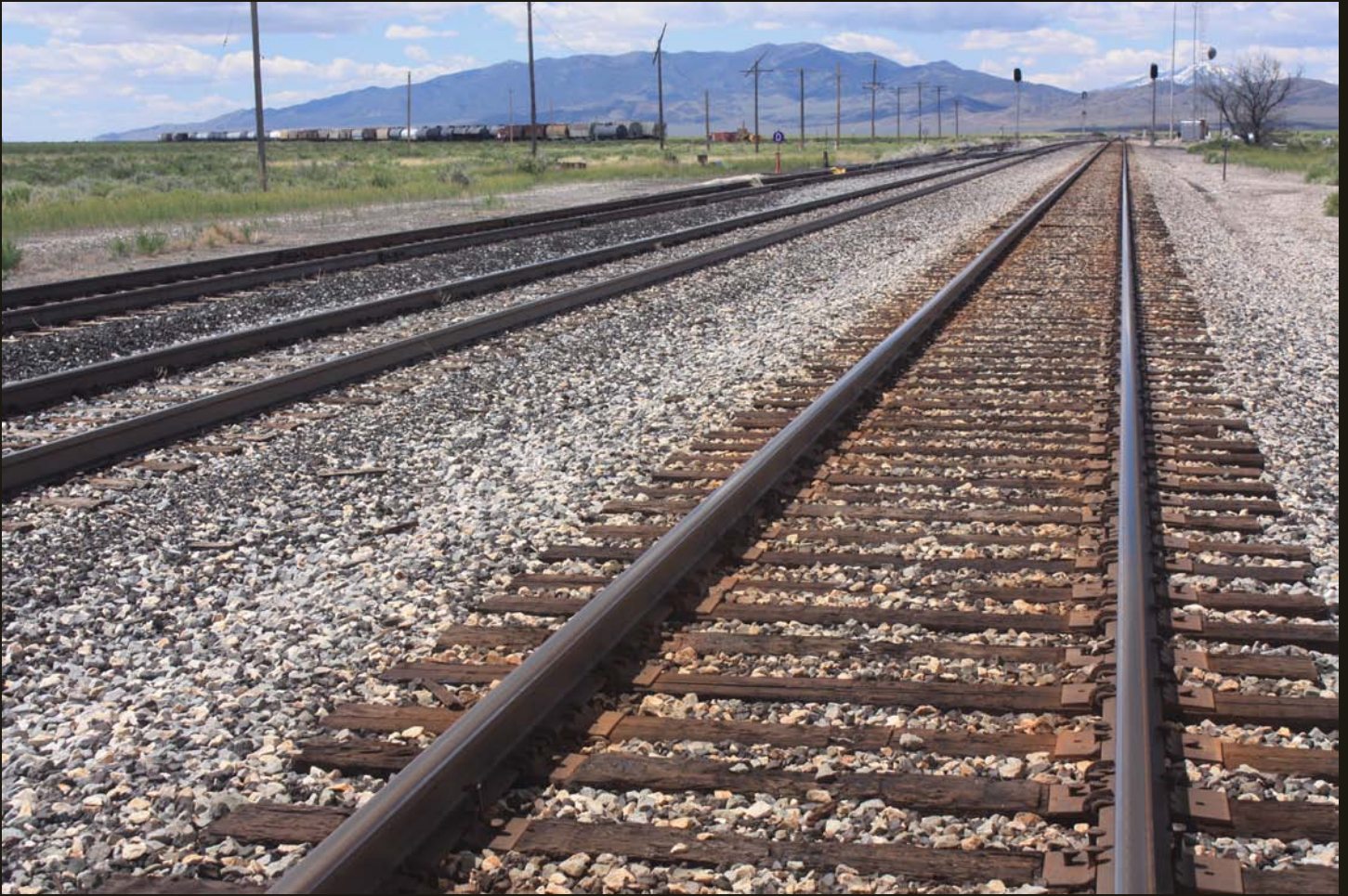
Southwestward view of the WP (1909), 1,000 feet northeast of the WP-NN grade crossing at Shafter. The original grade crossing has been removed and the NN (1906) north of the crossing is disconnected. The siding to the far left connects the WP to the NN south of the crossing and may have been built in 1996 for the BHP Nevada Railroad. Satellite imagery shows an abandoned WP turning wye to the left (southeast) of the viewer.
