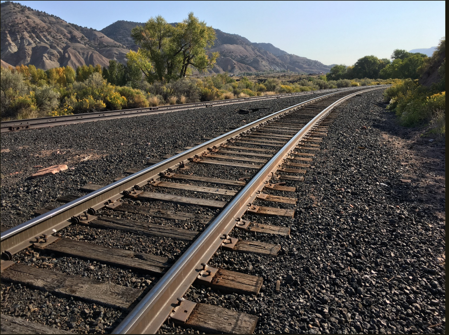
Eastward view 200 feet southeast of the previous location. The D&RG Aspen Branch (1887n) is in the foreground. The east branch of the wye is to its left (north) and runs parallel to the Aspen Branch, like a siding, for 1,700 feet before joining the mainline to Tennessee Pass.
