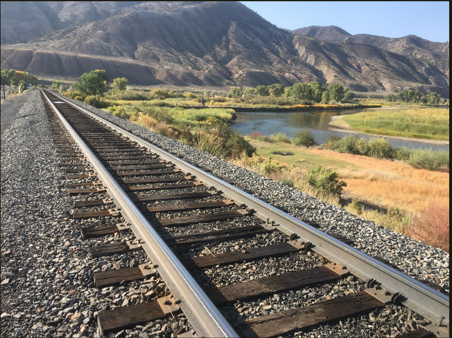
Southward view of the D&RGW Dotsero Cutoff (1934) at the same location as previous. The north tip of the wye that connects the Dotsero Cutoff to the D&RG Aspen Branch (1887n) is barely visible in the distance. The stream that enters the photo from the left is the Eagle River, which flows into the Colorado River just above the center of this photograph. The D&RG Aspen Branch (1887n) follows the Eagle River all the way from Tennessee Pass to this confluence with the Colorado River and follows the Colorado River from here westward through Glenwood Springs all the way to Grand Junction.
