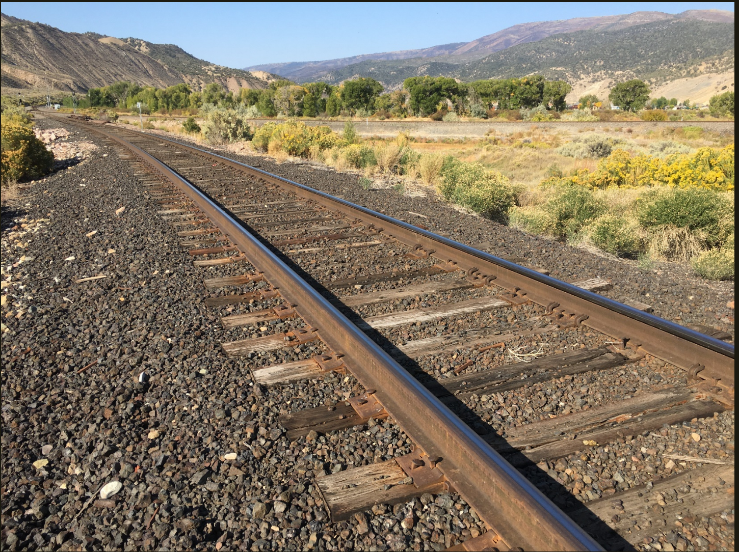
Westward view of the D&RG Aspen Branch (1887n) at the same location as previous. The west branch of the wye is visible across the photo in the distance and the two lines join in the left distance.
