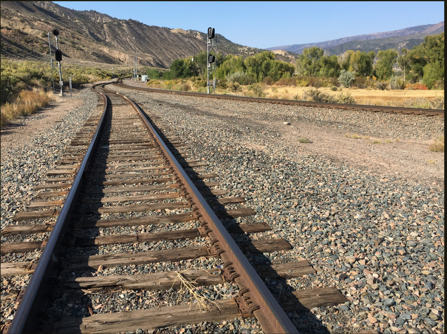
Southwestward view of the D&RG Aspen Branch (1887n) 500 feet southwest of the previous location. The west branch of the wye, which is the UP mainline, enters from the right and joins the Aspen Branch in the left distance, beyond which the mainline continues to Grand Junction and Utah.
