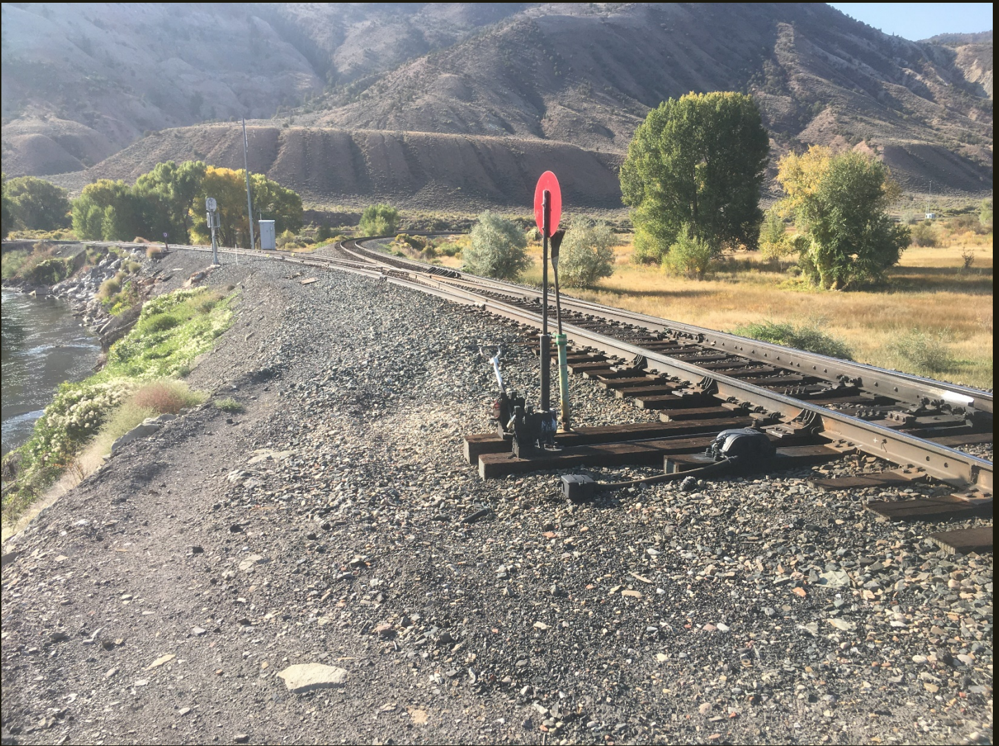
Southward view of the tip of the Dotsero wye a few steps south of the previous location. The Eagle River is on the far left and is diverted by the massive fill grade for the wye. The bolted rails on the east branch of the wye (on the left) connect to the part of the D&RG Aspen Branch (1887n) that goes to Tennessee Pass; that trackage has been inactive since the 1990's. The welded track on the west (right-hand) branch of the wye is today's UP mainline.
