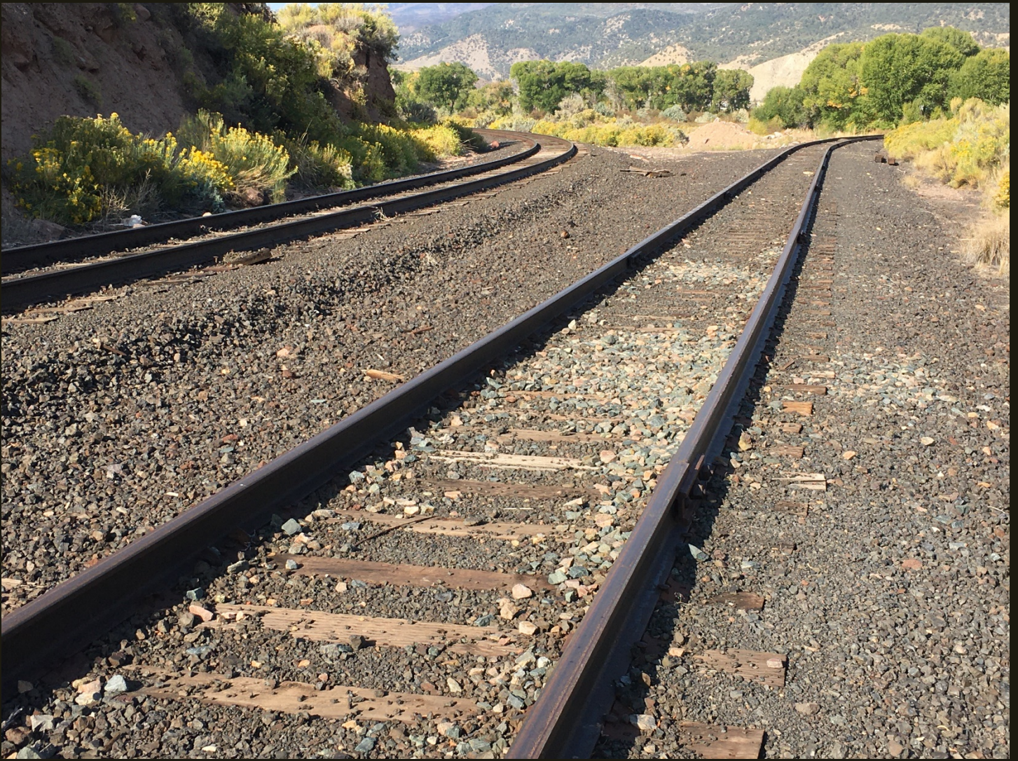
Westward view at the same location as previous. The east branch of the wye is in the foreground and the D&RG Aspen Branch (1887n) is to its left (south).
