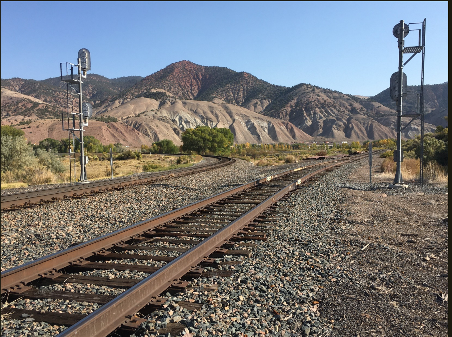
Northeastward view of the D&RG Aspen Branch (1887n) 150 feet southwest of the previous location. The west branch of the wye -- the mainline to the Moffat Tunnel since 1934 -- is to the left.
