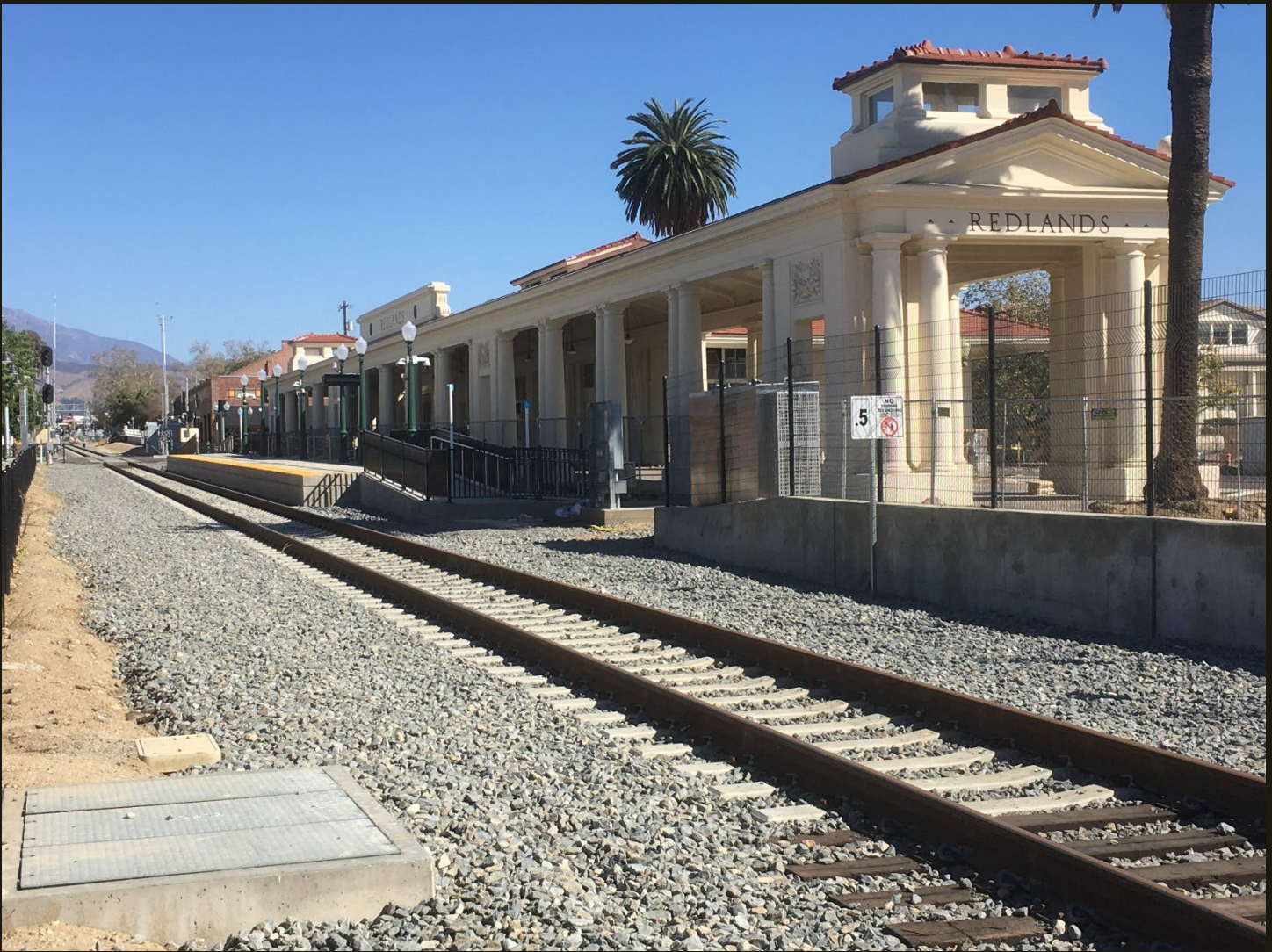
Eastward view of the CS Redlands Loop (1888) and the Redlands Santa Fe Depot, as seen in October 2021, several years after the other photos. Note the upgraded track and ballast for new commuter trains that run on the CS Redlands Loop (1888) between here and the San Bernardino Santa Fe Depot.
