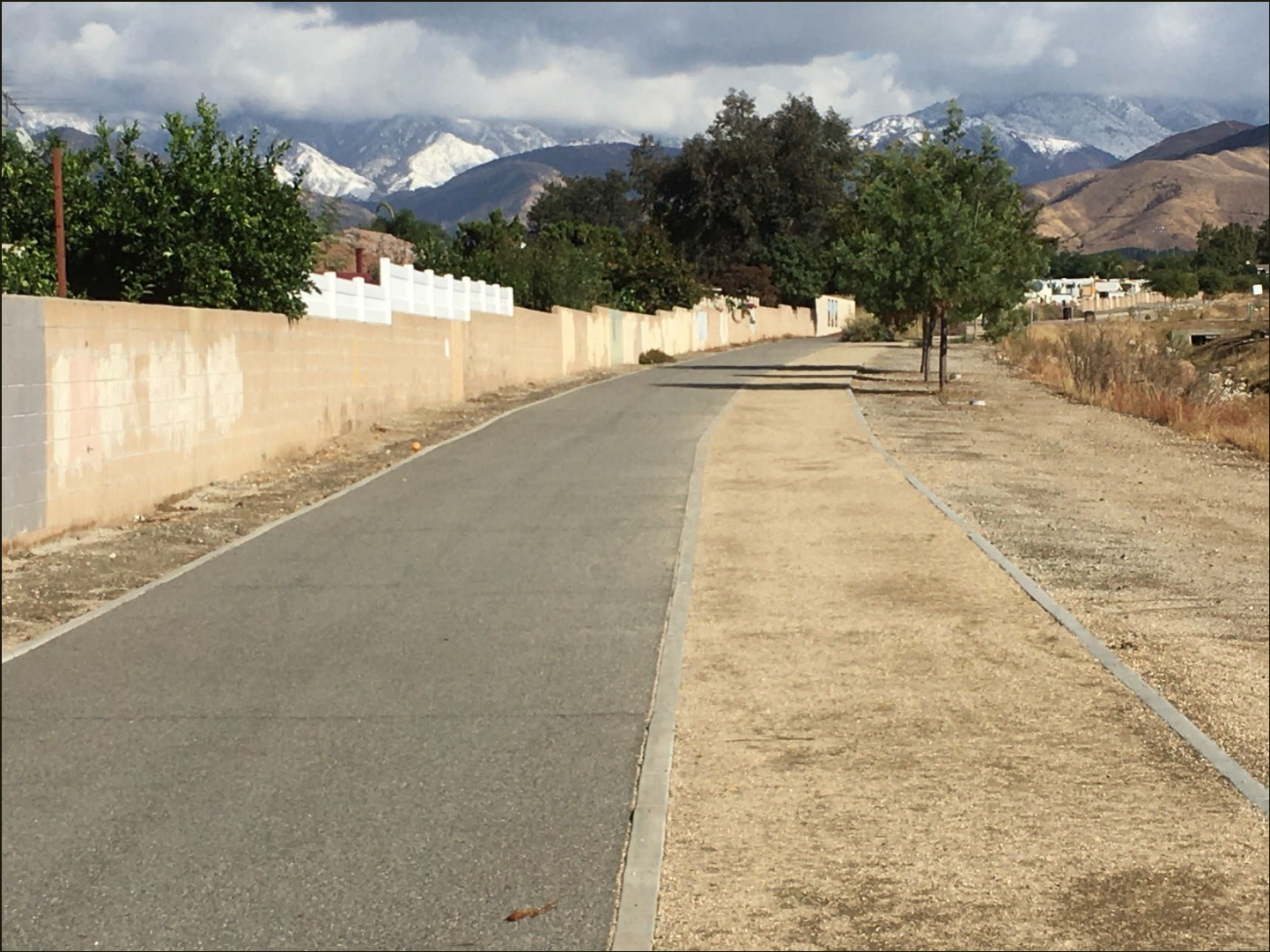
Northeastward view of the CS Redlands Loop (1888)/Orange Blossom Trail 400 feet northeast of the previous location.
