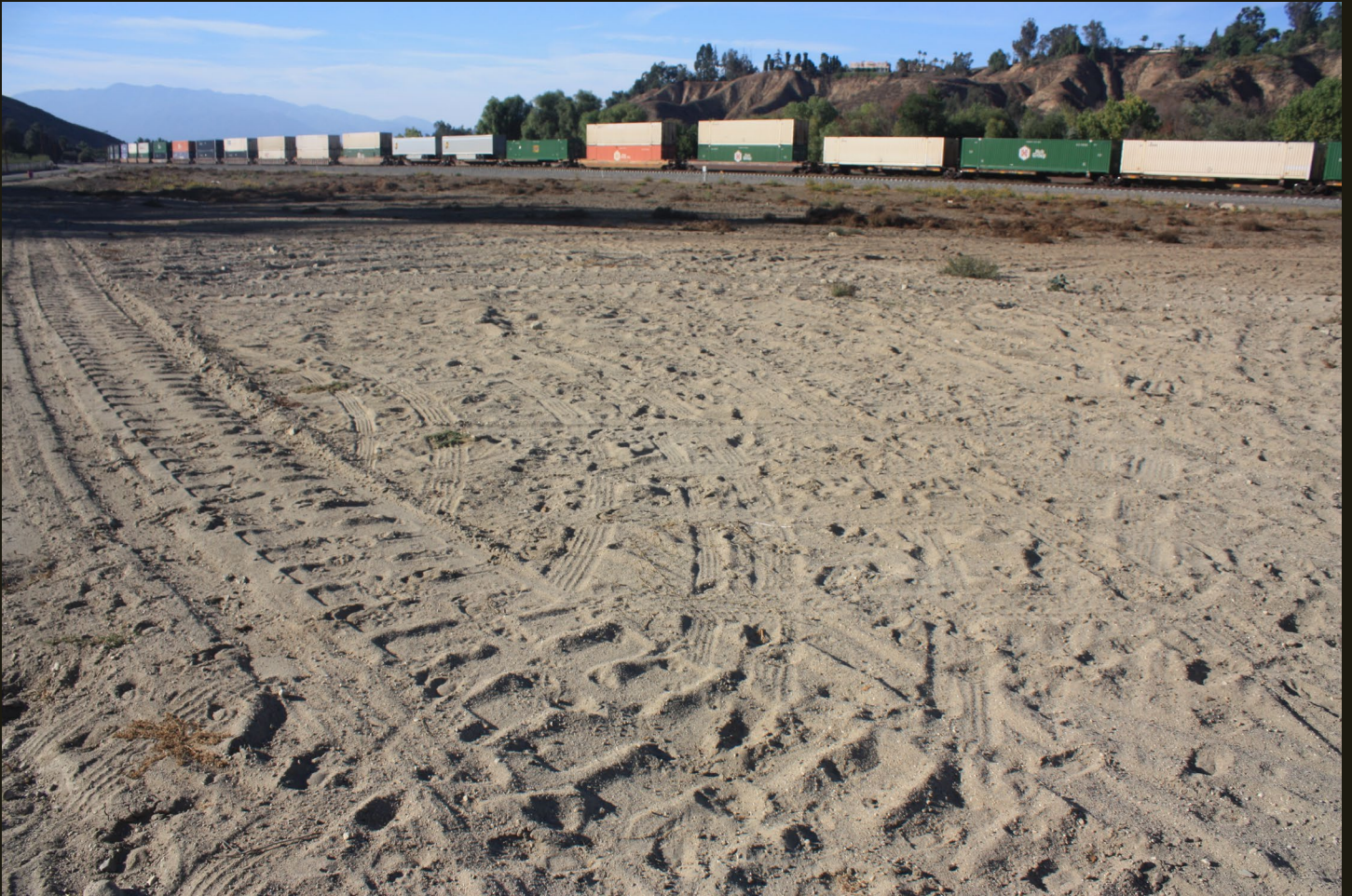
Northwestward view of the SP Sunset Route (1881) 7 miles northwest of the previous location, at the western entrance to San Timoteo Canyon, where the canyon opens up onto the fertile plains around Redlands. The houses on the bluff are the southern edge of Redlands and 10,000-foot Mount San Antonio ("Old Baldy") looms in the distance as yet another UP container train hauls empties back to LA.
