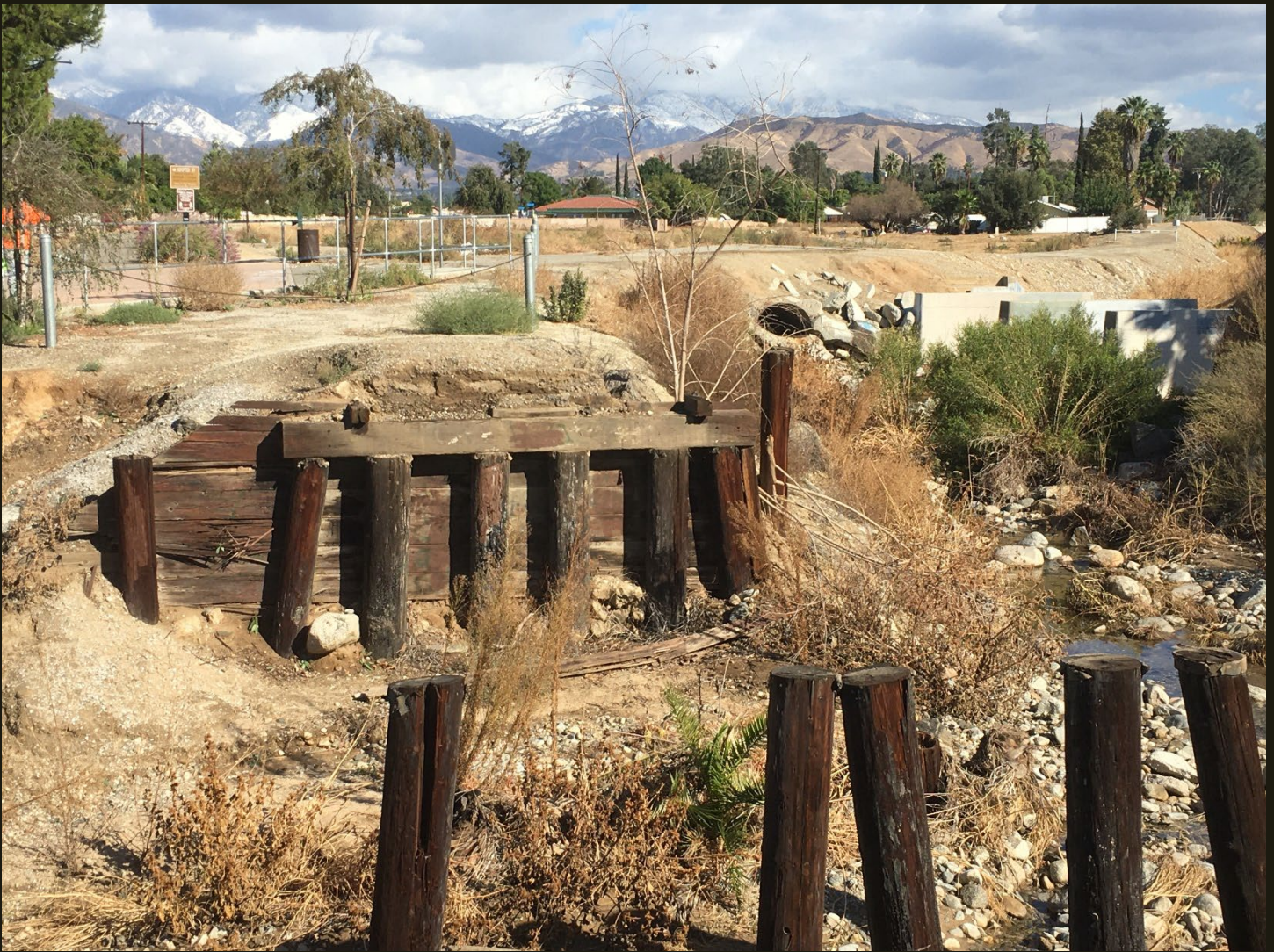
Northeastward view of the CS Redlands Loop (1888)/Orange Blossom Trail 2,000 feet east of the previous location. The trail goes around this wood-pile bridge over a small drainage and rejoins the original alignment in the right distance. I'm not sure if the concrete supports on the right were part of the railroad.
