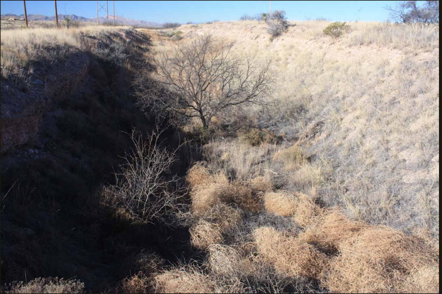
Westward view of the EP&SW (1912) cut grade, filled with tumbleweed, same location as previous. The parallel SP/UP double track is off to the left (near power poles).
