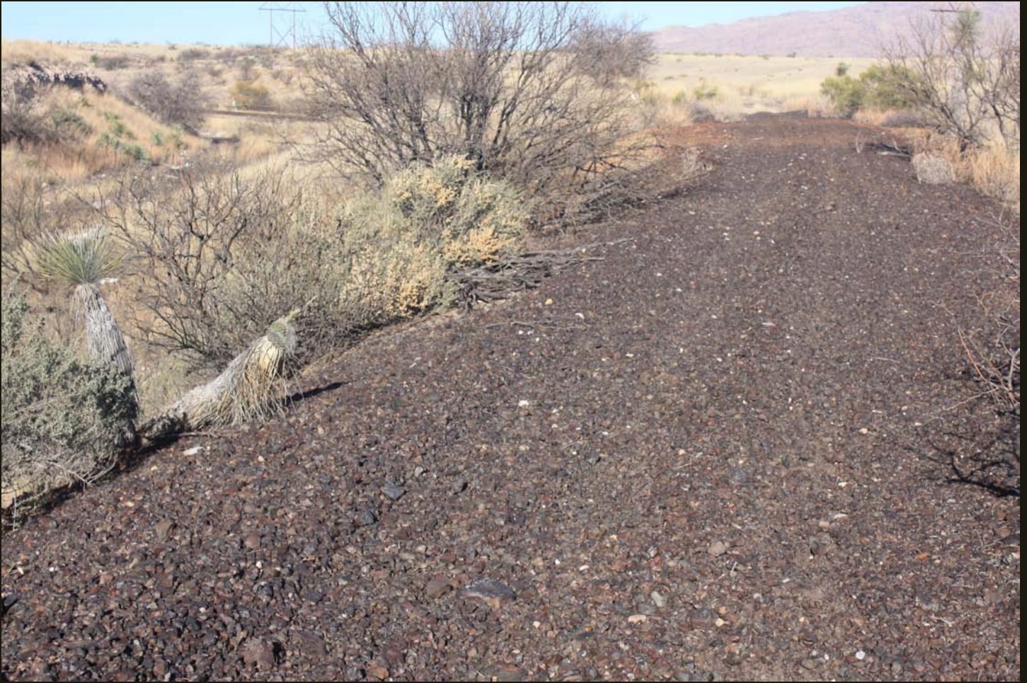
Northwestward view of the end of the EP&SW (1912) fill grade for the Mescal overpass (foreground) and the SP's 1920's re-alignment to the left and lower down (same level as the SP tracks, visible in upper left). From the 1920's until 1960's, that lower grade is where the SP's South Line split from the North Line to rejoin in El Paso.
