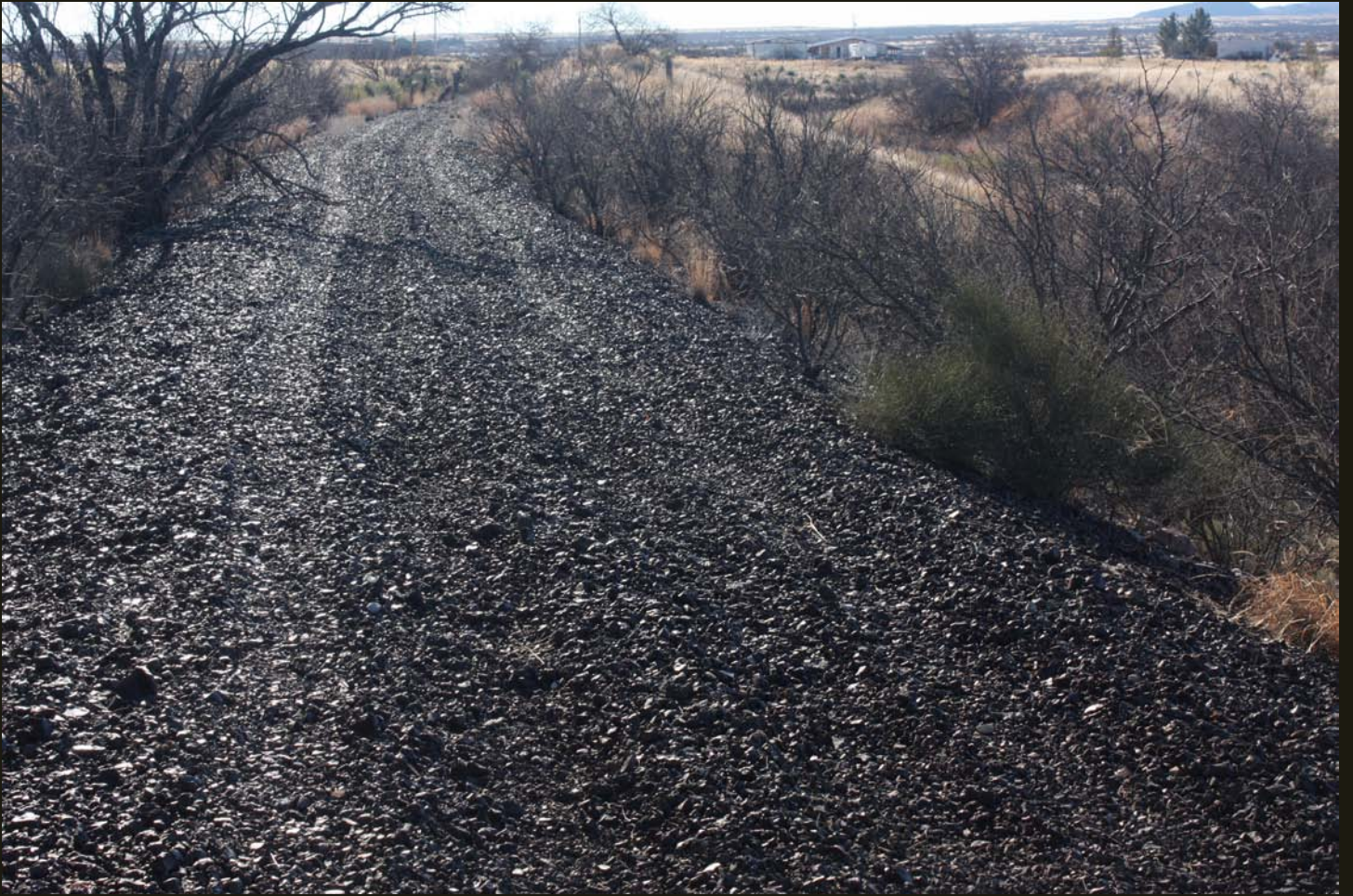
Southeastward view of the EP&SW (1912) fill grade for the Mescal overpass (foreground) and the SP's 1920's re-alignment to the right and lower down (in the cut grade on this side of the house).
