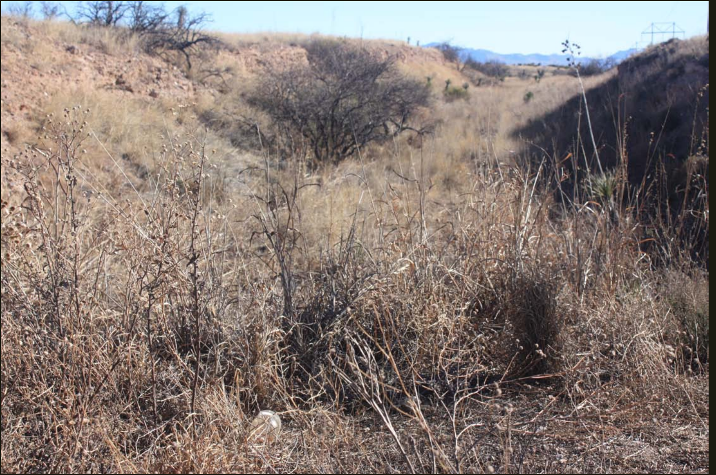
Eastward view of the EP&SW (1912) cut grade, a quarter mile west of Mescal. The SP/UP double track is off to the right (south).
